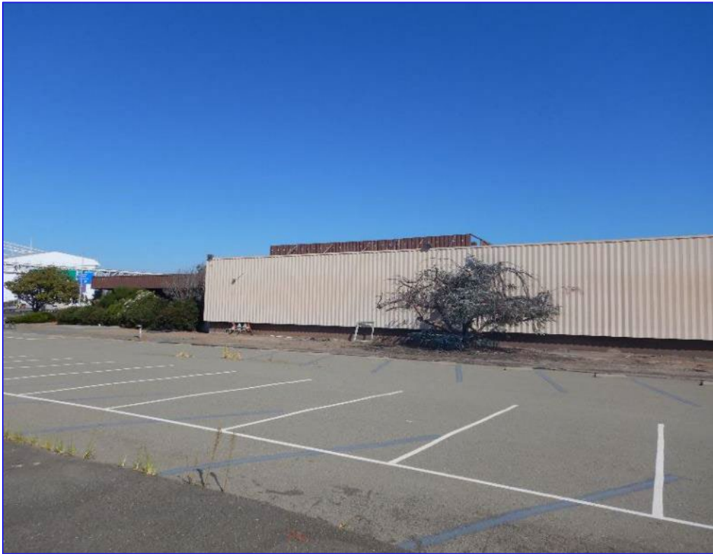
Photograph 13: Catering Building (M111), looking north
