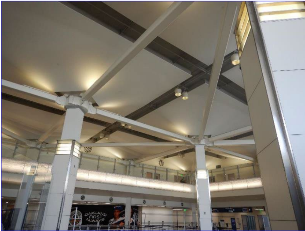
Photograph 9: M102 interior seismic improvements
