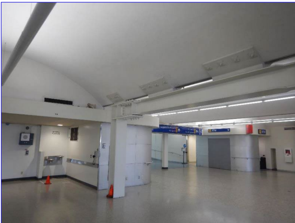
Photograph 8: Interior view of seismic improvements (M101)
