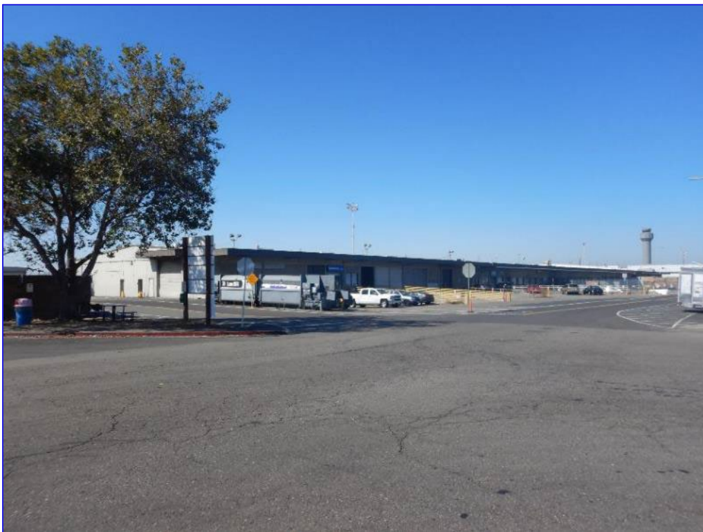
Photograph 12: Air Cargo Building (M106/M112), looking north
