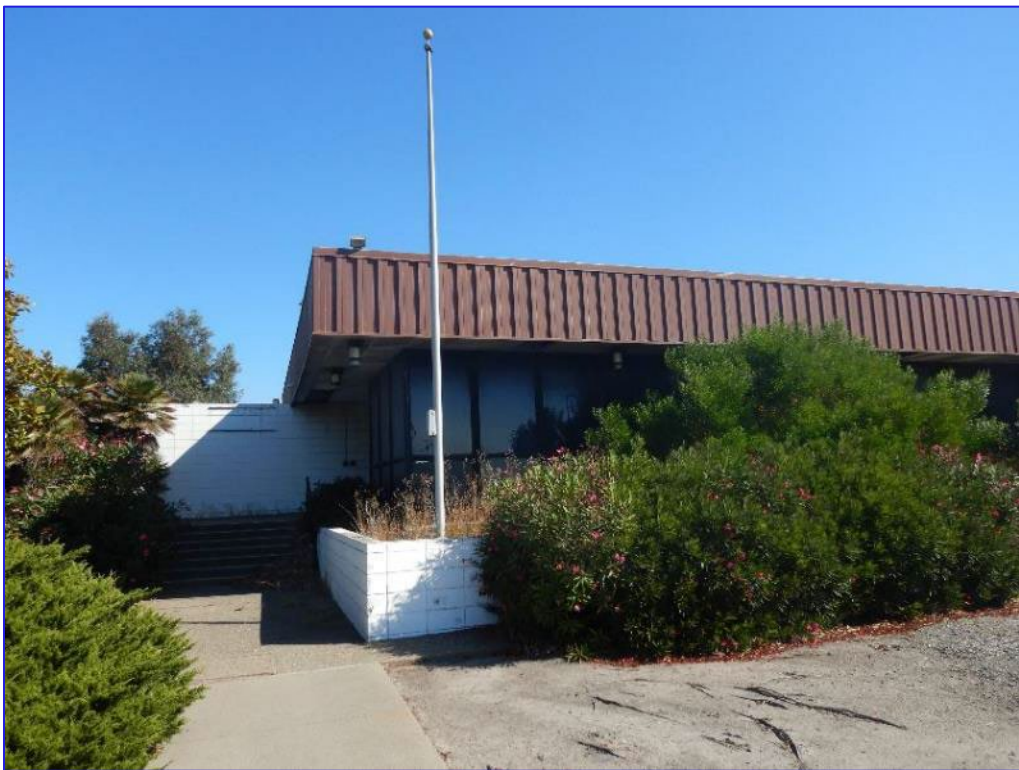
Photograph 14: Catering Building (M111), looking northeast
