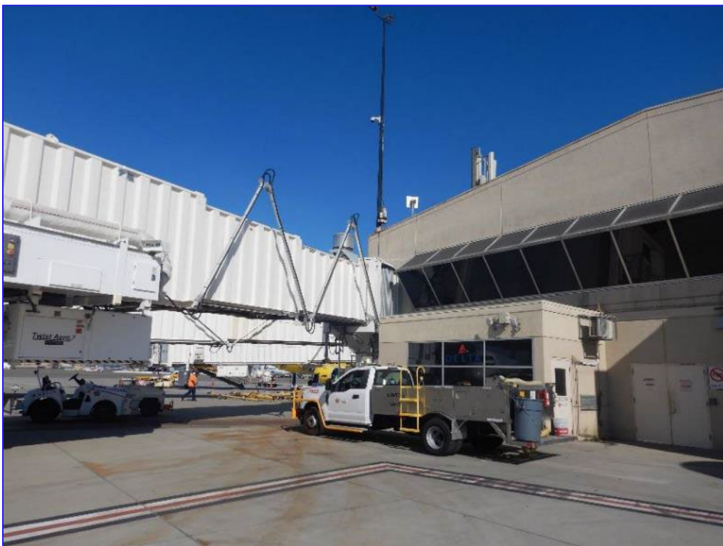
Photograph 10: M103, looking north (original 1 st Floor with various exterior modifications, 1980s addition of 2nd floor and passenger boarding bridge)
