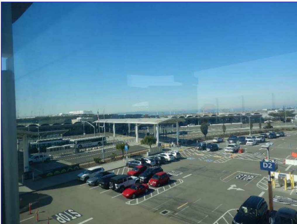
Photograph 2: Terminal 1 Overview, looking SW from BART station
