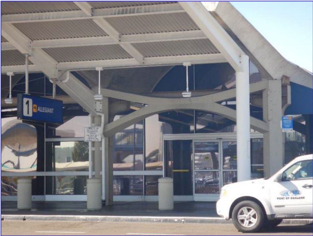
Photograph 5: Detail view of M101 entryway, looking SW
