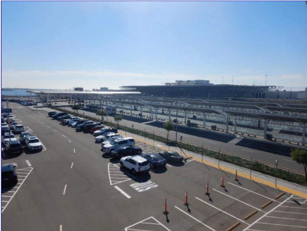
Photograph 3: Overview of Terminal 2, looking south from BART station
