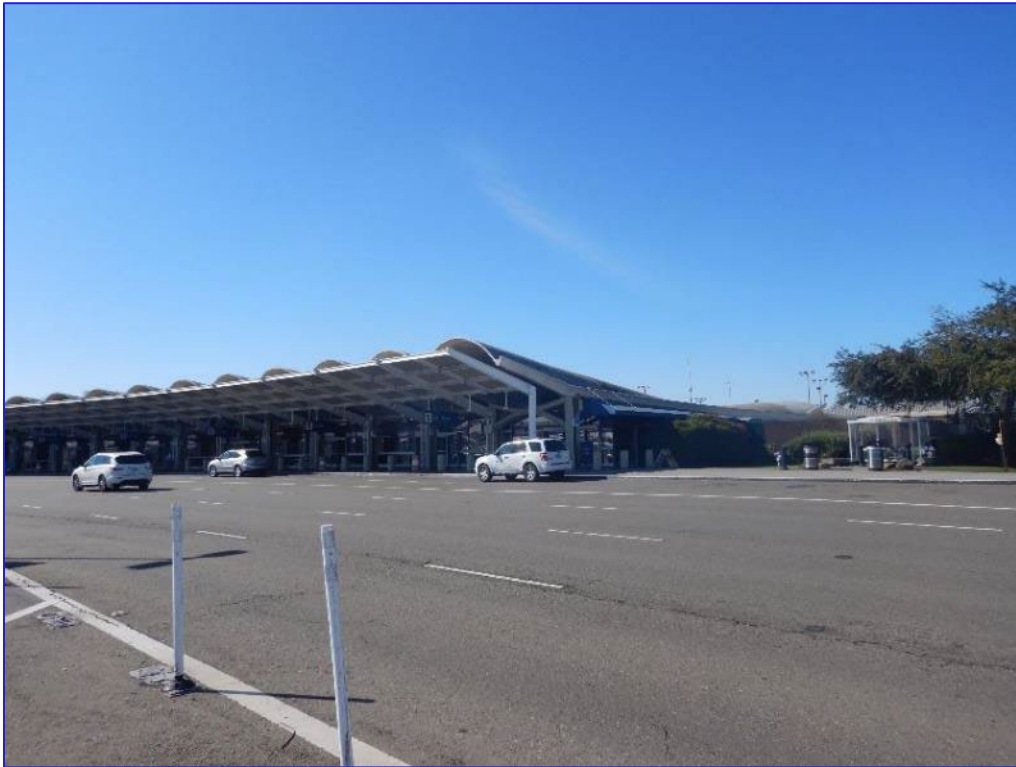
Photograph 1: Terminal 1 (M101), looking south
