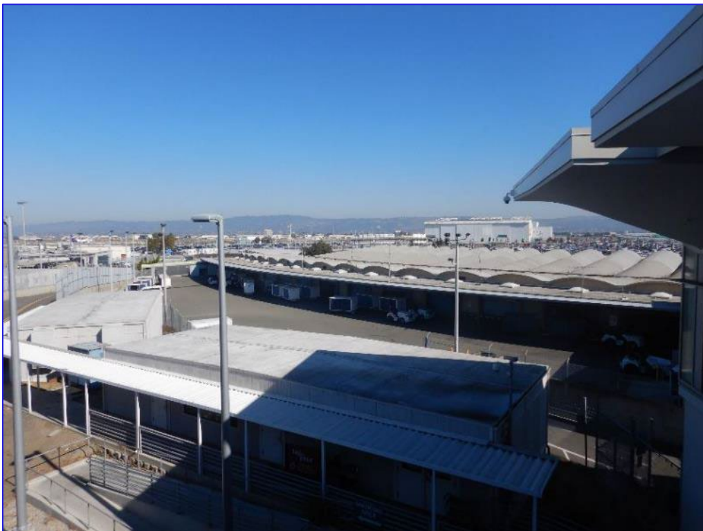
Photograph 4: Backside view of Terminal 1 (M101), looking NW from M102
