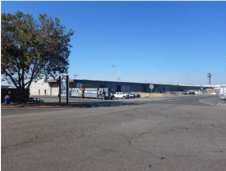
Figure 7. View of Air Cargo Building (M106) Facing West
