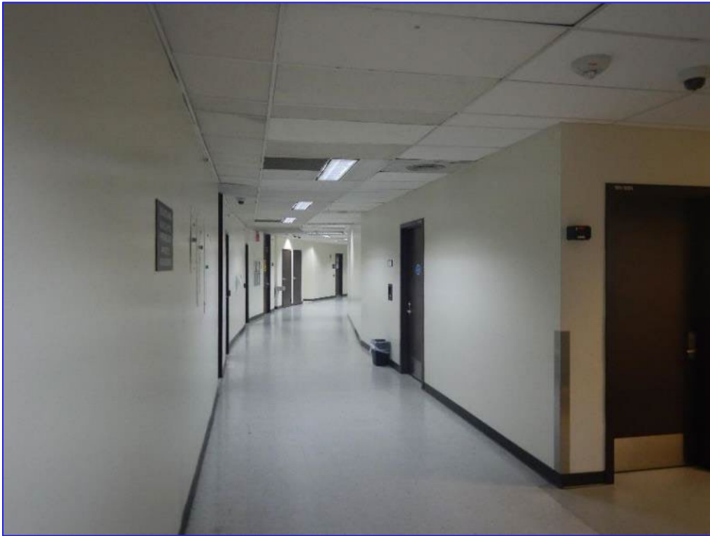
Photograph 11: Representative view of original M103 with interior modifications, looking north
