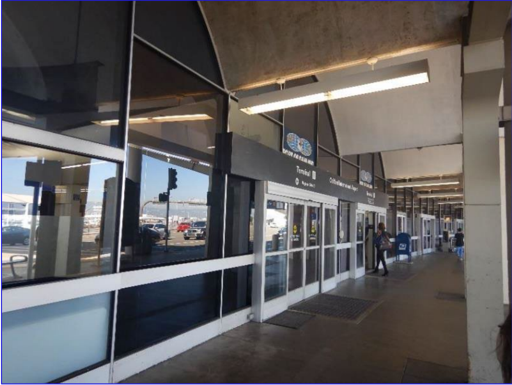
Photograph 6: Detail view of M101 entryway
