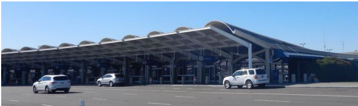
Figure 5. View of Terminal 1 (M101), Showing Ticketing and Baggage Claim Building
