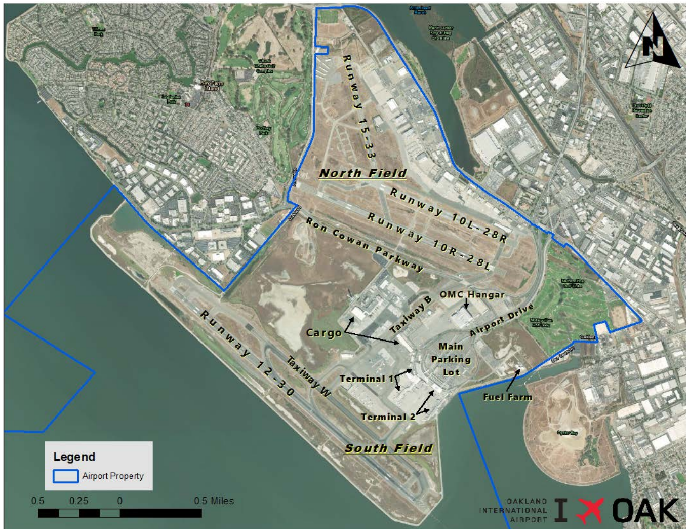
Figure 2 Existing Facilities at OAK
