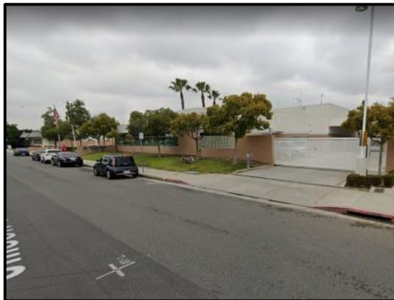
PHOTO 11: View looking northwest of the maintenance building at the existing TMF
