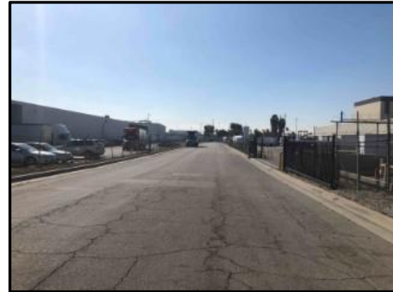
Photo 2: View facing south on project site driveway showing CNG tank at center and the closed CREF facility at right.
