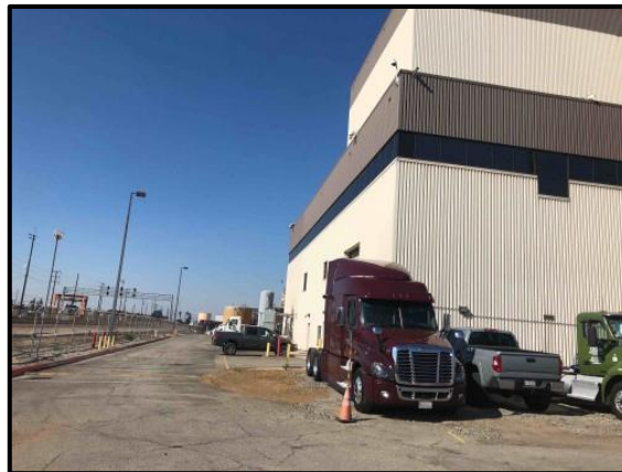
Photo 3: View looking west showing the closed CREF building to the right and the BNSF rail yard offsite to the south on the left.
