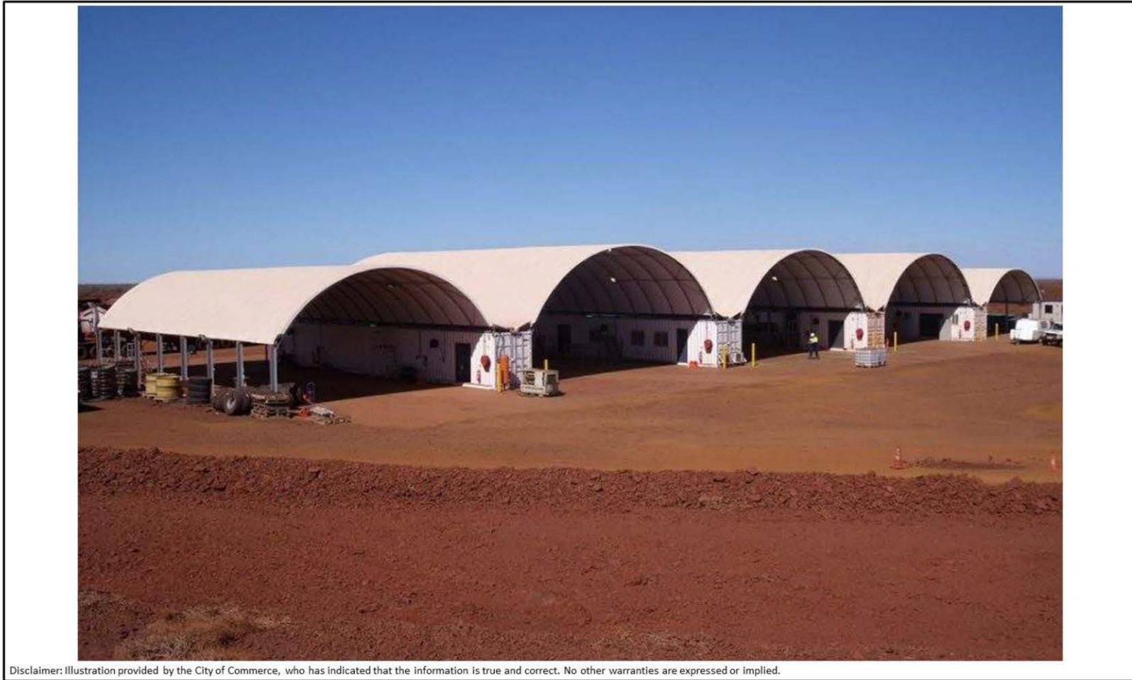
Figure 3.8-1 EXAMPLE OF MODULAR CONTAINER SHELTERS
