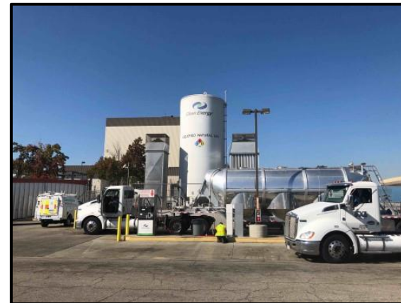
Photo 4: View looking west of the CNG fueling station in the east part of the project site; part of the closed CREF facility is in the background.
