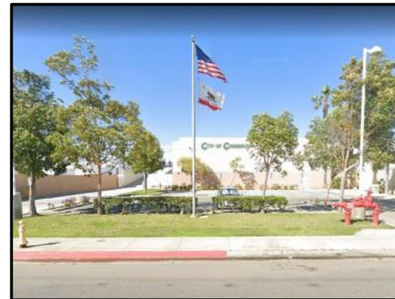
Photo 12: View looking north of the maintenance building at the existing TMF
