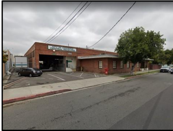
PHOTO 9: View looking northeast of the provisor (warehouse) building on the existing TMF site
