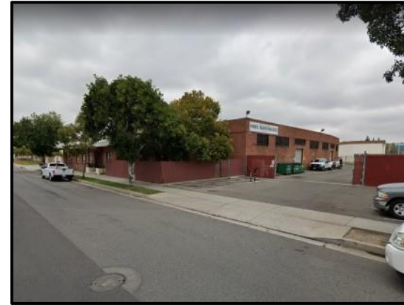
PHOTO10: View looking northwest of the provisor (warehouse) building on the existing TMF site
