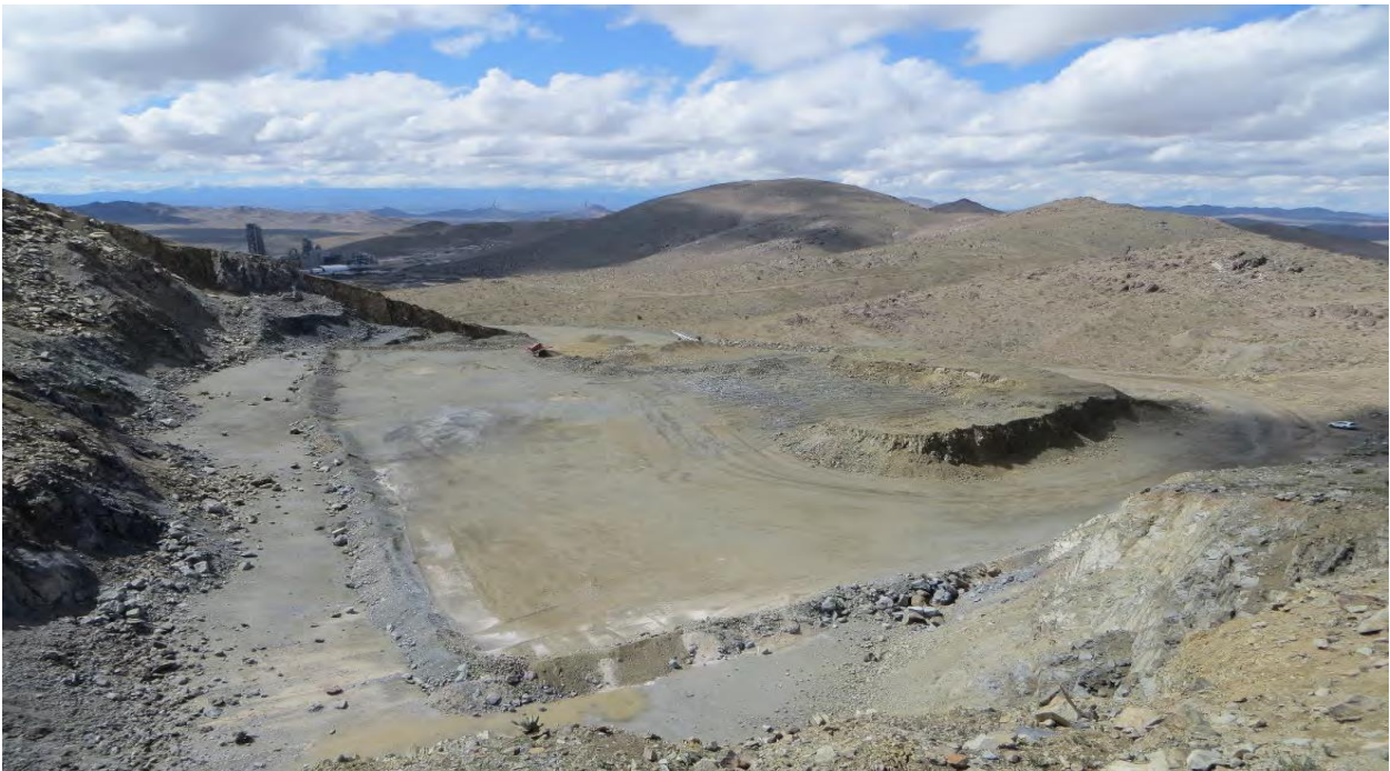
Photo 4: From the eastern portion of the project site looking west over the existing mine area. CEMEX cement plant in distance to west.
