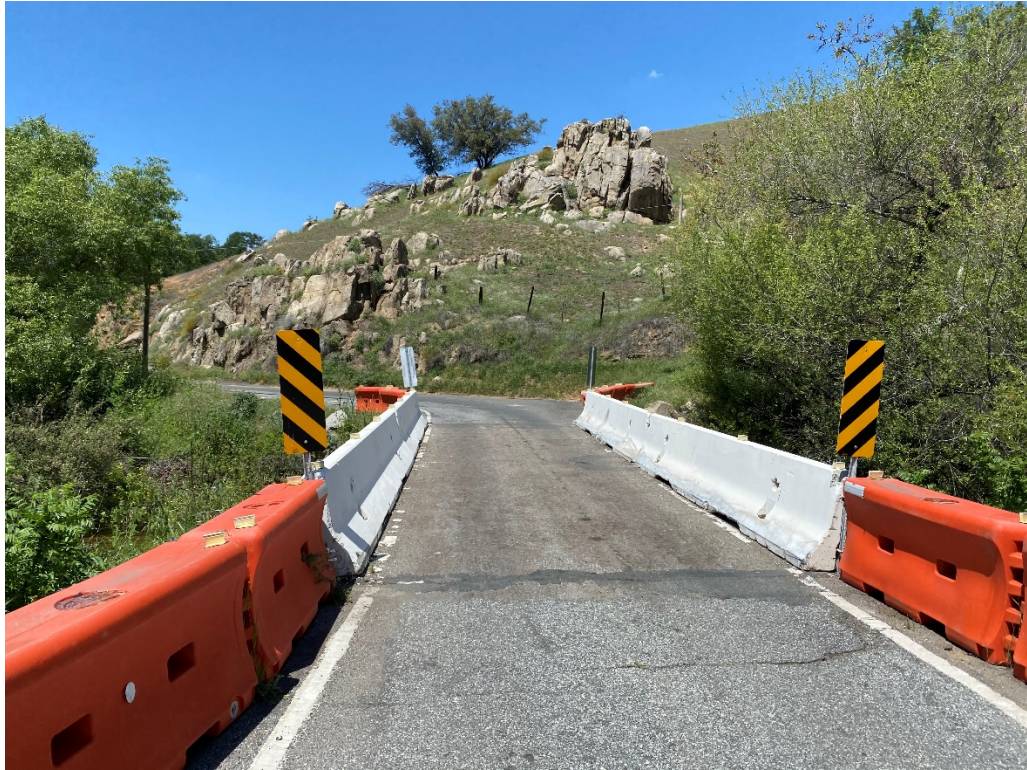
M109 over White River Bridge Replacement Project November 2020
