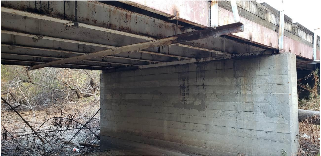
Photograph 5: Representative photograph of the existing bridge.
