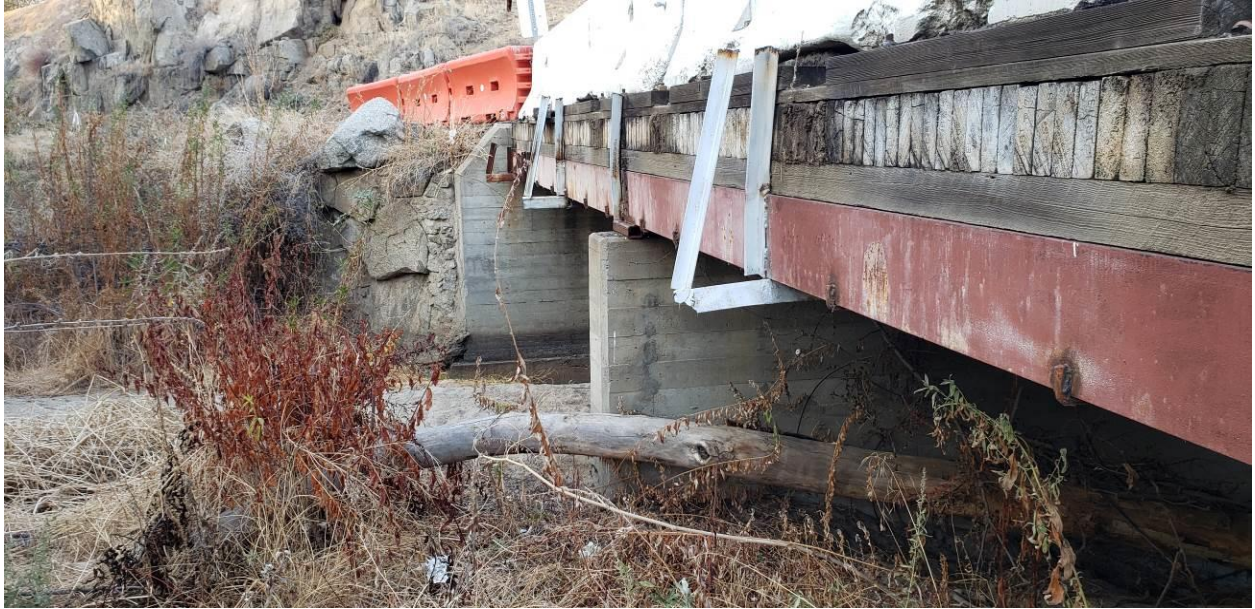
Photograph 3: Representative photograph of the existing bridge.
