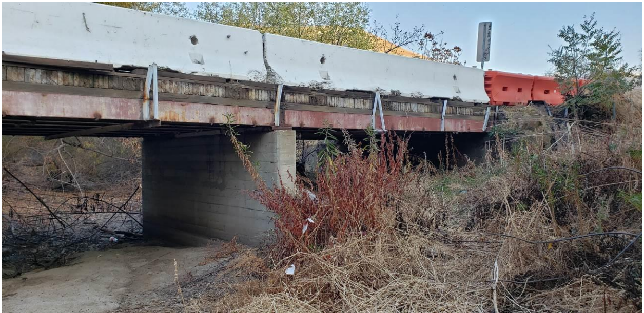
Photograph 6: Representative photograph of the existing bridge.
