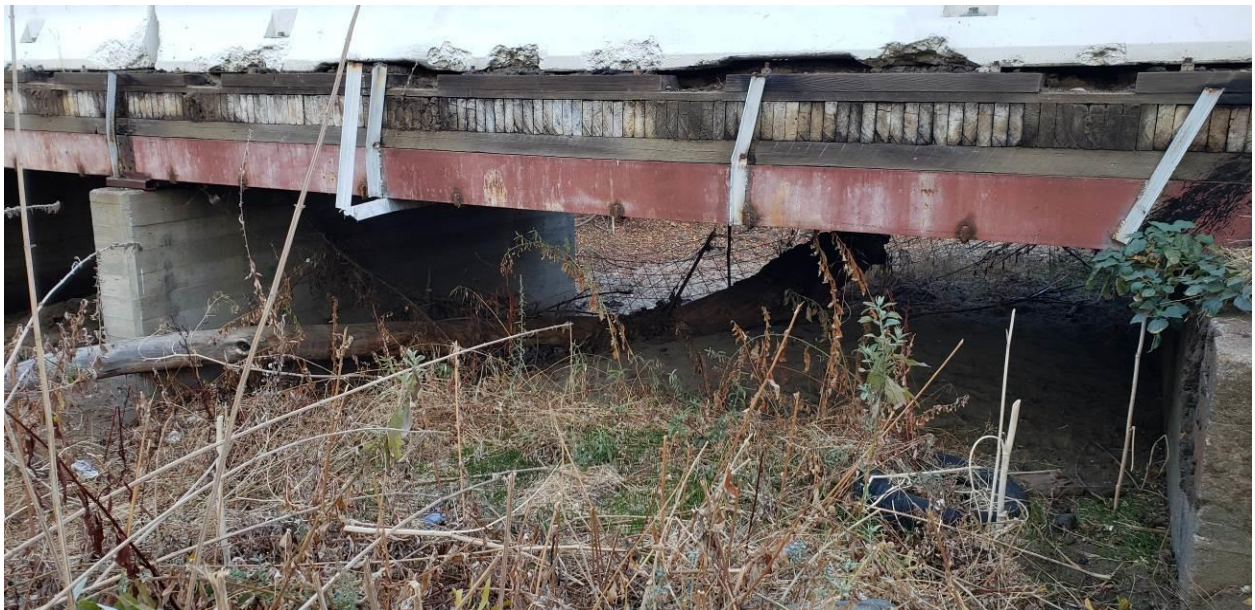
Photograph 4: Representative photograph of the existing bridge.
