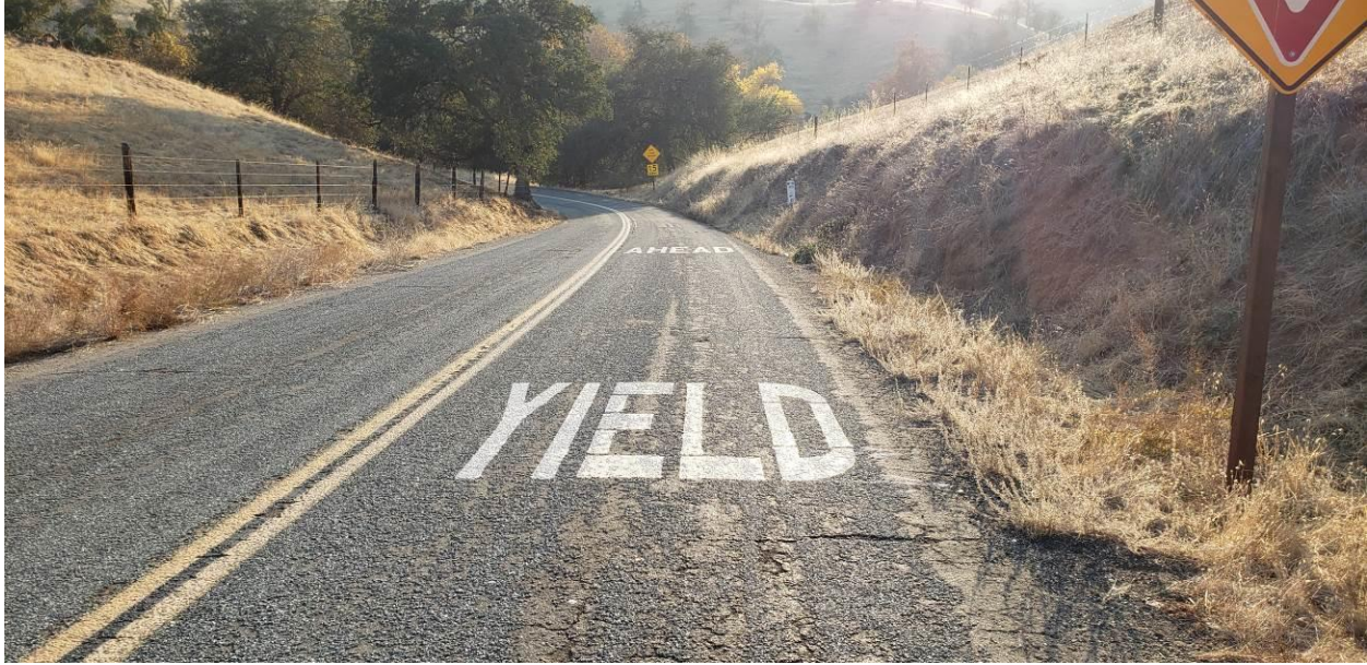
Photograph 1: Representative photograph of existing road looking south approaching the existing bridge.
