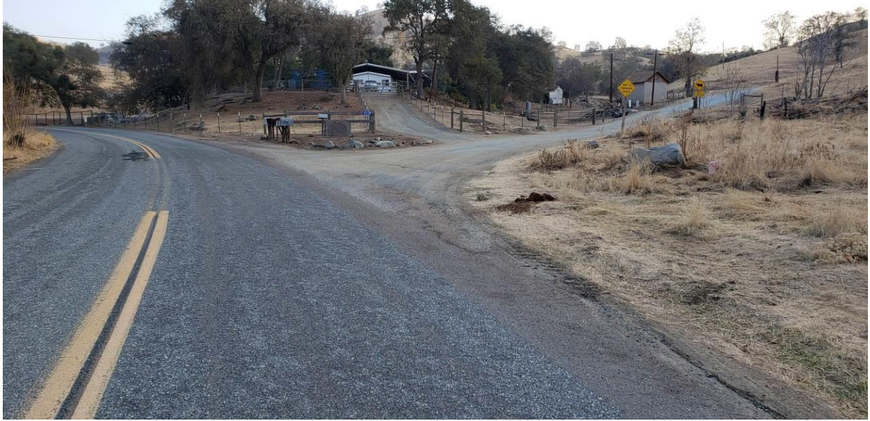
Photograph 9: Representative photograph of utility pole and transformer.
