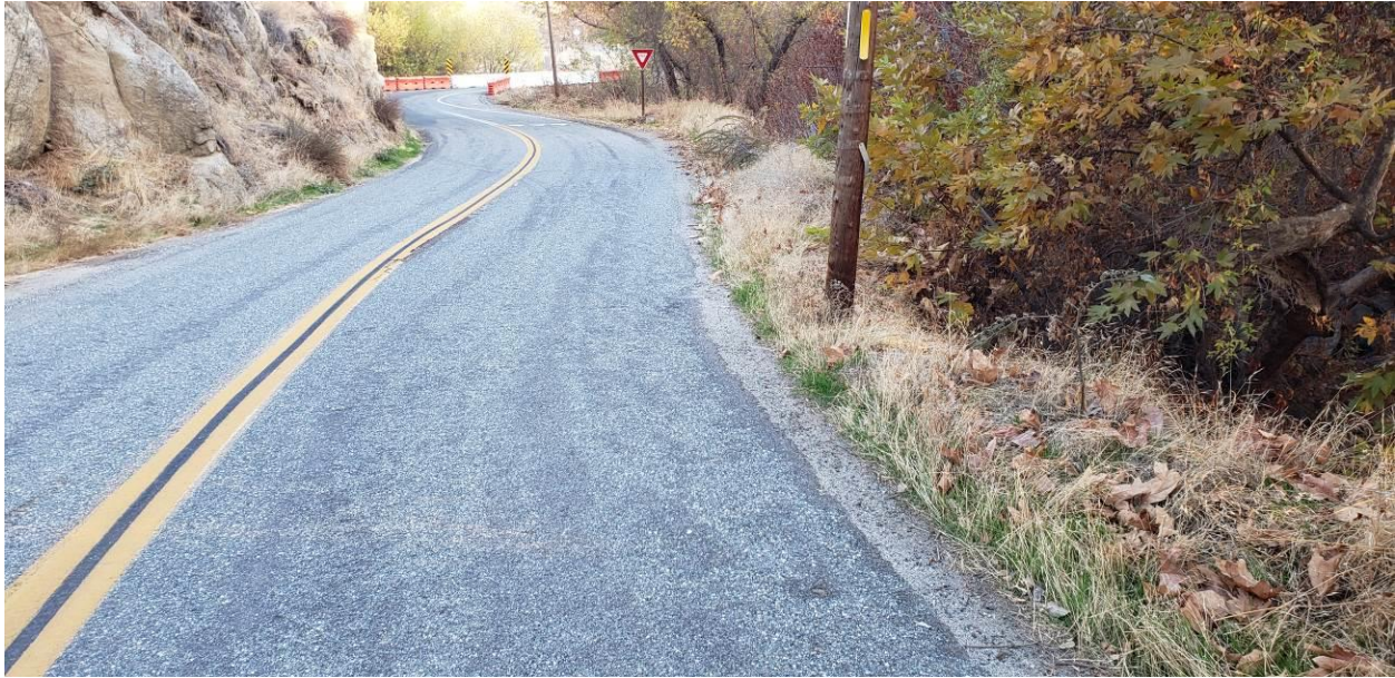
Photograph 2: Representative photograph of existing road looking south approaching the existing bridge.
