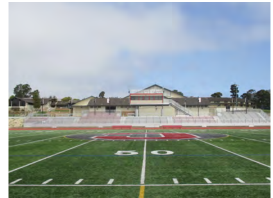
④ Carmel High School Stadium home bleachers and press box (from south looking north)
