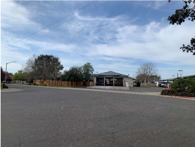
South-east of site facing north-west
