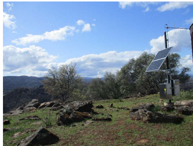
From site facing west
