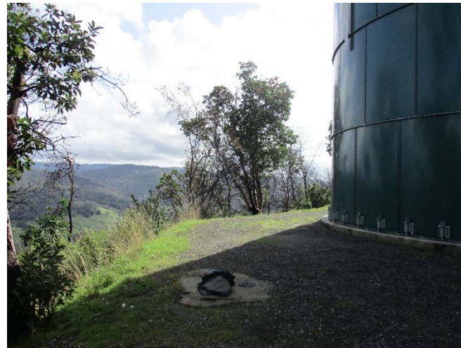
North of site facing south-east
