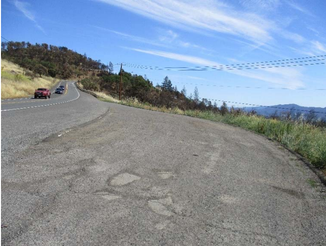
Site facing east
