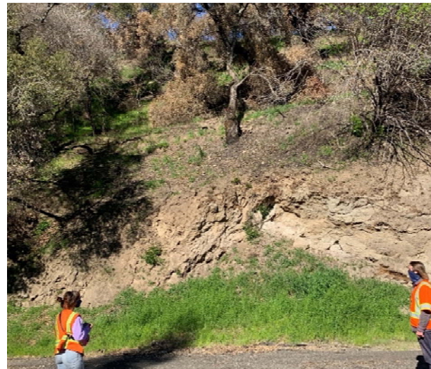
From site facing north
