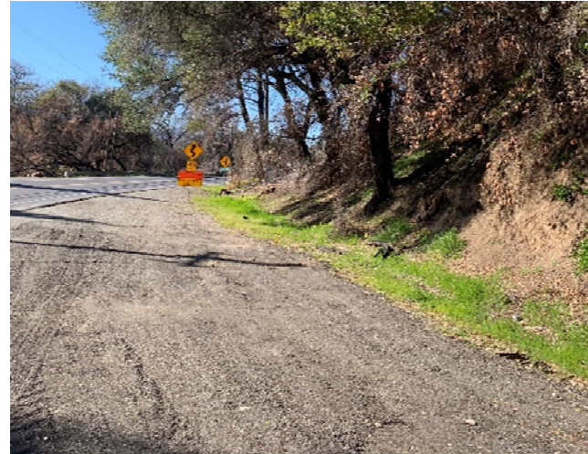
From site facing west
