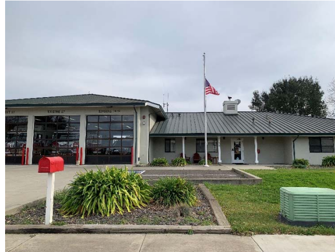
North-west of site facing south-east
