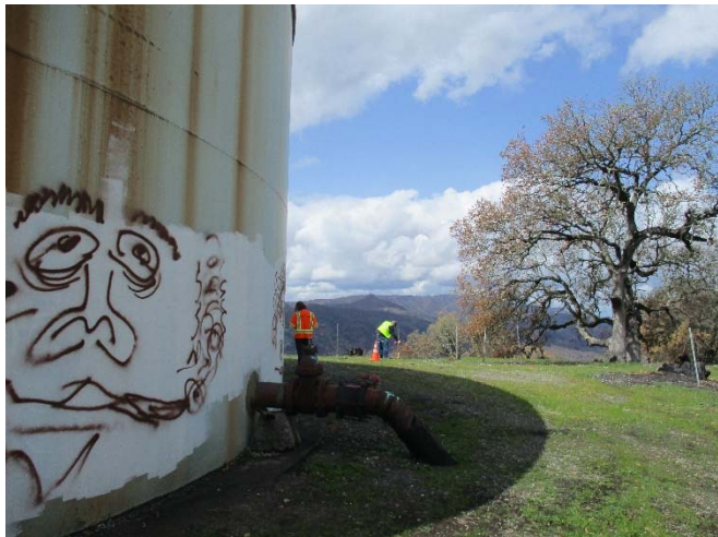
South-east of site facing north-west
