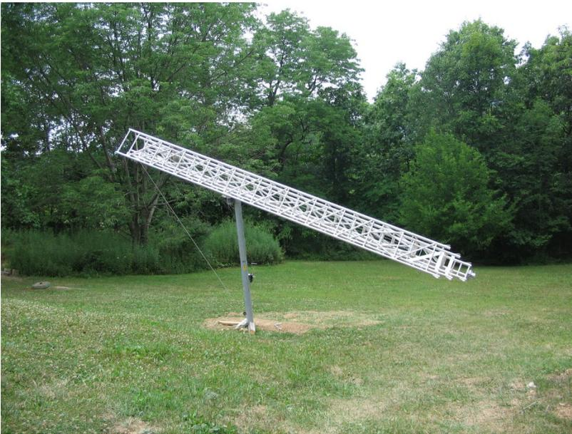
Sample Retracted Telescoping Lattice Tower Set on Center Support Pole
