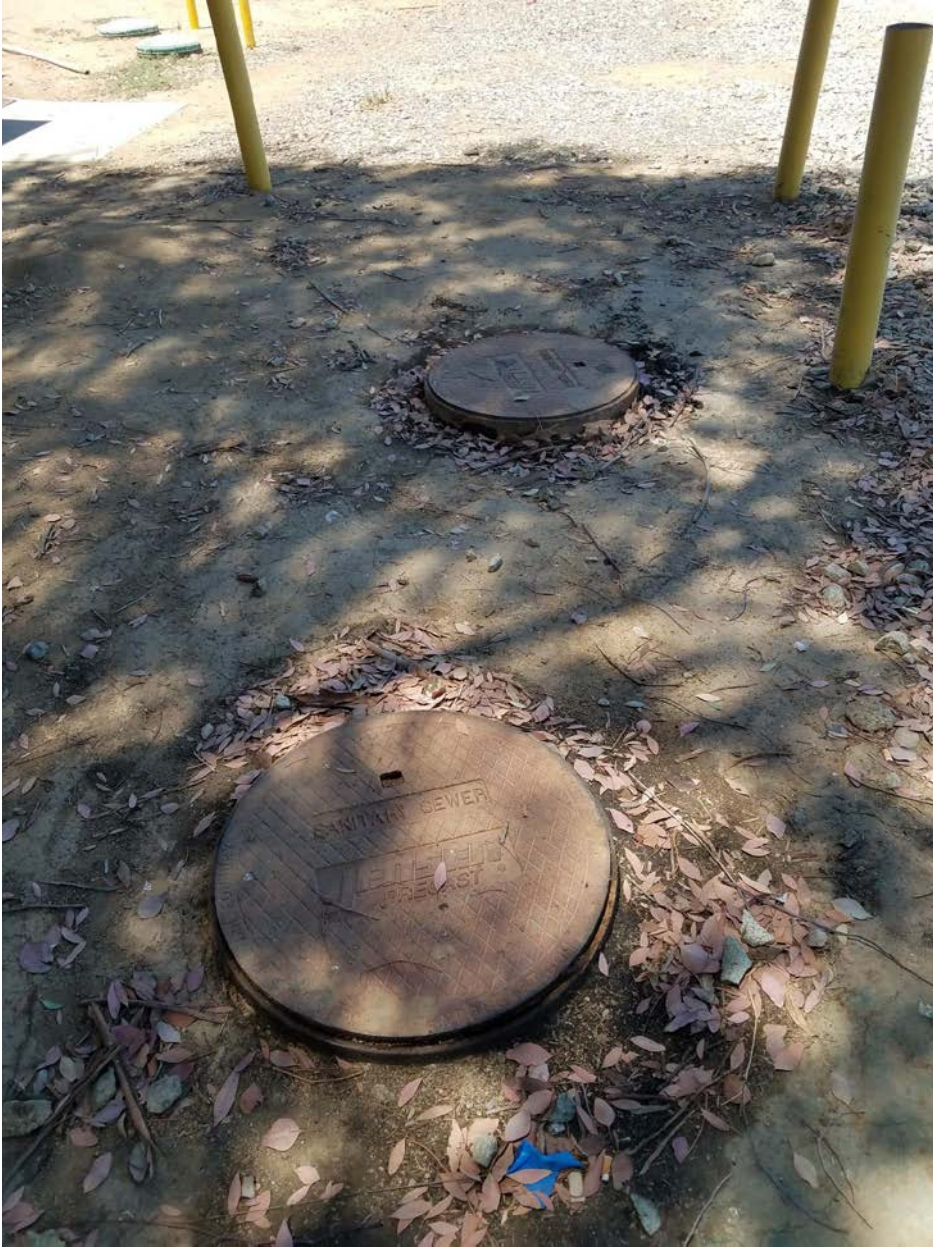
Appears to be septic or restaurant clean out grease trap.
