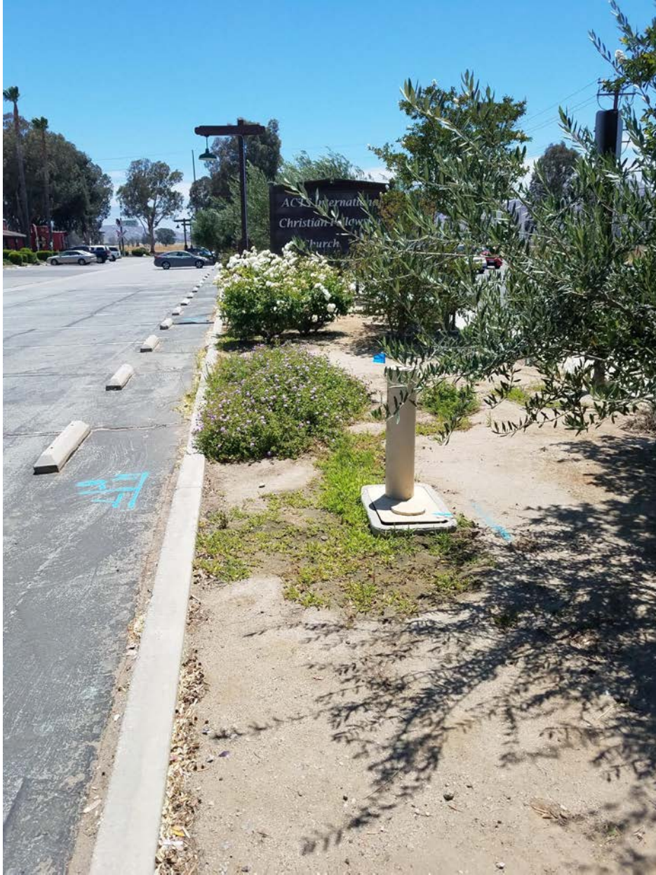
View looking east at water utilities in landscape adjacent to Highway 74.
