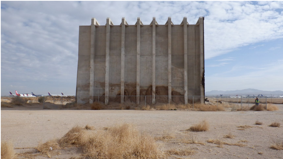
Photograph 11. View northeast of the southwest elevation of Facility 811.
