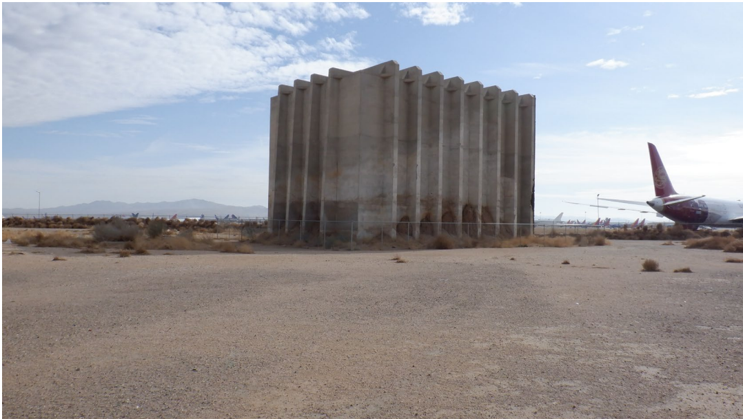
Photograph 10. View east of the northwest and southwest elevations of Facility 811.
