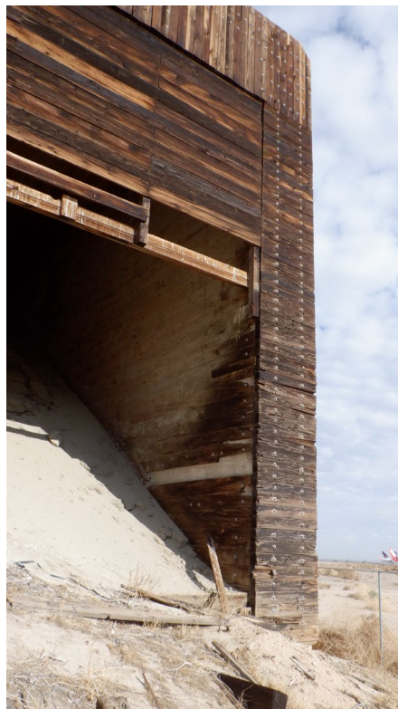
Photograph 14. View north of timber interior and exterior wall-cladding.
