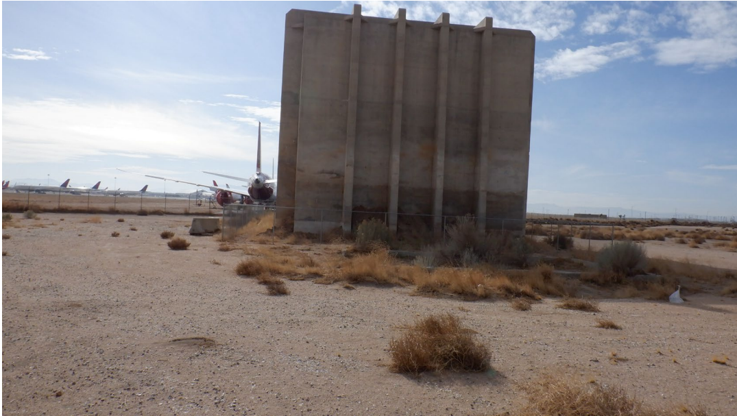
Photograph 9. View southeast of the northwest elevation of Facility 811.
