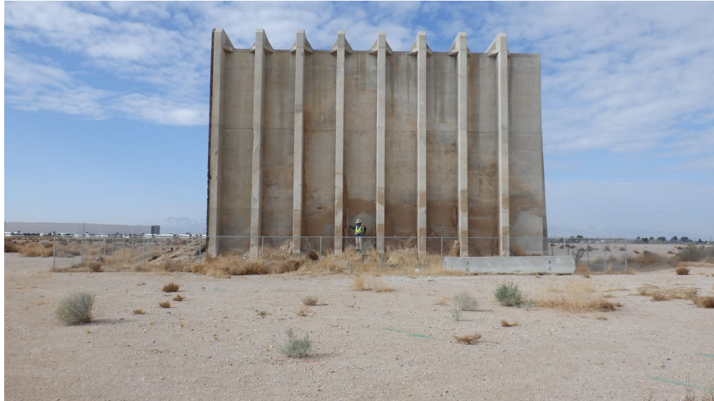
Photograph 7. View southwest of the northeast elevation of Facility 811.
