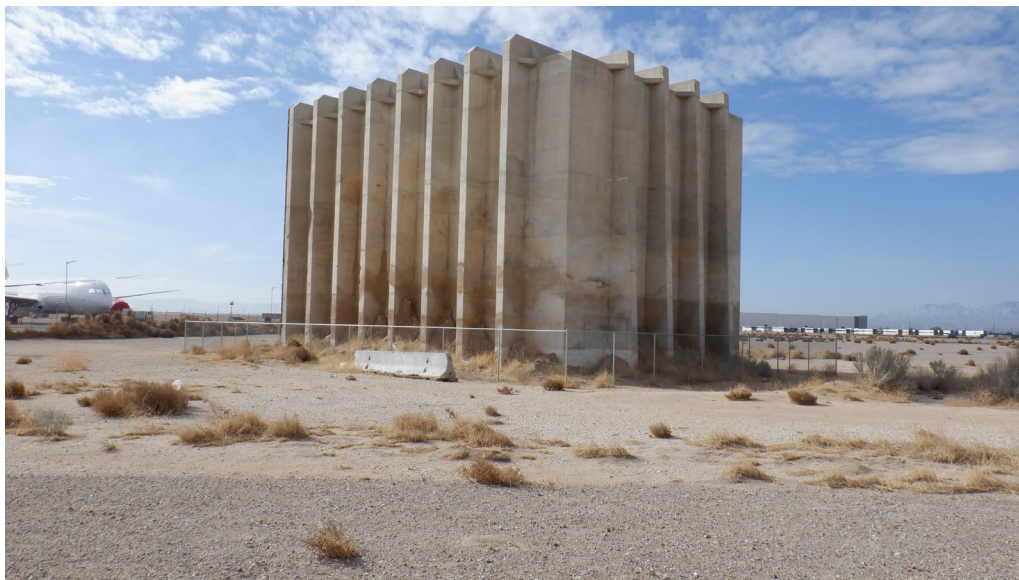
Photograph 8. View south of the northeast and northwest elevations of Facility 811.
