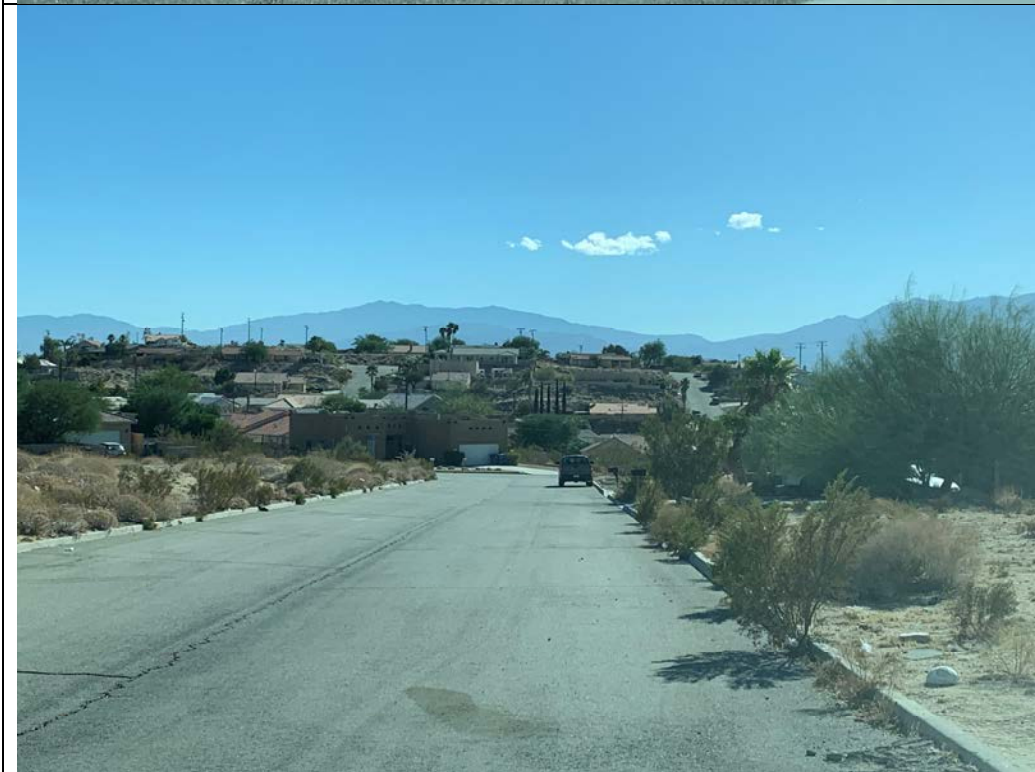
Photo 8. Project alignment near the southwest portion of the Project Area; south of Hacienda Avenue.
