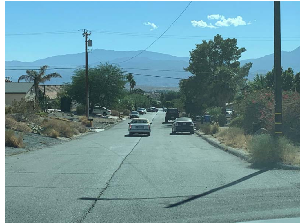
Photo 7. Project alignment near the eastern portion of the Project Area; south of Hacienda Avenue.
