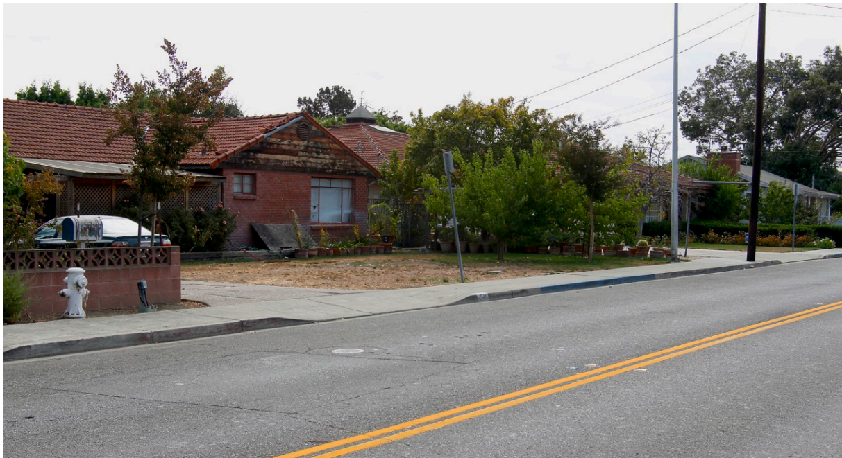
b) Existing residential development opposite (south of) project site
