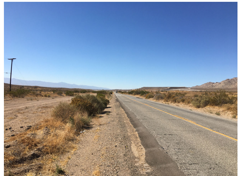
Photo 4 Description: Middle of alignment looking southwest
