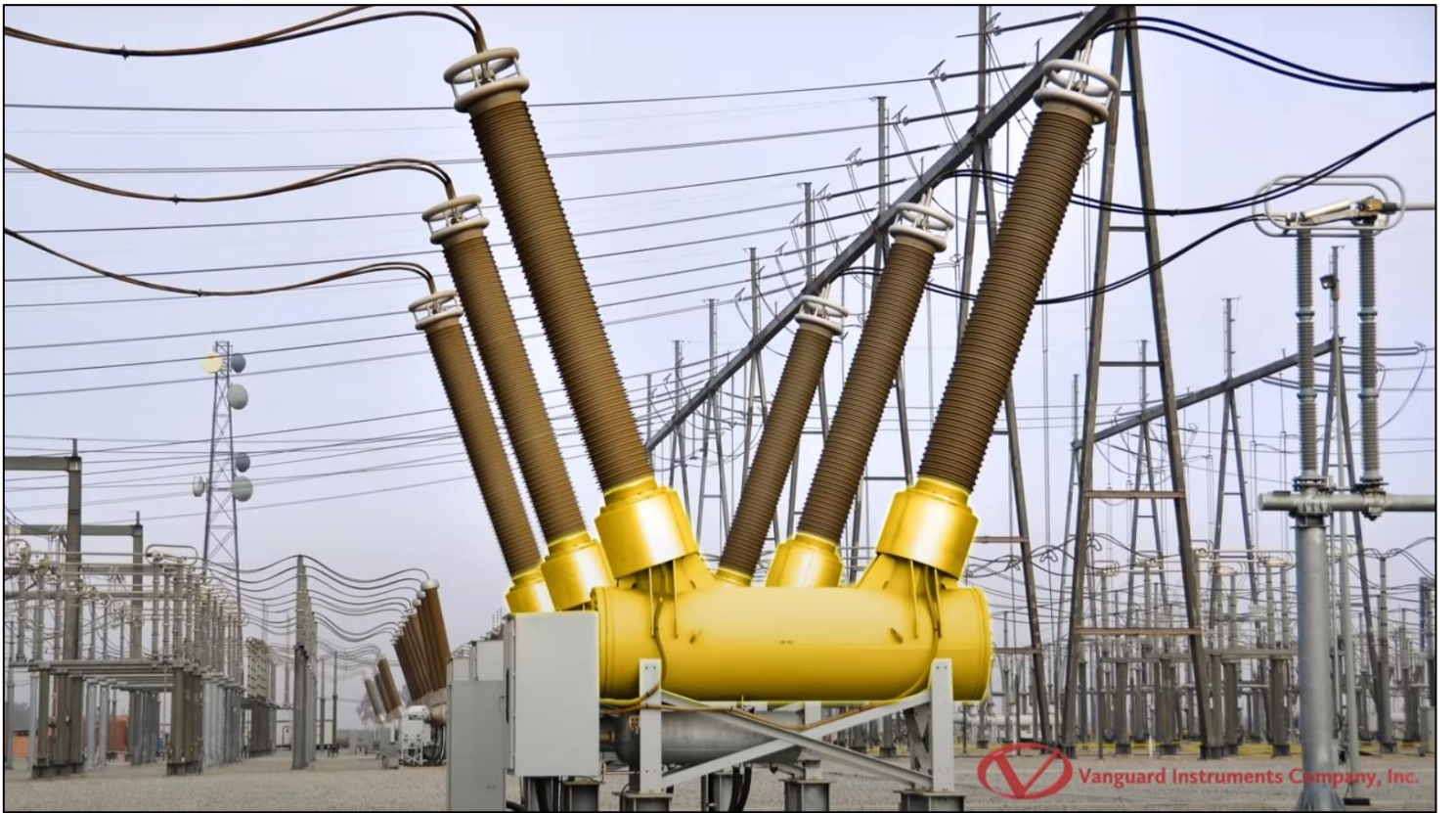
Avenue 42 Substation Breakers Replacement CANO and CESO Project (No. 30035644)
