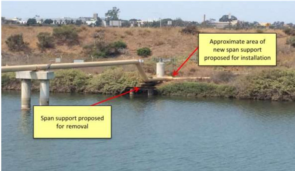
FIGURE 2. VIEW WEST ACROSS ATASCADERO CREEK FACING THE SPAN SUPPORT REMOVAL/REPLACEMENT LOCATION. NOTE THE WOODEN SPAN PROPOSED FOR REMOVAL IN THE CENTER OF THE PHOTO.
