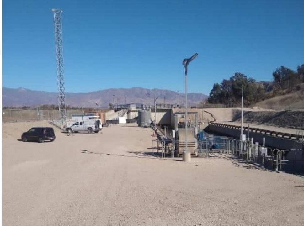
Photo 1: Facing northeast from the middle of Upland Work Area 1 (January 14, 2021).
