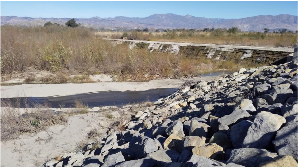
Photo 12: Facing north at the Downstream Work Area from the boundary of Upstream Work Area 1 (January 14, 2021).
