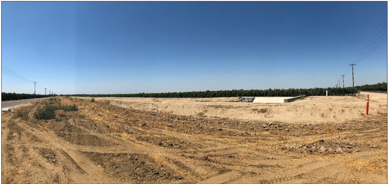
Photograph 2: View of the northeast corner looking southeast.
