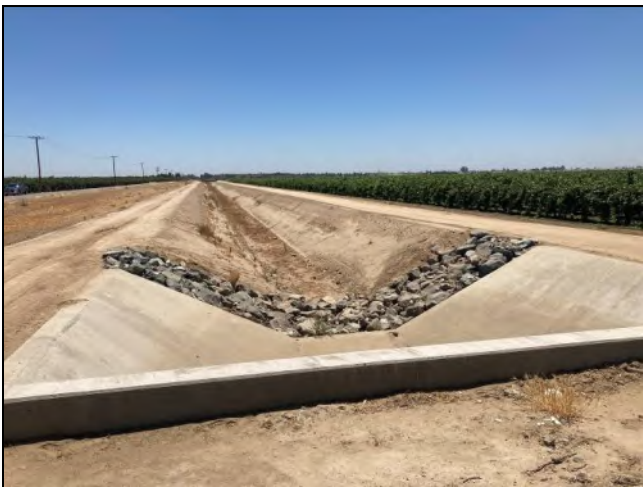
Picture 5: Canal along the eastern border of the Subject Property.
