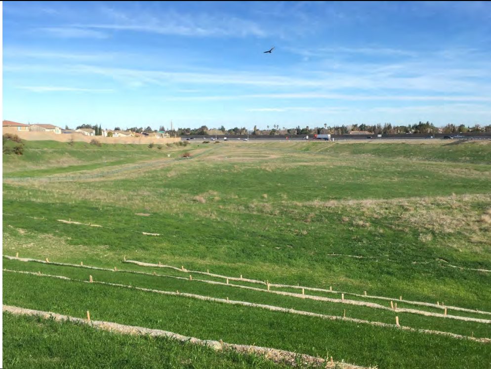
1. Facing north, the photo depicts an overview of the Survey Area. Road extension work was actively occurring during the time of the survey, and the adjacent area just south of the Property has been recontoured as seen in the foreground, delineated by erosion control wattles.
