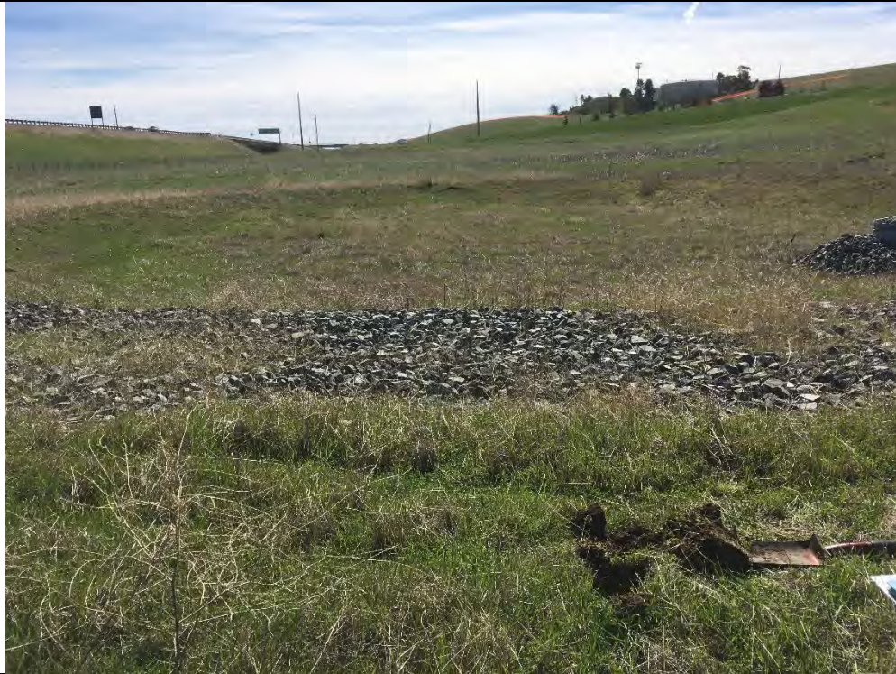
9. Facing south, the photo depicts an overview of the detention basin. In the foreground, the gravel and rock layer that surrounds the basin perimeter can be seen. The shovel in the lower right corner marks the upland sample point 5A.
