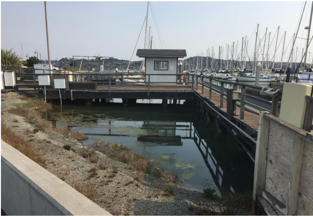
Photo 11. View of entrance to Basin 3, including gate and dock house, with utility lines and boxes affixed to side of dock, looking east.
