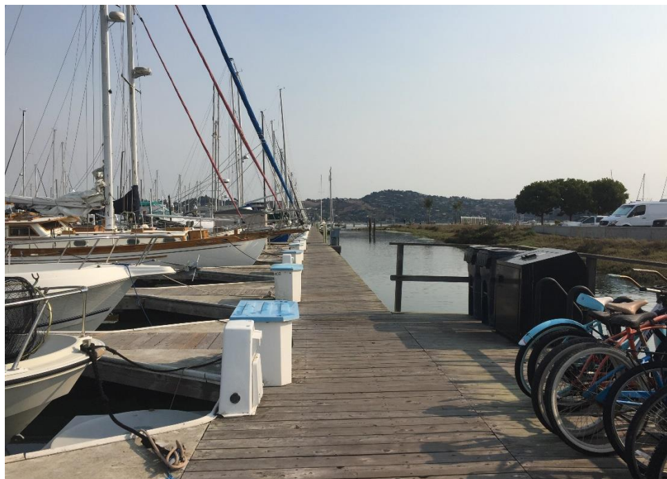
Photo 4. View of dock deck with bike rack, waste receptacles, dock boxes, and podiums, looking northeast. (MIG site visit, 9/29/2020)
