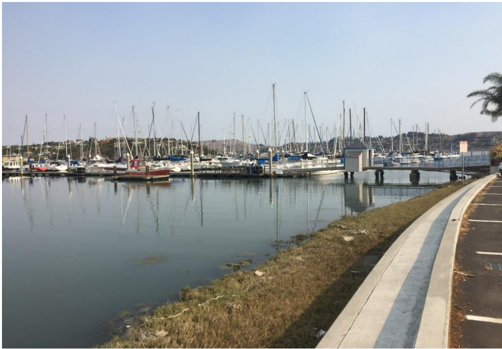
Photo 15. View of Basin 4 entrance and docks, including gangway and dock house, from marina parking lot, looking north. (MIG site visit, 9/29/2020)
