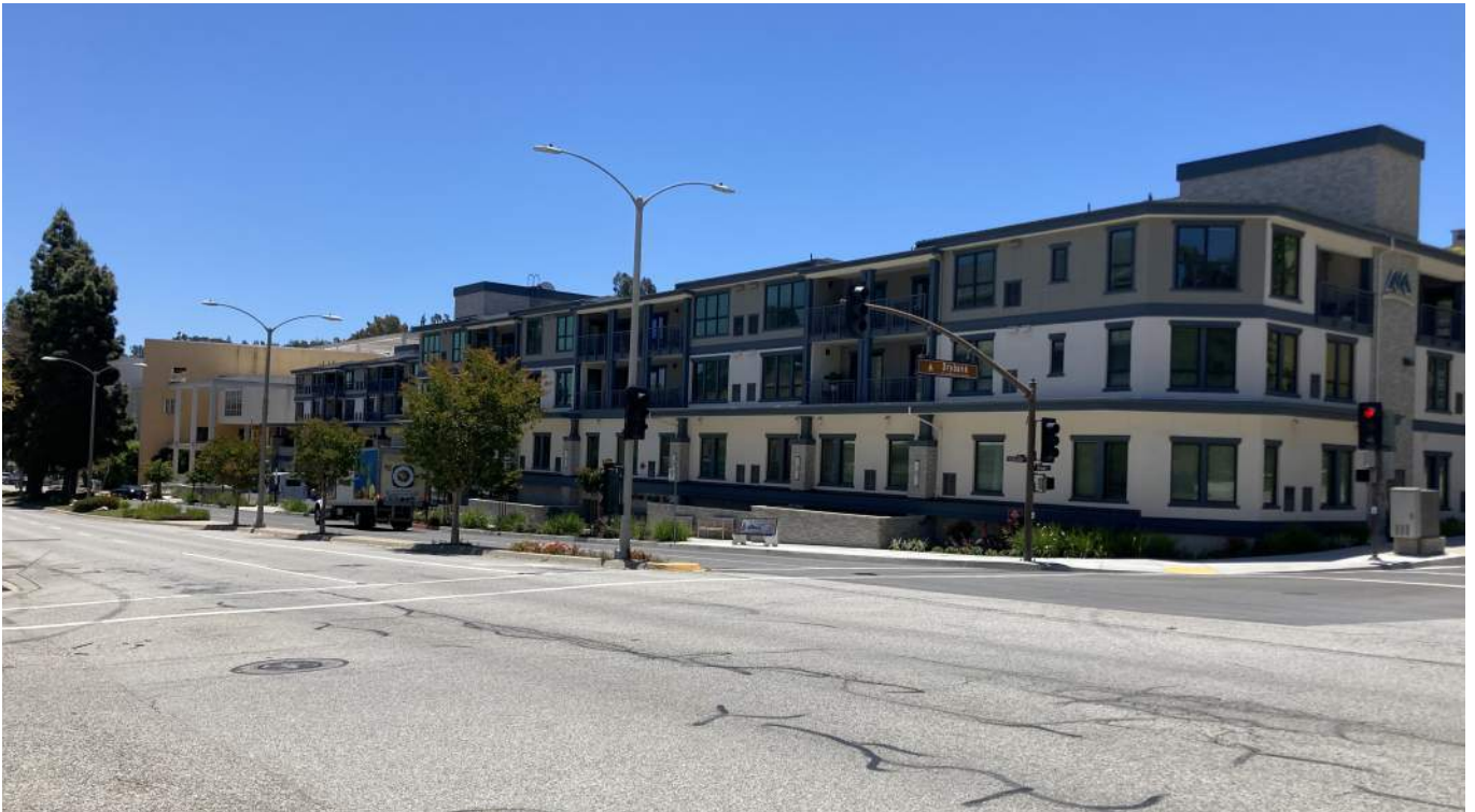
View of the Merrill Gardens Senior Housing complex on the southeast corner of Silver Spur Road and Drybank Drive, looking south.
