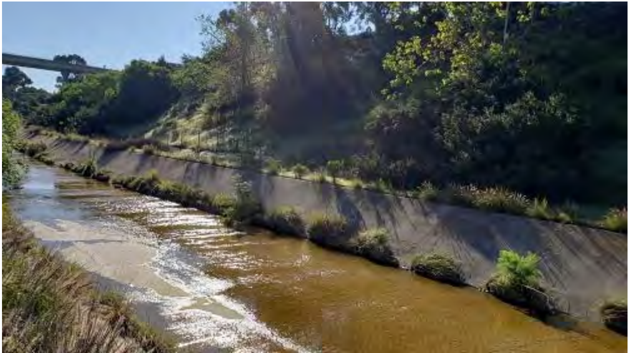
Photo 3. Chollas Creek, looking upstream. I-805 overpass visible from upper left in photo.
