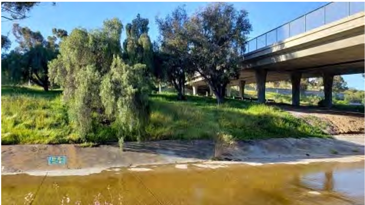
Photo 6. View of Chollas Creek adjacent to Home Avenue Bridge, looking south.
