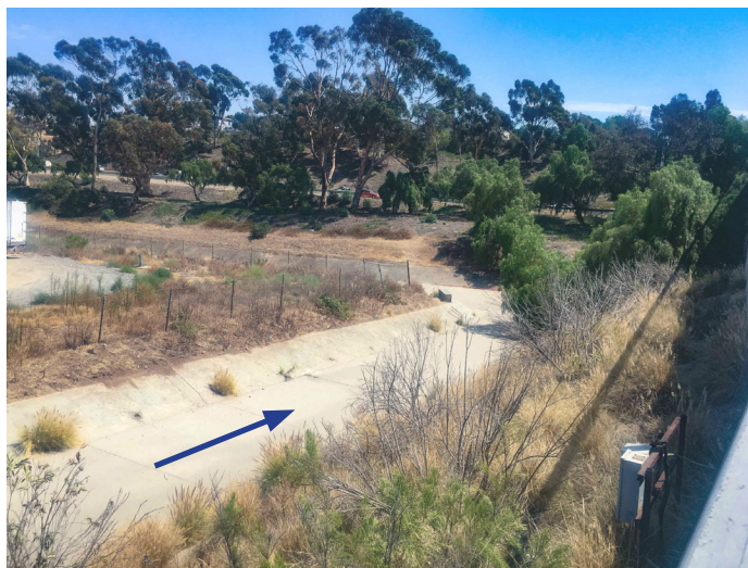
Figure 4: Existing Home Avenue Channel at Confluence
