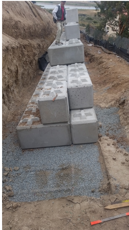
Figure 10: Typical Enviro-Block Wall Installation
