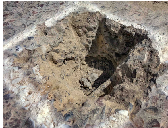
Figure 9: Channel Bottom Boring
