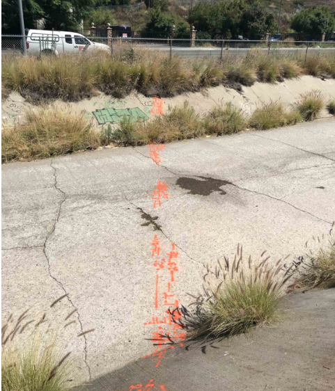
Figure 7: Markout from Duct-Rodding
