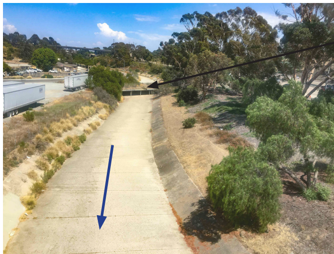
Figure 3: Existing Channel - Downstream
