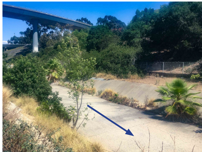
Figure 2: Existing Channel - Upstream
