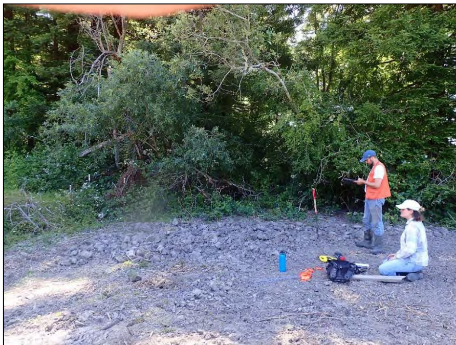
Photo 4 – View of the area adjacent to the western property line and central drainage ditch (Photo June 17, 2019).
