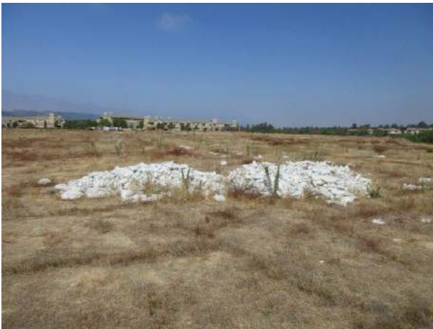
9. View of sandbags containing rocks on the central portion of the subject property.
