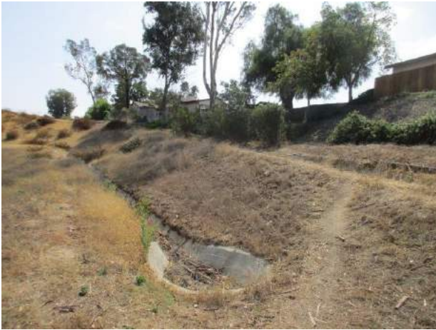
7. View of engineered stormwater drainage on the southern side of the subject property.
