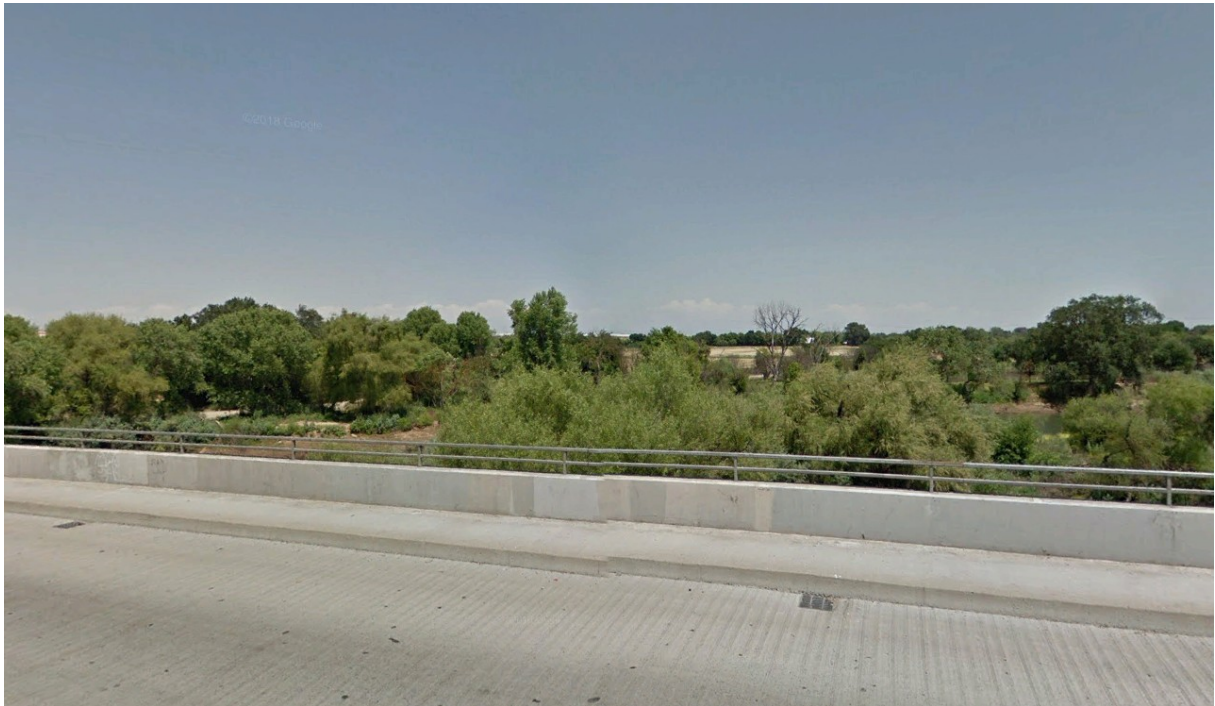
Figure 2.2-14. View from Mitchell Road Bridge looking east after improvements.
