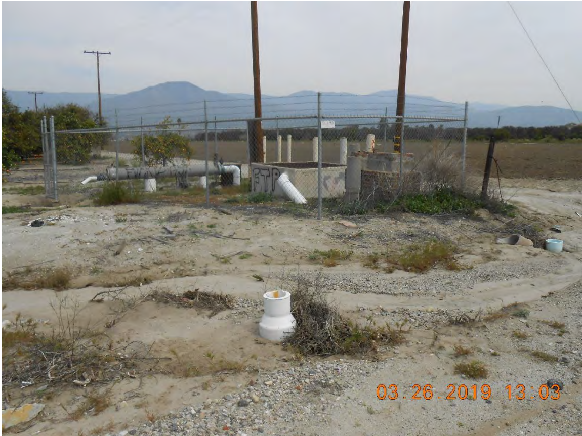
Northerly view of idle water well near the southeast corner of the subject property.
