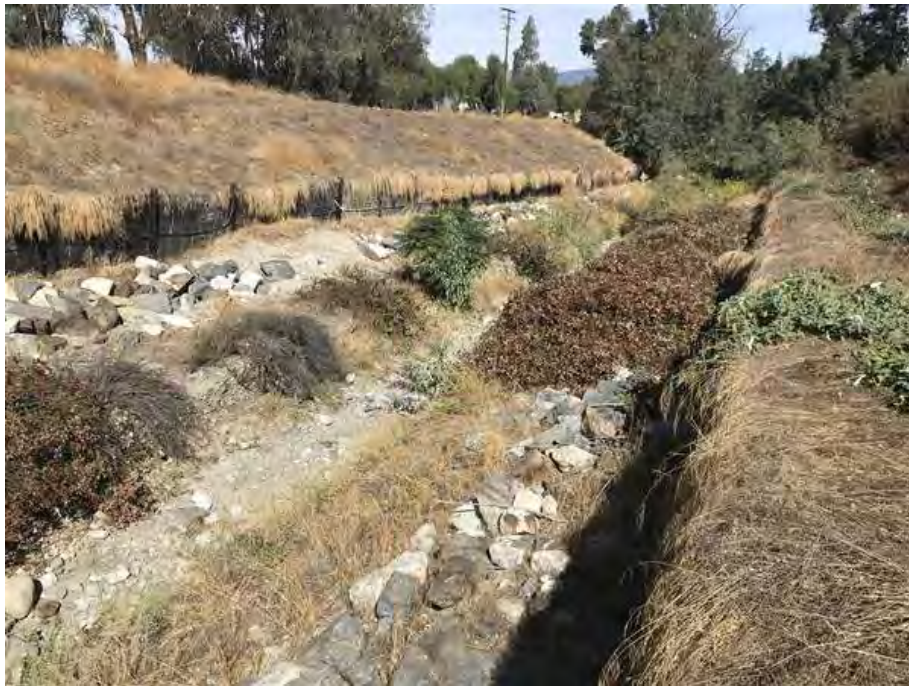
Photograph 1: View of the off-site drainage looking downstream.
