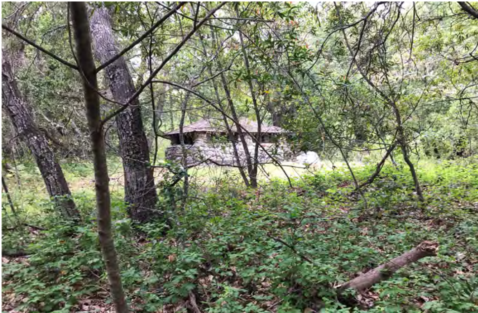
Photo 1. Looking north towards existing PBSSP facilities.
