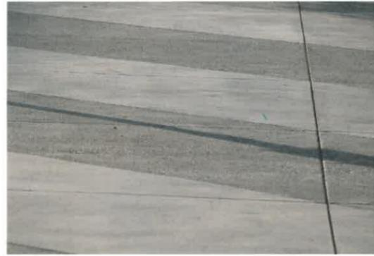
**CONCRETE PAVING WITH ALTERNATING FINISH**
