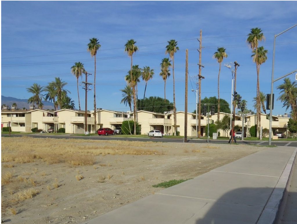
Photograph 5: Looking southwest towards the southeast corner of the intersection of Requa Avenue and Monroe Street.
