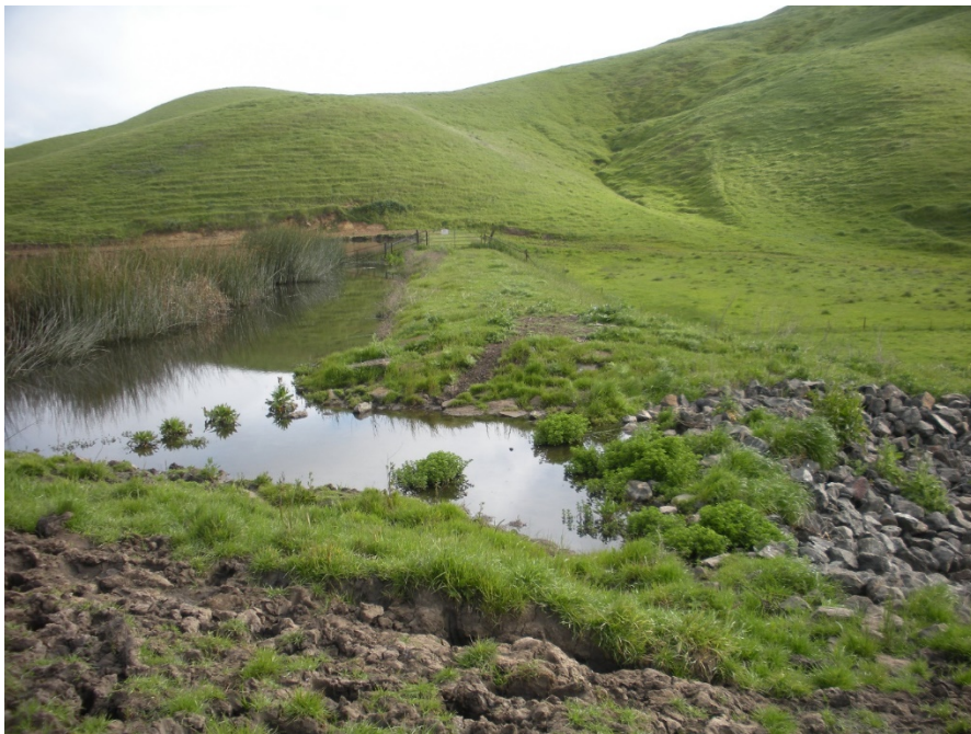
Figure 2. Lynch Canyon Dam spillway.
