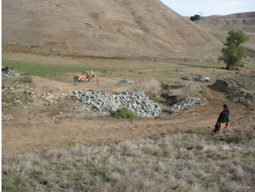
Figure 11. Emergency spillway repairs conducted at Lynch Canyon Reservoir in November 2006.
