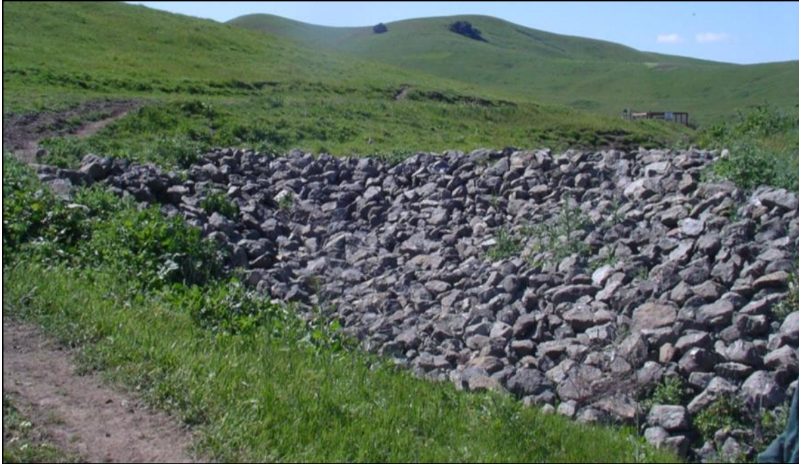
Figure 17. The Lynch Canyon Reservoir spillway.
