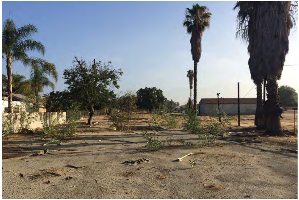
View 1. Taken from southwest corner, facing north. Showing concrete pads and the gas pump building.
