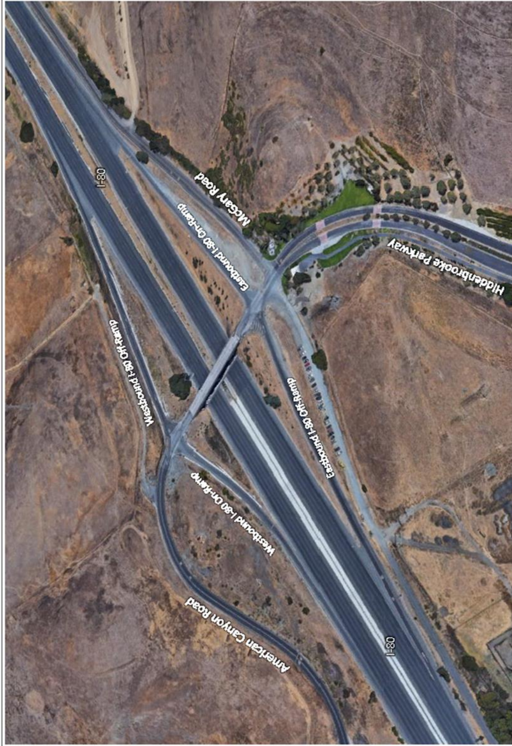
I-80/Hiddenbrooke Parkway Interchange
