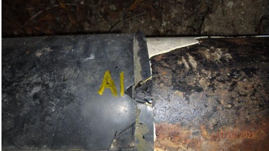
112321-ELLWOOD-A1 Black Pipe Wrap and Mastic (No Asbestos Detected)
