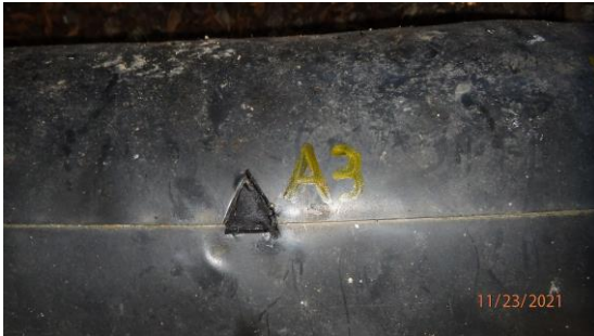
112321-ELLWOOD-A3 Black Pipe Wrap and Mastic (No Asbestos Detected)
