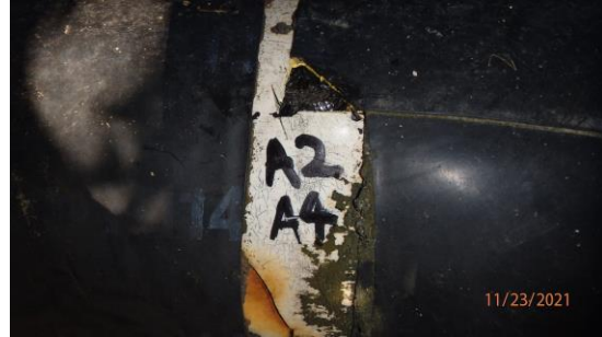
112321-ELLWOOD-A2 White Pipe Wrap and Mastic (No Asbestos Detected)
