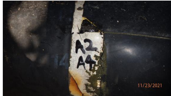
112321-ELLWOOD-A4 White Pipe Wrap and Mastic (No Asbestos Detected)
