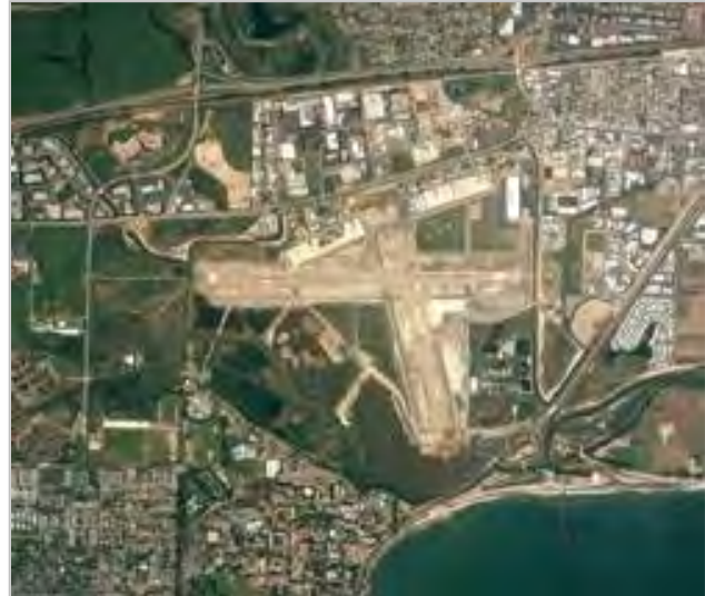
Aerial Photograph of the Santa Barbara Municipal Airport
