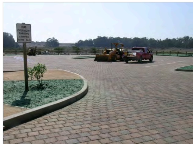
Coastal Access Parking at Santa Barbara Shores Park
