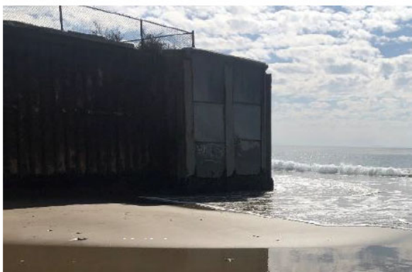
Low sand level – Mar 2020 at 0’ to 3’ tides
