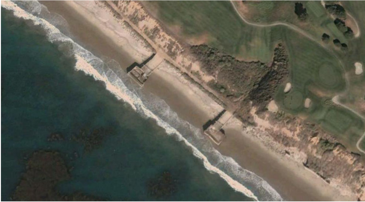
Figure A-5. Shoreline Condition in September 2007
