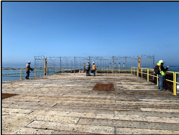
Topside of 421-1 Pier Looking South
