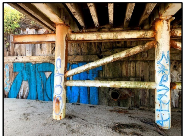
Substructure of 421-2 Pier
