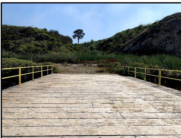
Topside of 421-2 Pier Looking North
