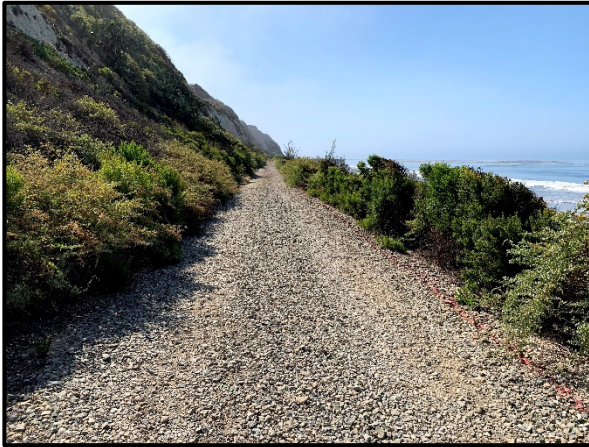
Access Roadway Looking East
