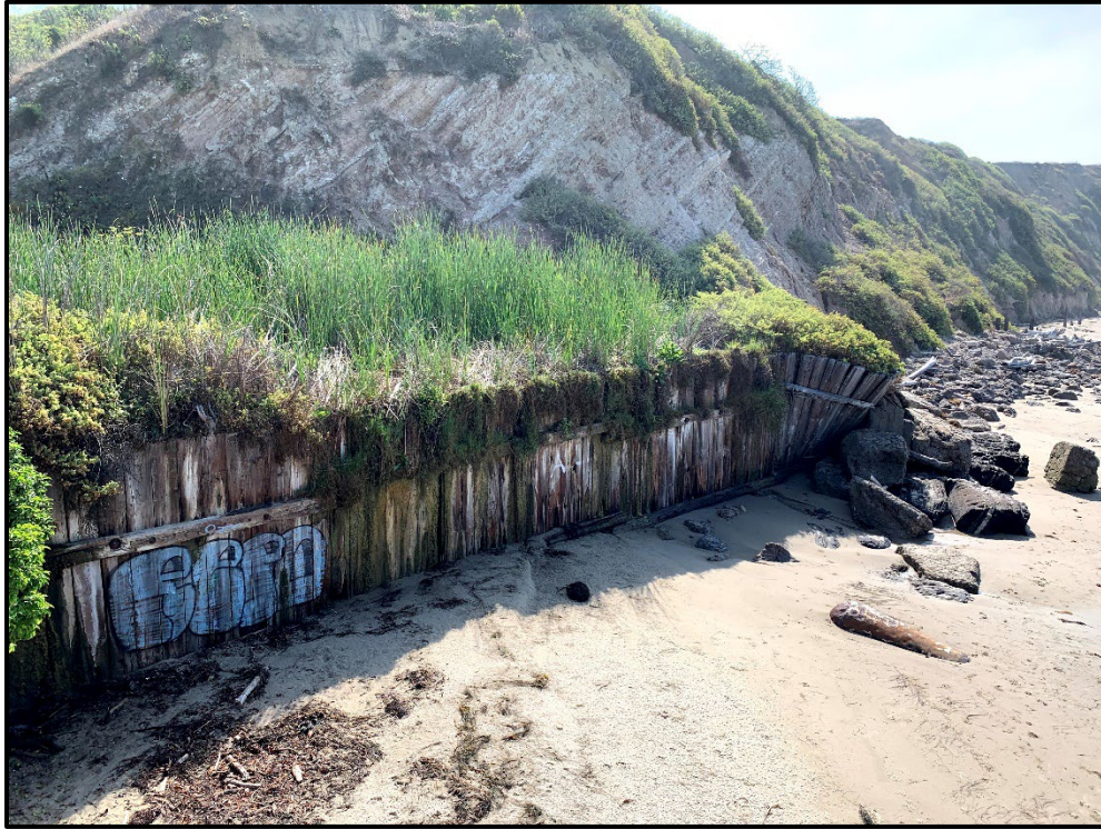
Figure 2-20. End of Wooden Seawall (75 feet east of 421-2 Pier)
