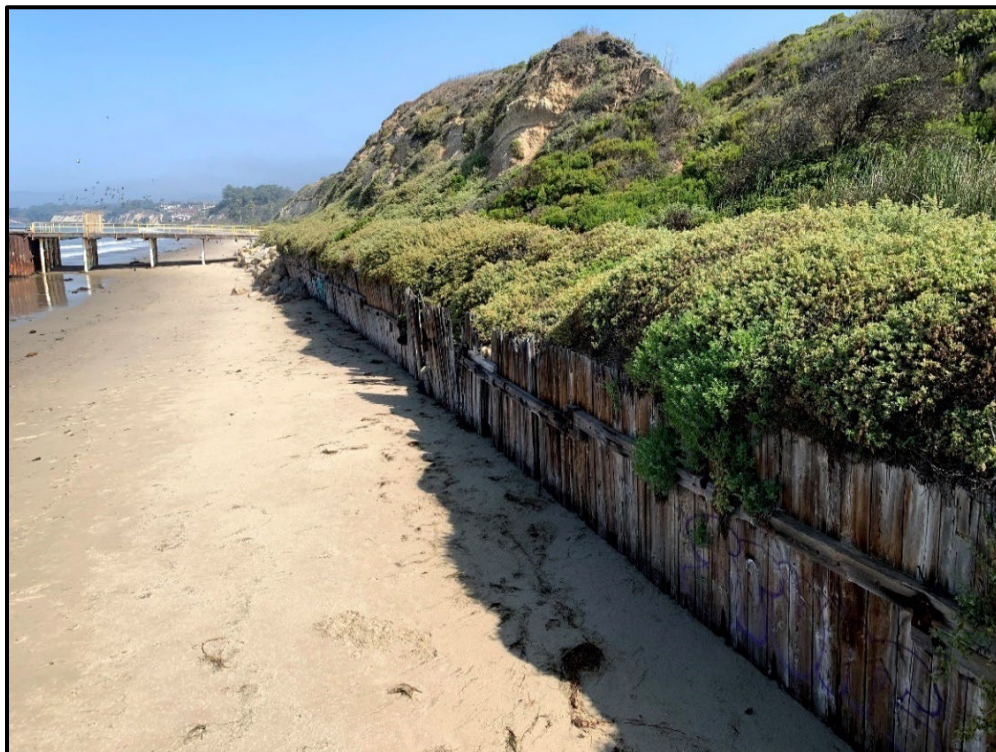
Figure 2-19. Existing Wooden Seawall Between Pier 421-1 and 421-2
