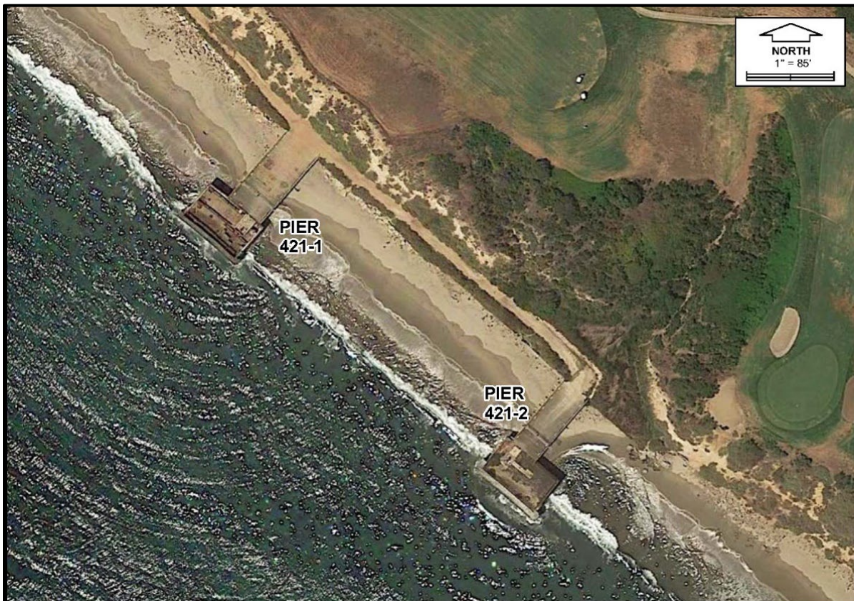
Figure 2-9. PRC 421 Pier Areas
