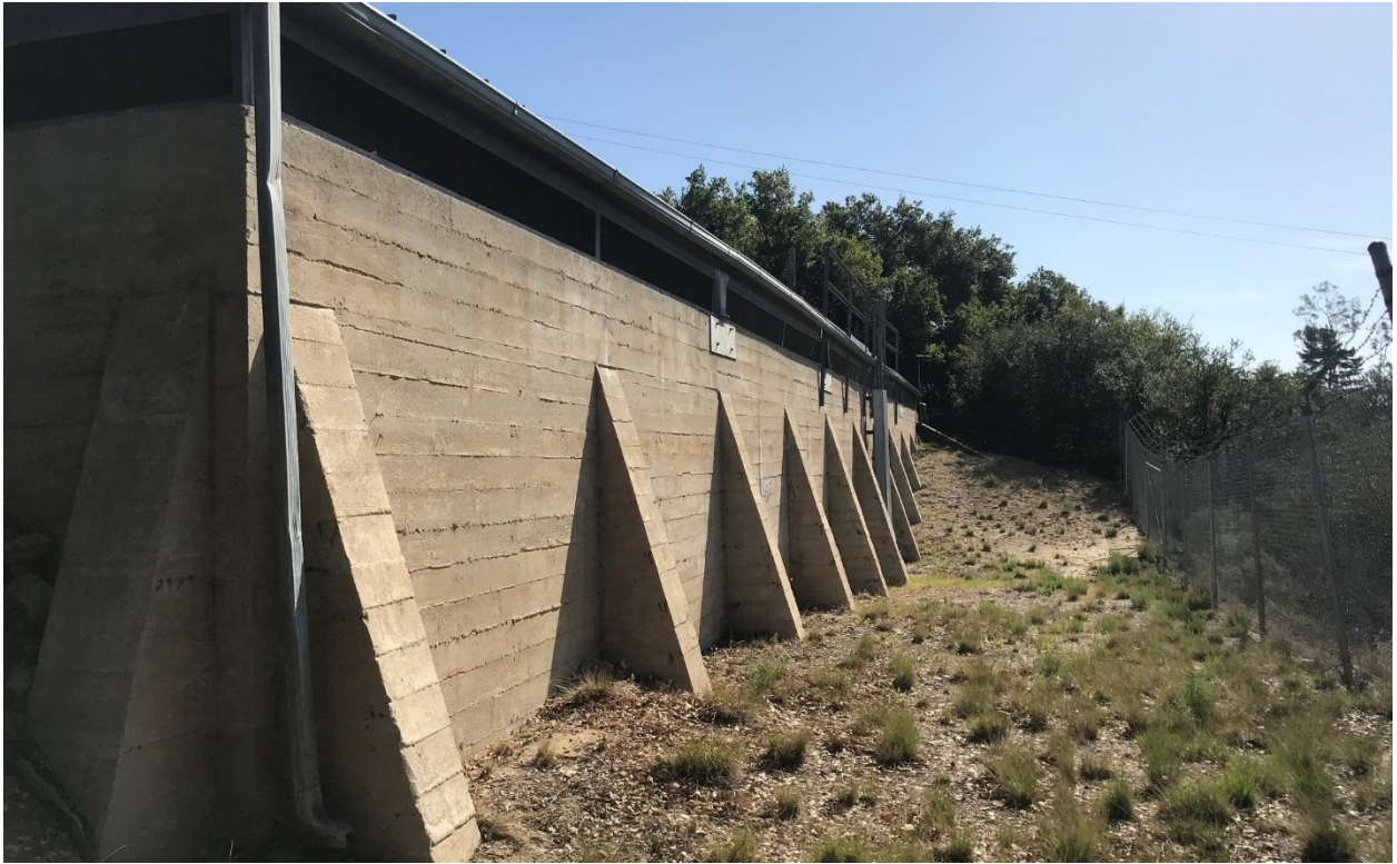
Figure 21 Cold Springs Reservoir, South Elevation, View to the Northeast
