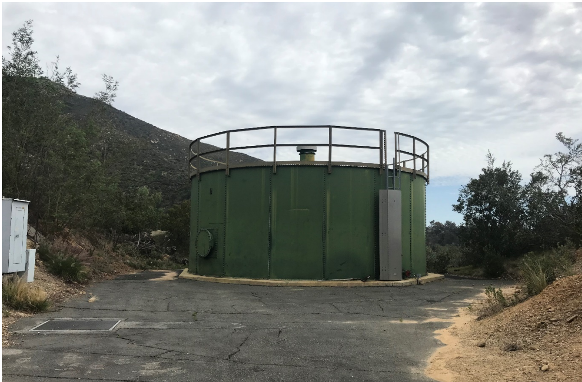
Figure 15 Water Tank, West Elevation, View to East
