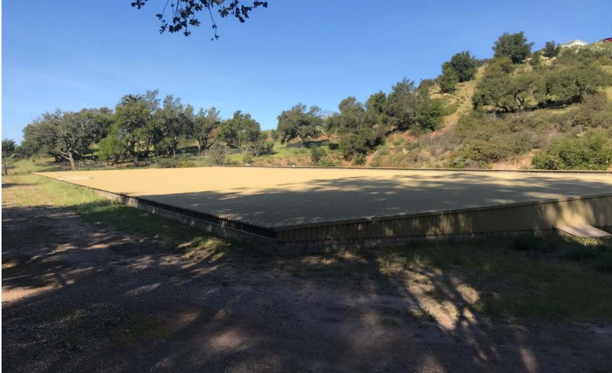
Photograph 1. Terminal Reservoir south and east elevations, view facing west.
