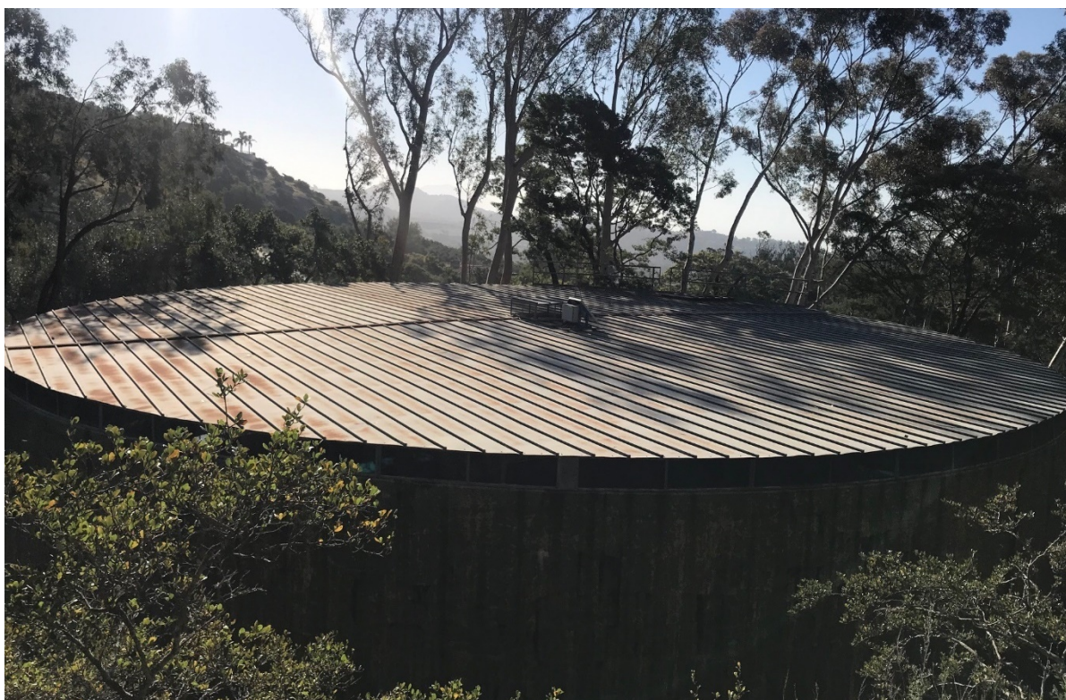
Photograph 2. Roof of Buena Vista Reservoir, view facing east.
