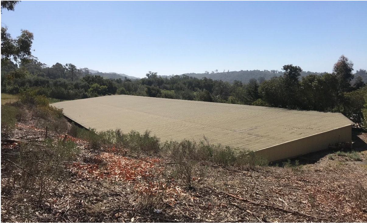
Photograph 1. Romero Reservoir north and west elevations, view facing southeast.
