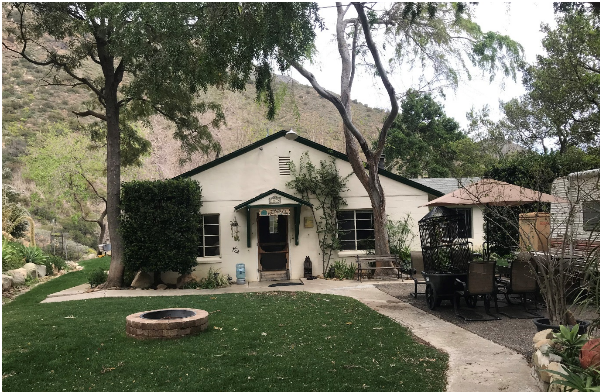
Figure 25 Caretaker's Residence, West Elevation, View to the Northeast
