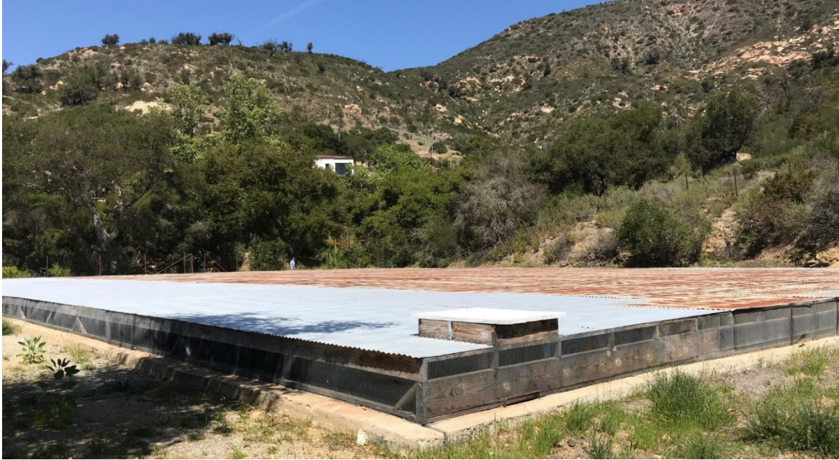
Figure 33 Southeast Corner of Park Lane Reservoir, View to the North
