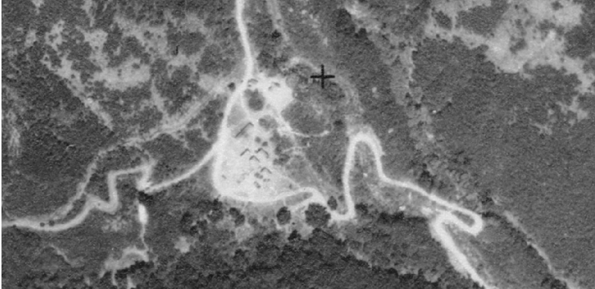
Figure 28 Aerial Photograph of Douulton Reservoir and Treatment Plant Site, 1928
