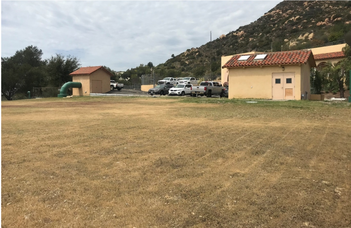
Figure 10 Bella Vista Reservoir Viewed from the Roof, with the Blower (Left) and Pump Station (Right) in Background, View to the Northwest
