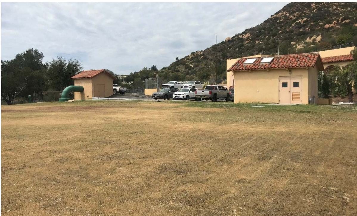
Photograph 1. Bella Vista Reservoir viewed from the roof facing northwest, with the pump station (right) in the background.
