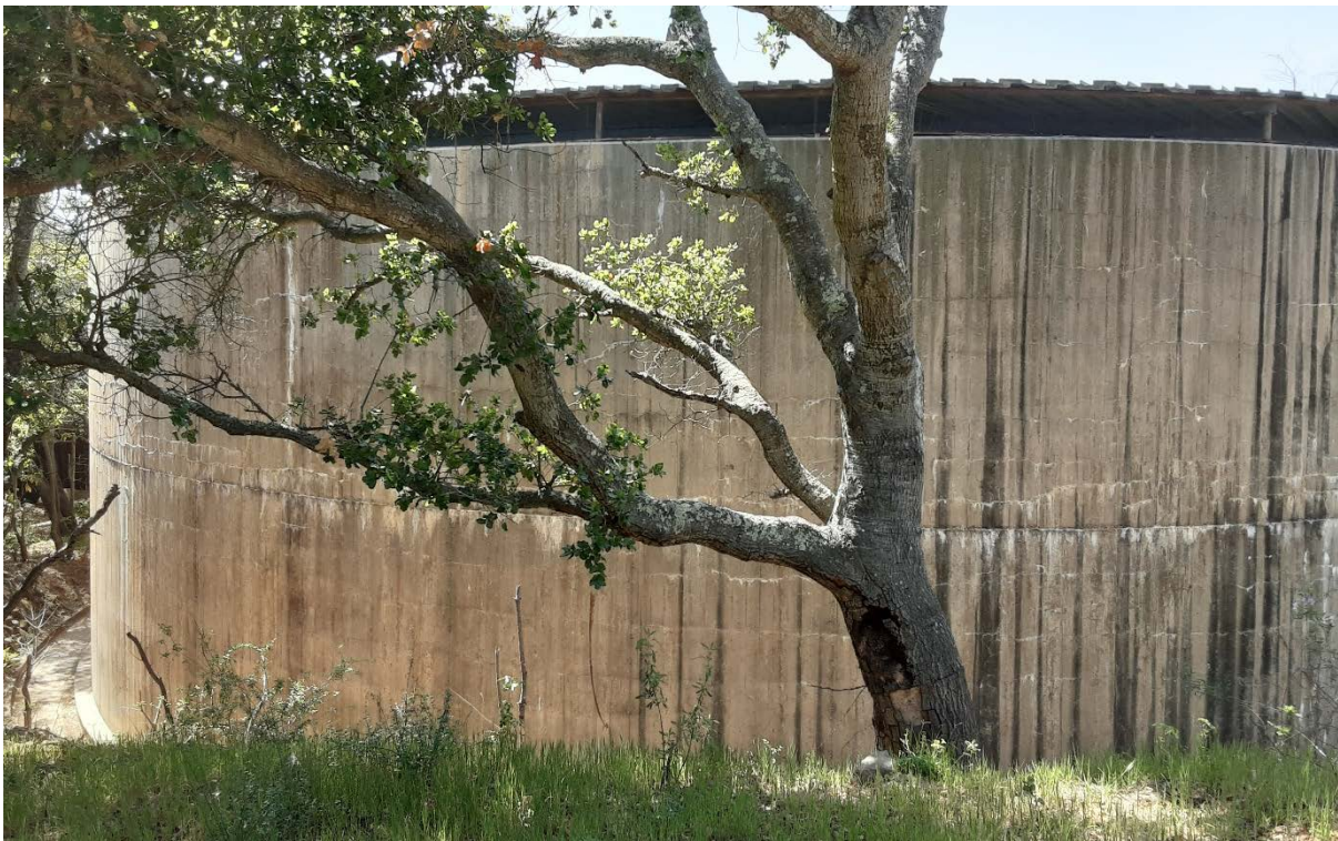
Photograph 2. Hot Springs Reservoir wall, view facing south.
