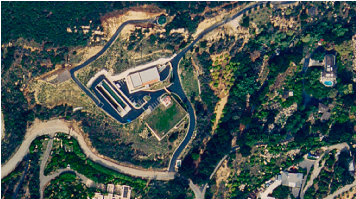
Figure 18 Aerial Photograph of Buena Vista Reservoir and Treatment Plant, 1995
