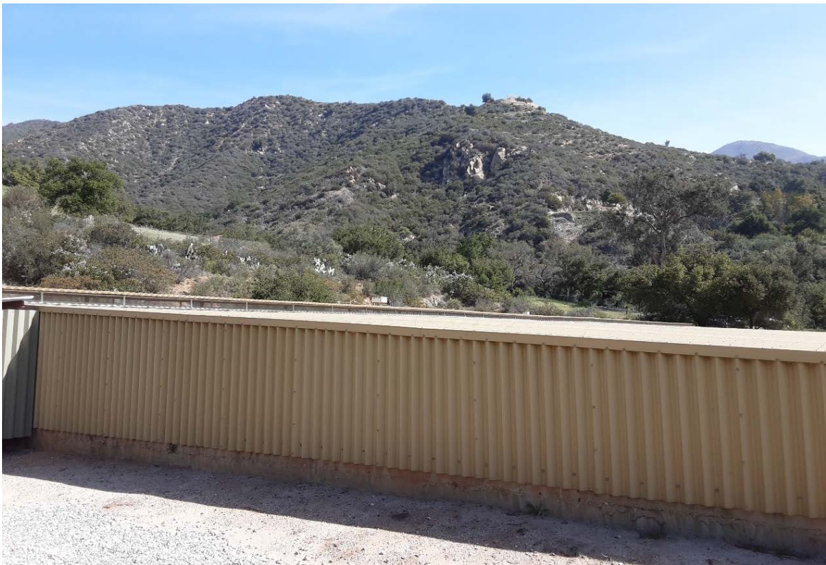
Photograph 2. Terminal Reservoir wall, view facing north.
