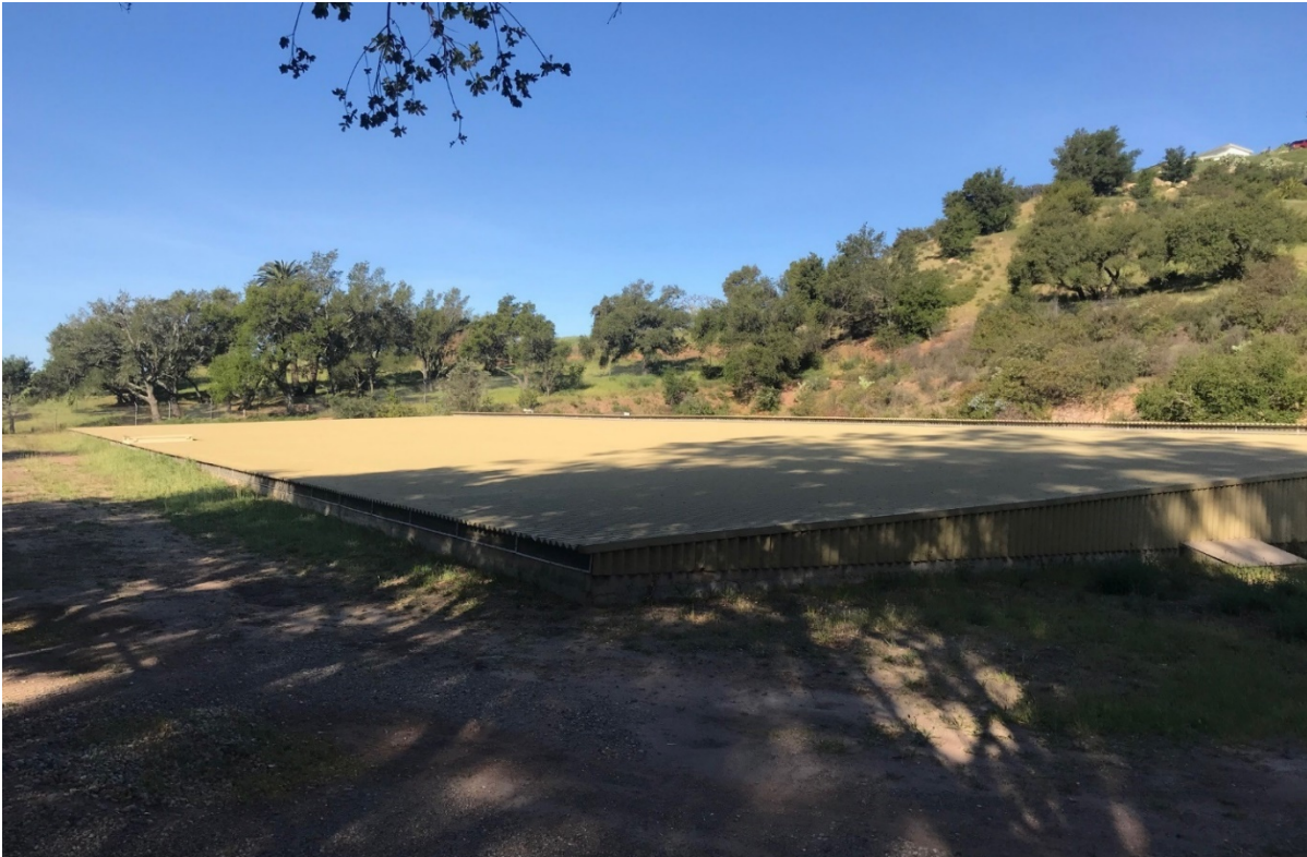
Figure 38 Terminal Reservoir, South and East Elevations, View to the West
