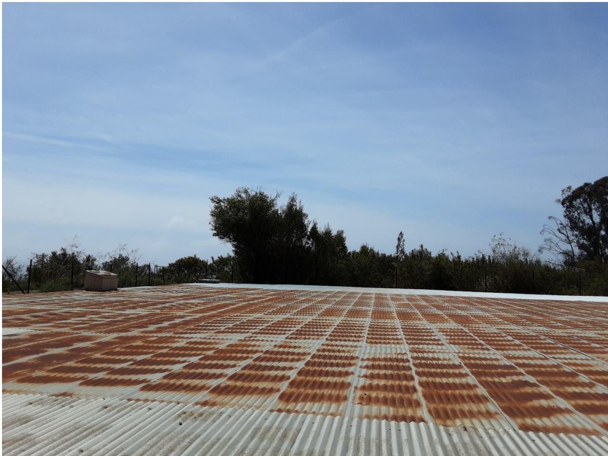
Photograph 2. Roof of Park Land Reservoir, view facing south.
