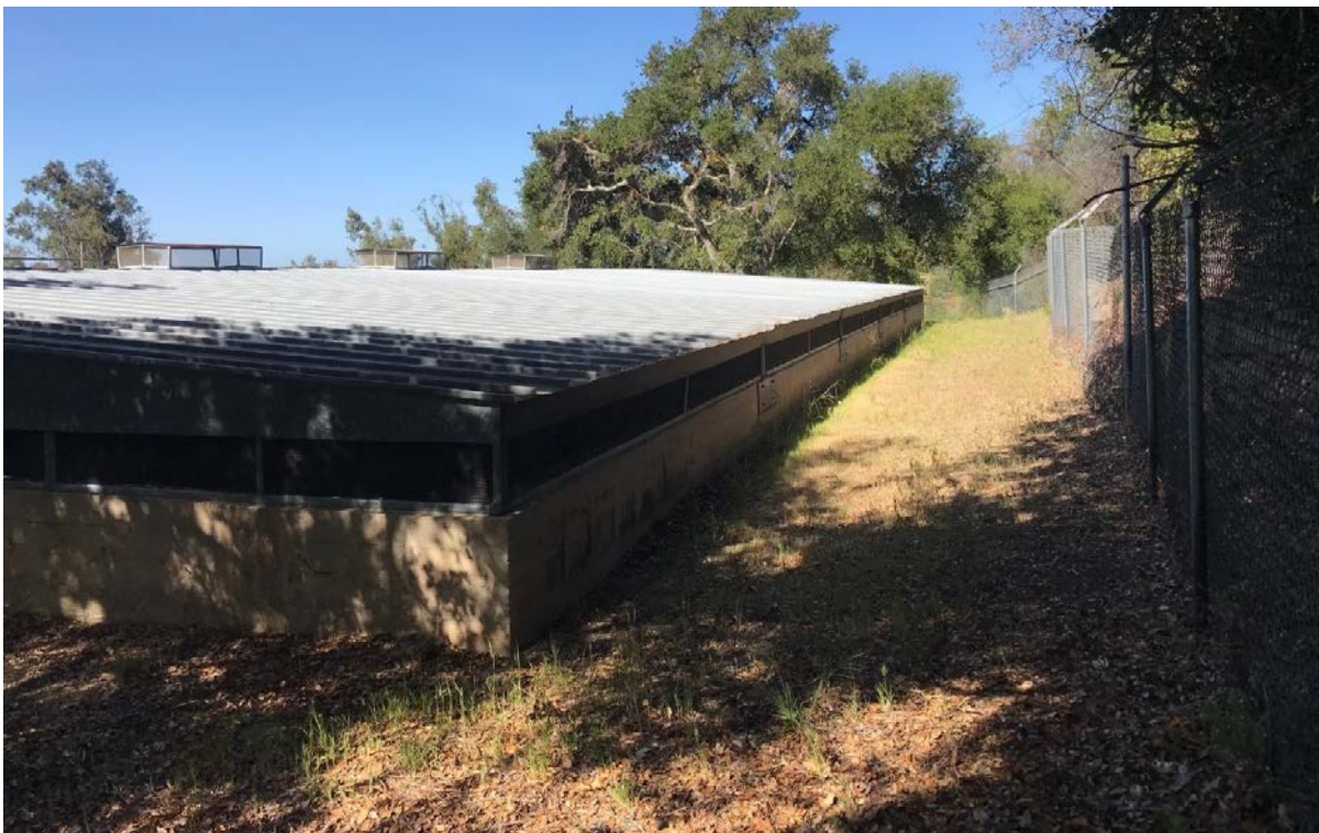
Photograph 2. Cold Springs Reservoir north and east elevations, view facing southwest.
