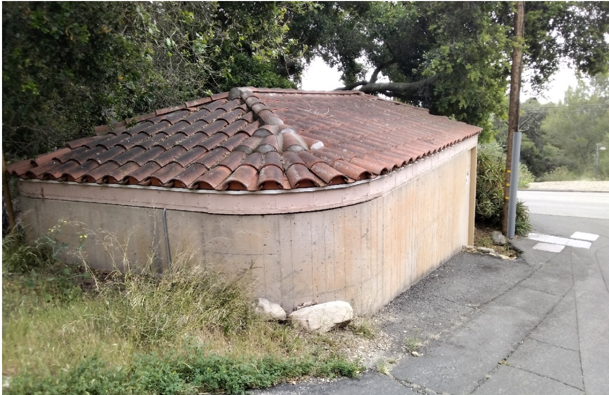
Figure 16 Control Building, North and West Elevations, View to the Southeast
