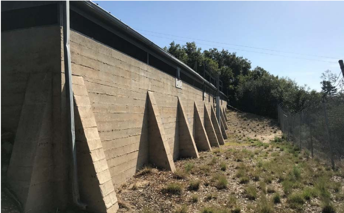
Photograph 1. Cold Springs Reservoir south elevation, view facing northeast.
