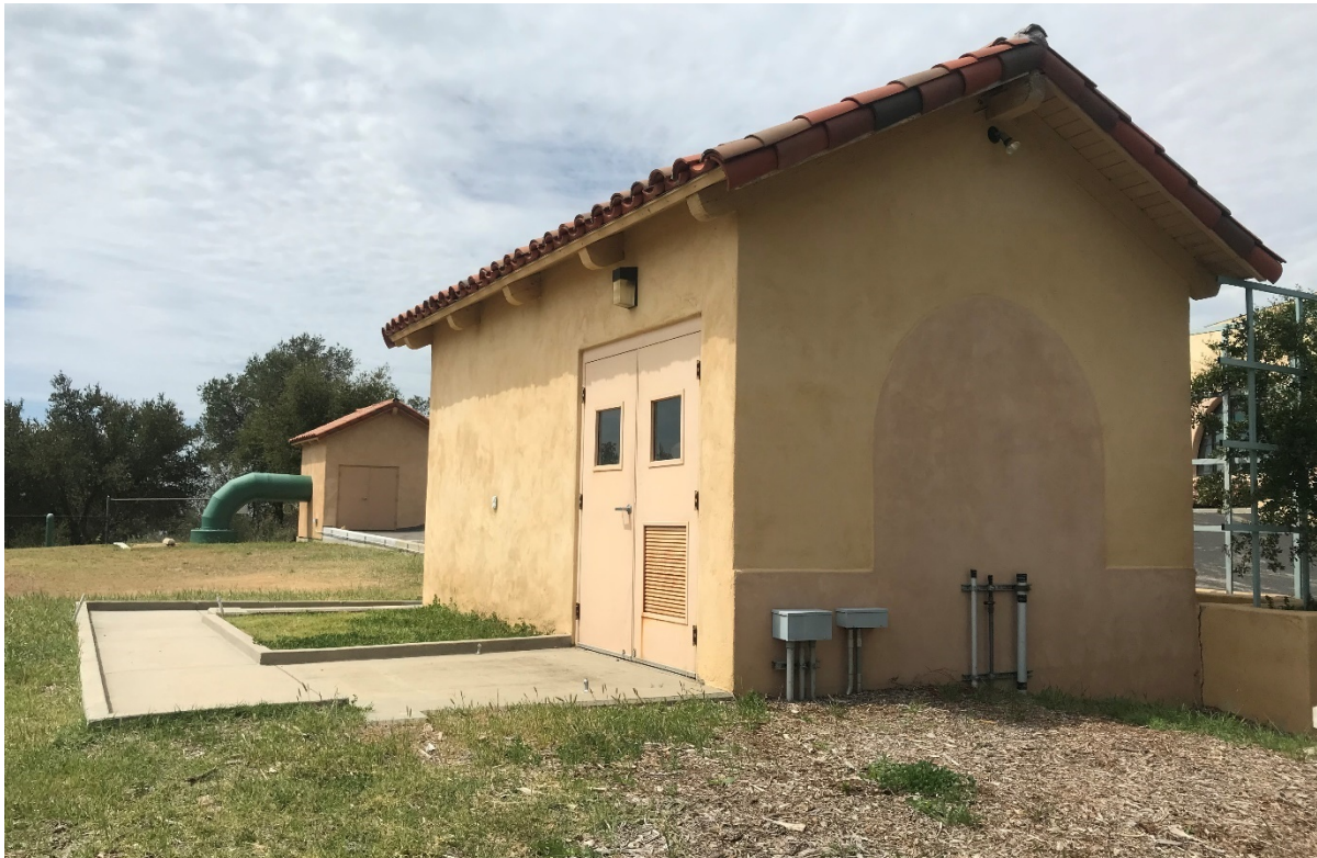
Figure 11 Pump Station, South and East Elevations, View to the Northwest
