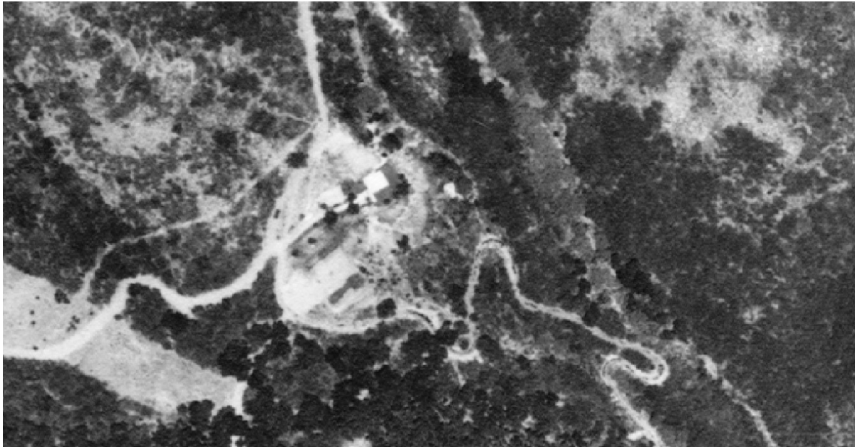
Figure 29 Aerial Photograph of Douulton Reservoir and Treatment Plant Site, 1961
