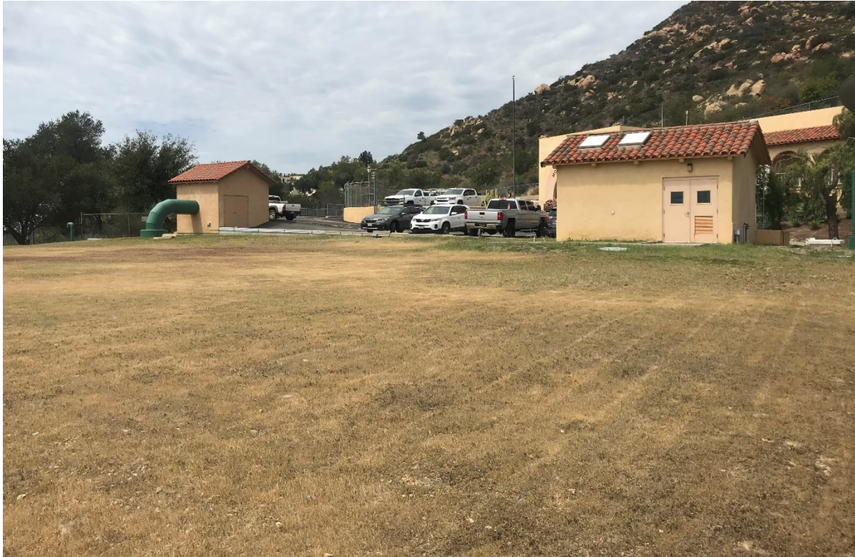
Figure 10 Bella Vista Reservoir Viewed from the Roof, with the Blower (Left) and Pump Station (Right) in Background, View to the Northwest
