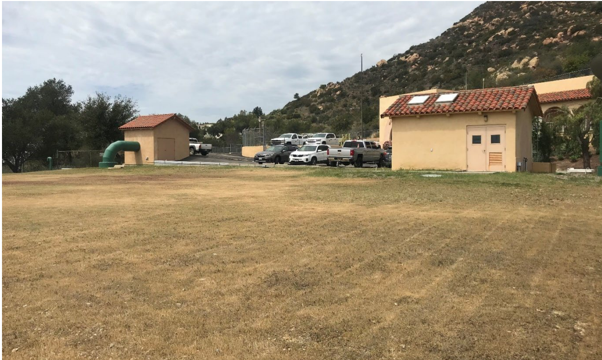
Photograph 1. Bella Vista Reservoir viewed from the roof facing northwest, with the pump station (right) in the background.
