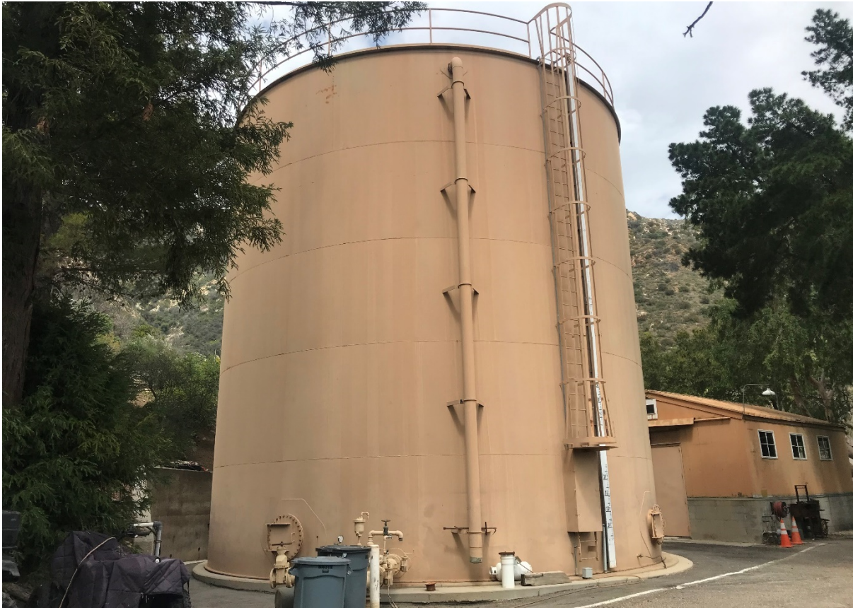
Photograph 1. Southwest side of Doulton Reservoir, view facing northeast.
