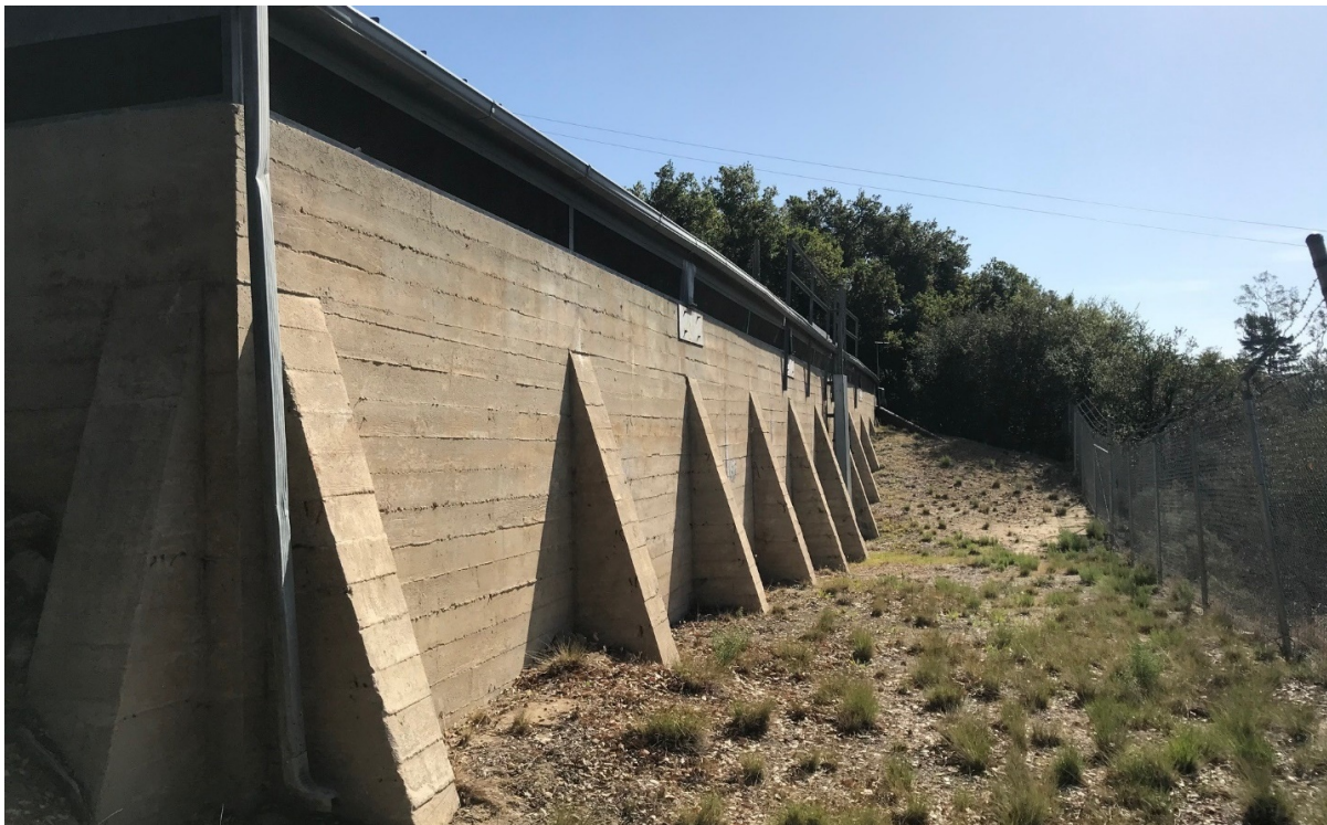
Photograph 1. Cold Springs Reservoir south elevation, view facing northeast.
