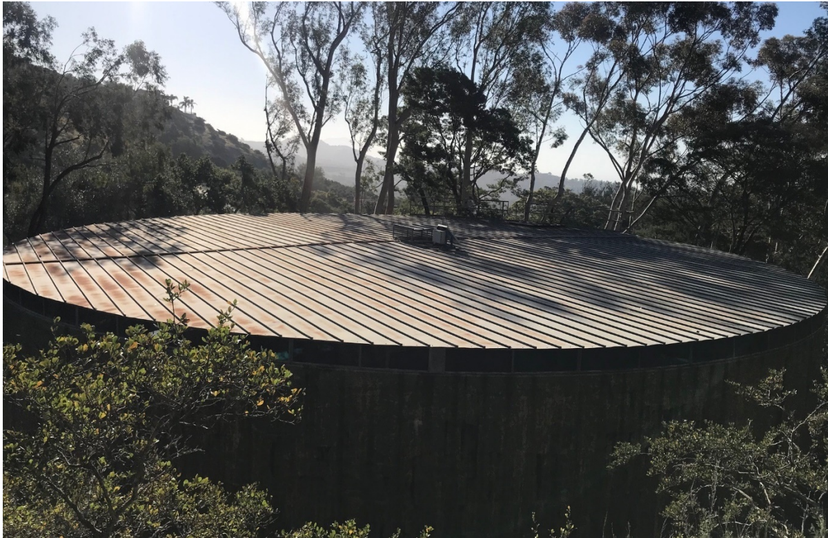
Figure 20 Roof of Buena Vista Reservoir, View to the East
