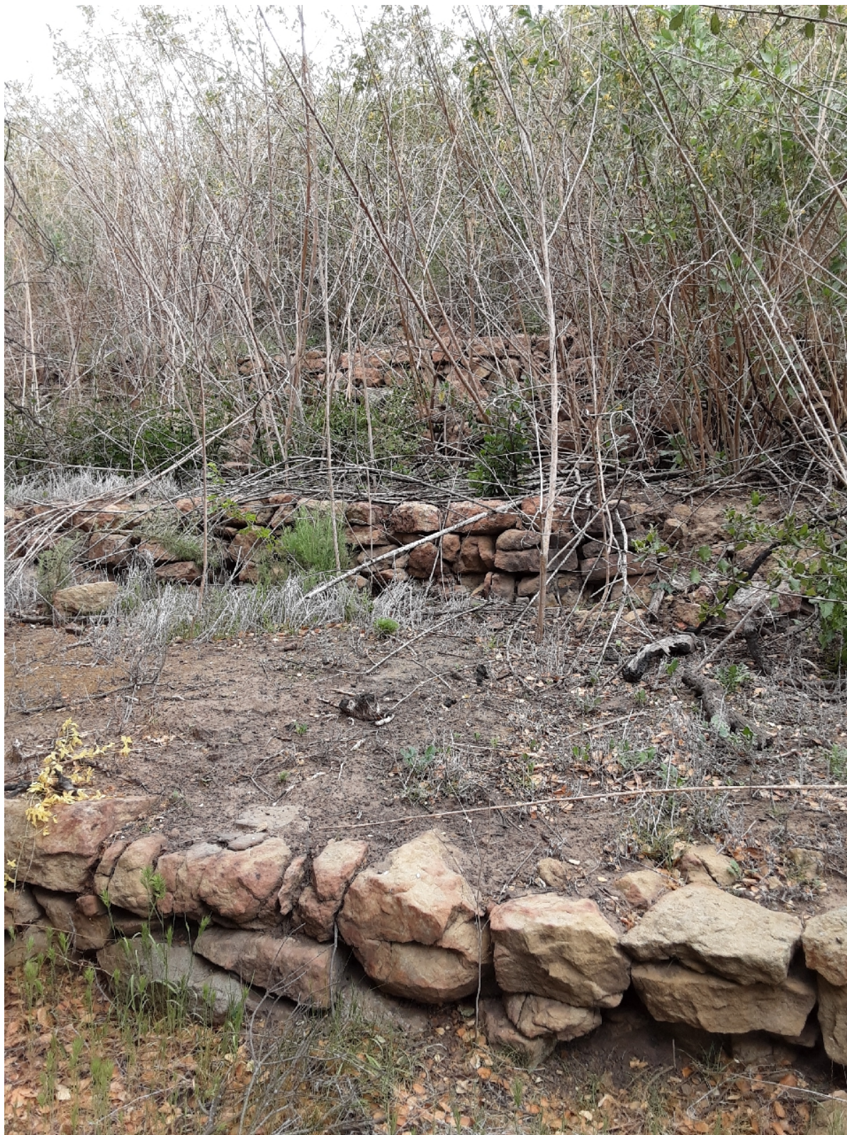
Figure 34 Retaining Wall, Southwest Elevation, View to the North
