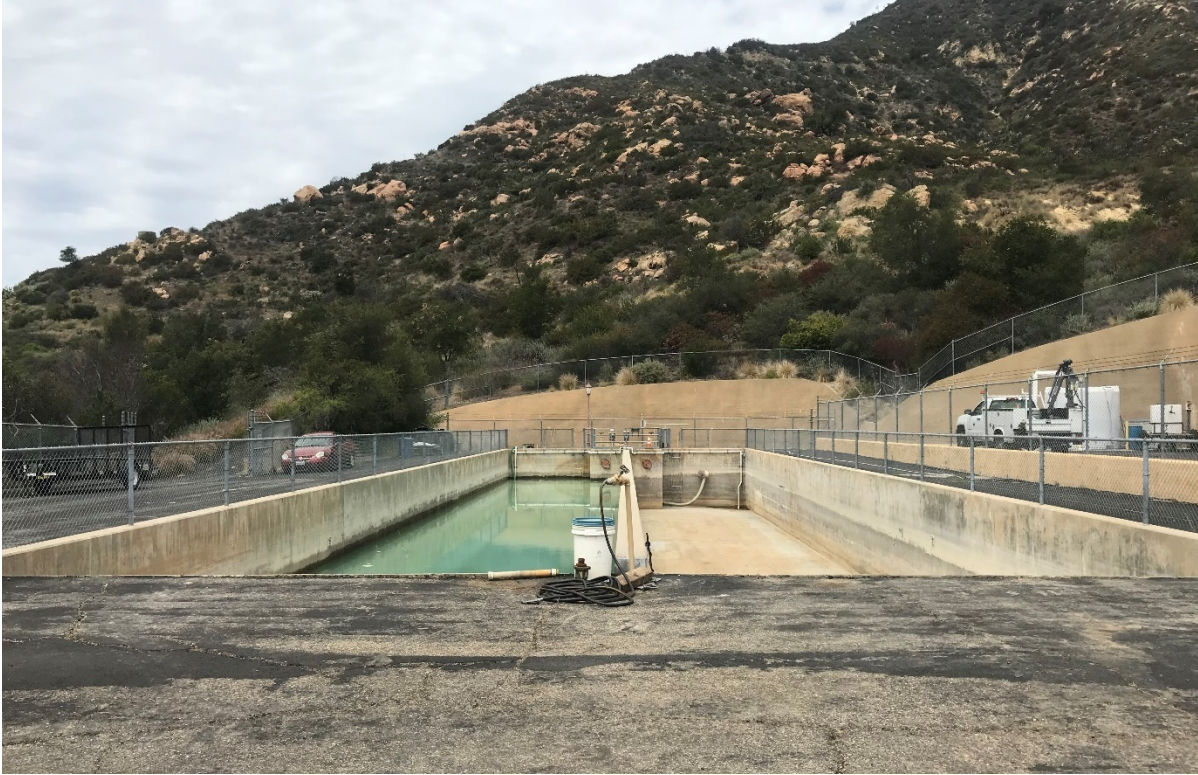
Figure 14 Settling Basins, View to the Northwest
