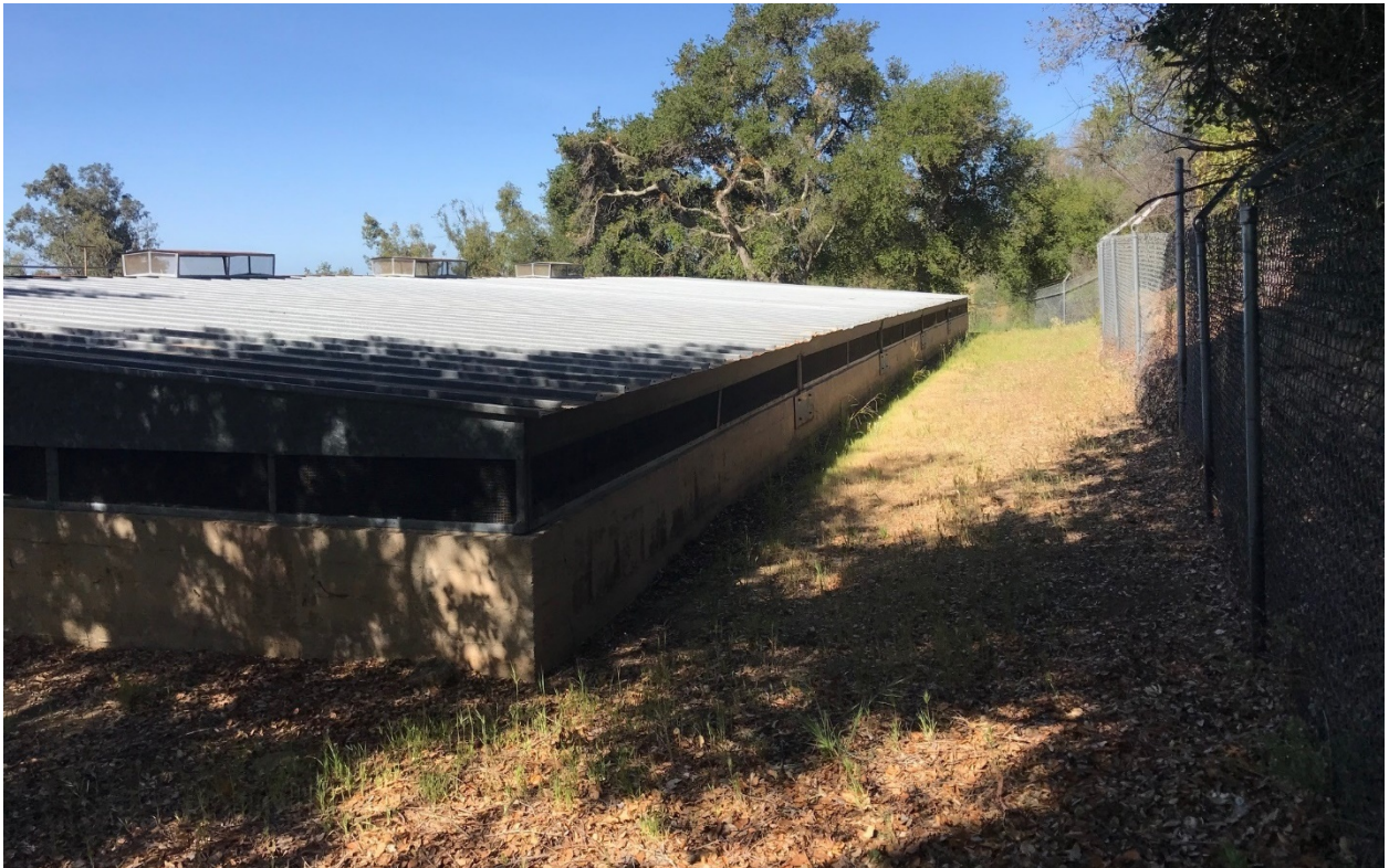
Figure 22 Cold Springs Reservoir, North and East Elevations, View to the Southwest
