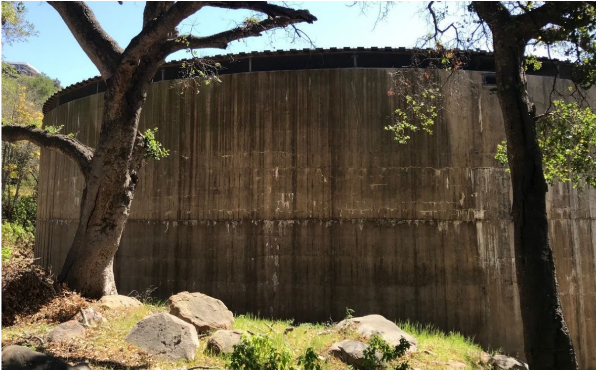
Photograph 1. Hot Springs Reservoir west elevation, view facing east.
