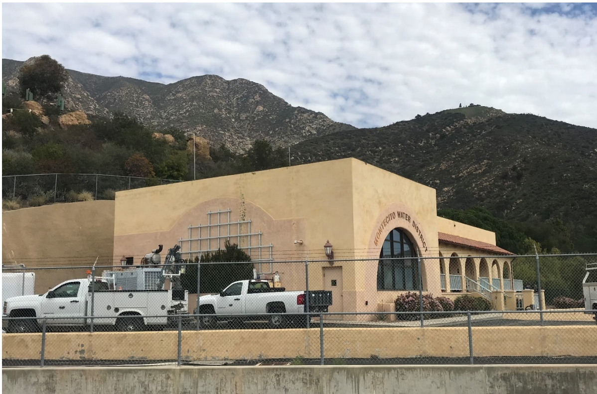
Figure 13 Treatment Plant Building, South and West Elevations, View to the Northeast
