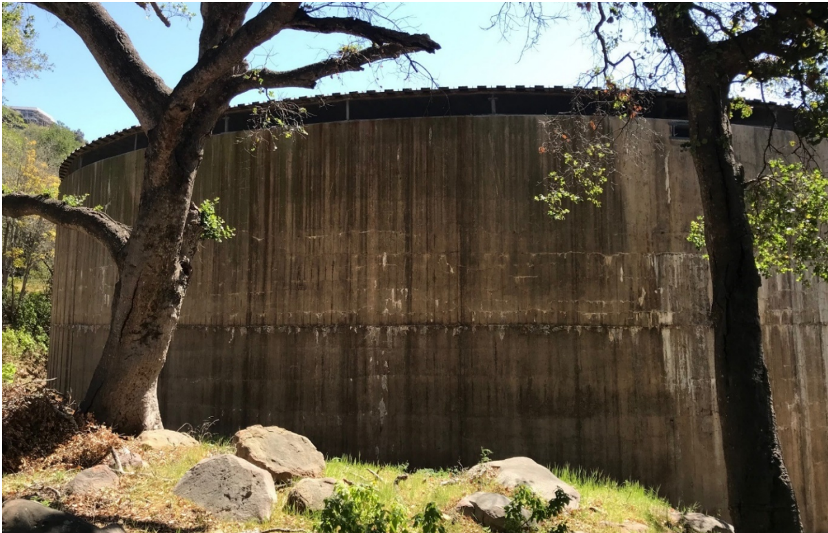
Figure 31 Hot Springs Reservoir, West Elevation, View to the East
