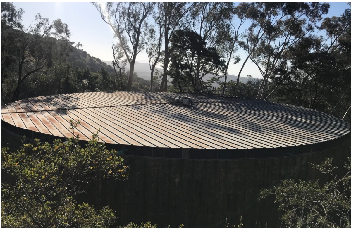
Photograph 2. Roof of Buena Vista Reservoir, view facing east.
