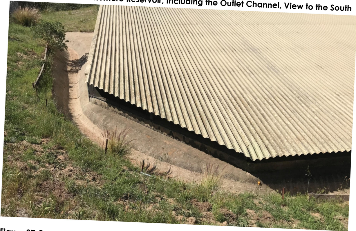
Figure 37 Pump Station, South and West Elevations, View to the Northeast
