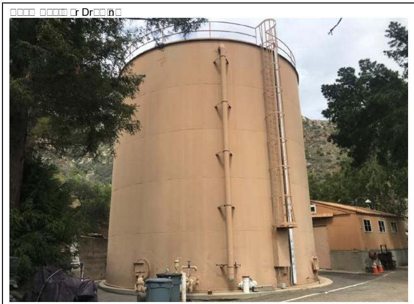
Doulton Reservoir with treatment plant to the right, view to the northeast
