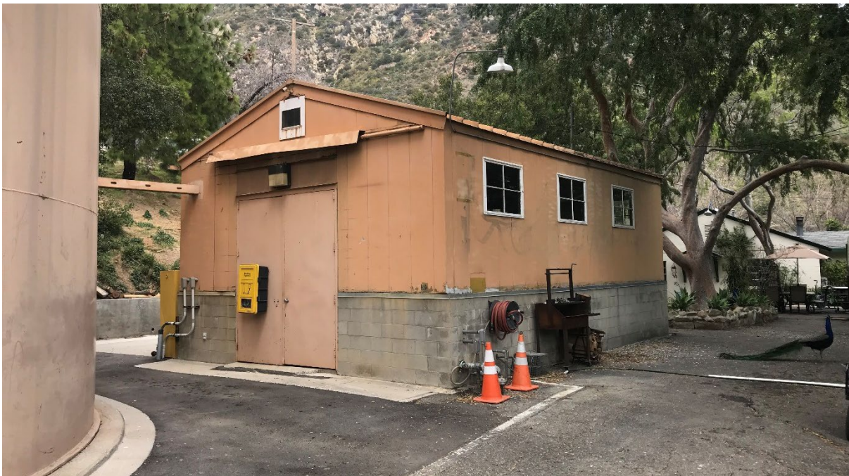
Photograph 2. Treatment Plant south and west elevations, view facing north.
