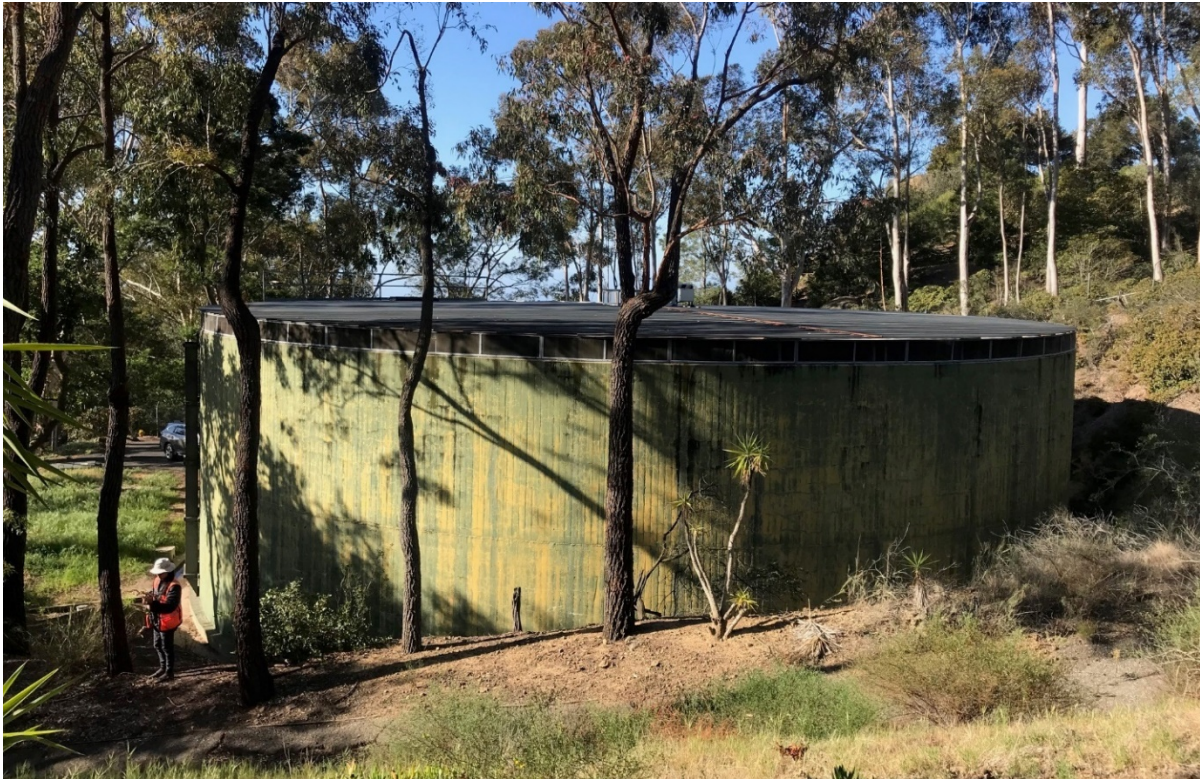
Photograph 1. North elevation of Buena Vista Reservoir, view facing south.
