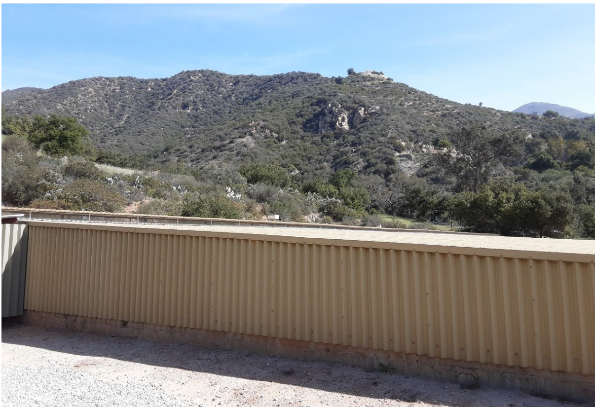
Photograph 2. Terminal Reservoir wall, view facing north.
