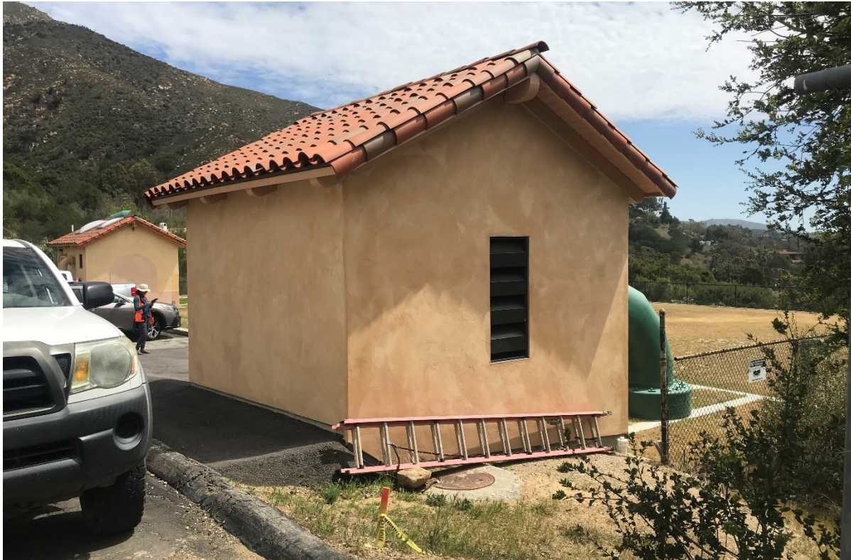
Figure 12 Blower, North and West Elevations, View to the Southeast
