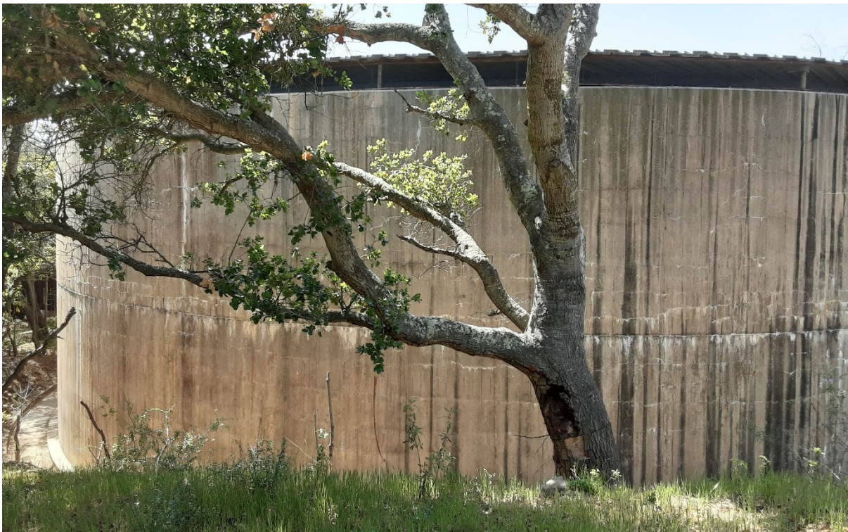
Photograph 2. Hot Springs Reservoir wall, view facing south.
