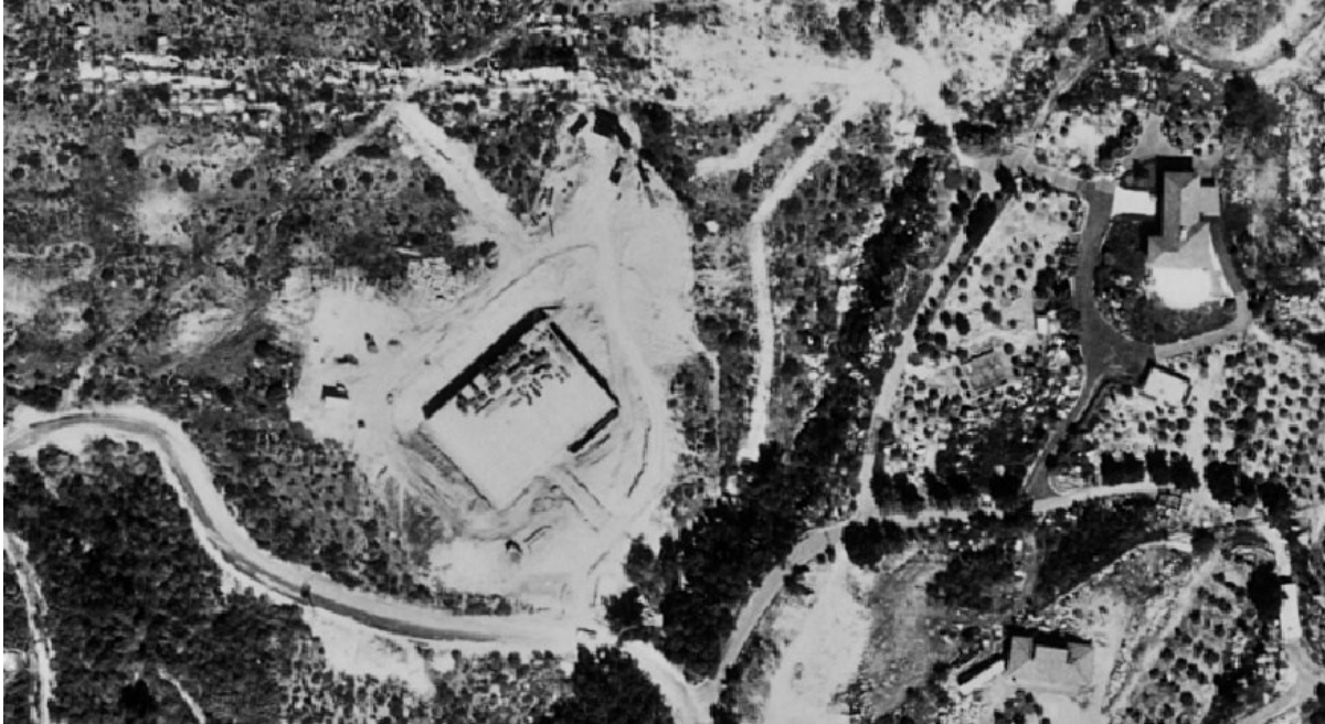
Figure 17 Aerial Photograph of Bella Vista Reservoir Under Construction, 1975
