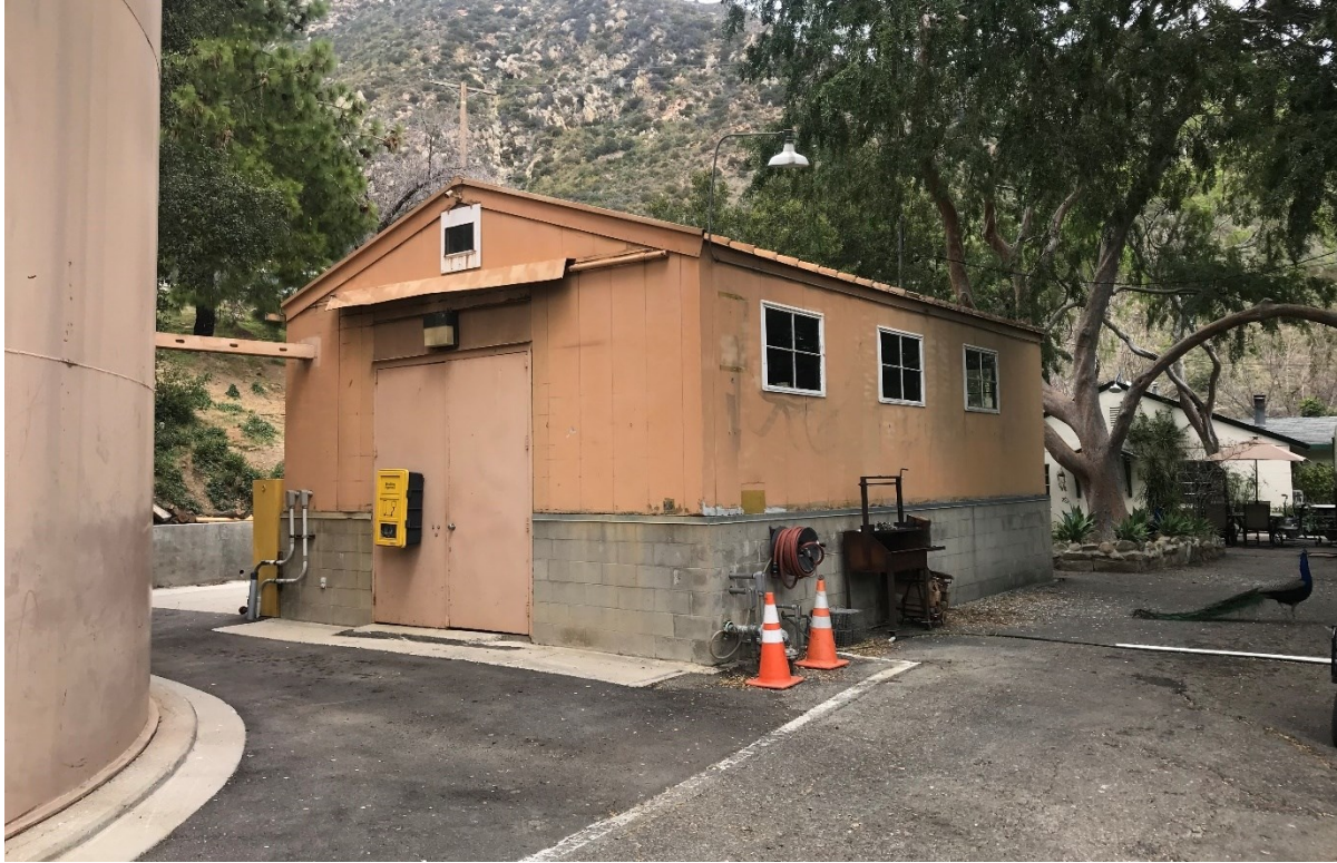
Figure 24 Treatment Plant, South and West Elevations, View to the North
