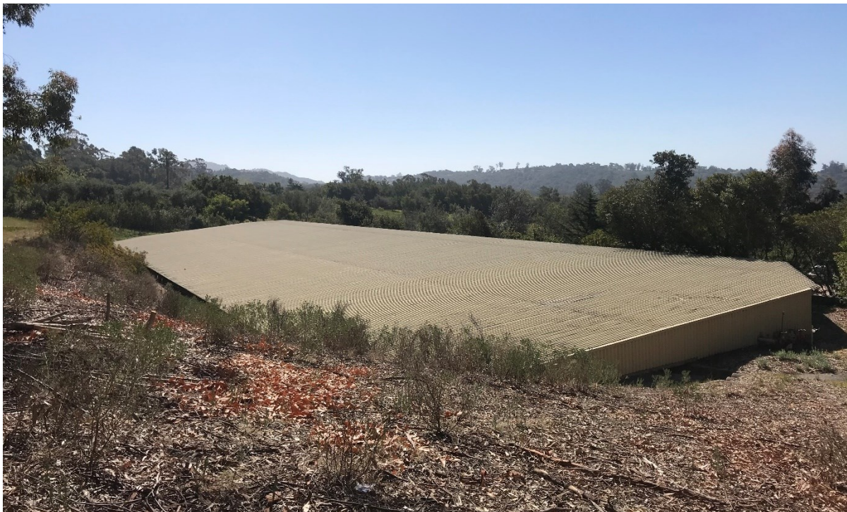
Figure 35 Romero Reservoir, North and West Elevations, View to the Southeast
