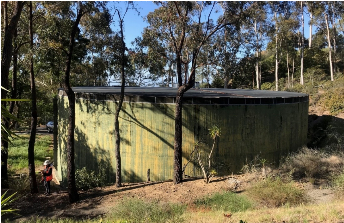
Figure 19 Buena Vista Reservoir, North Elevation, View to the South
