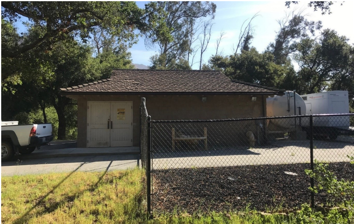
Figure 39 Pump Station Building, West Elevation, View to the Northeast
