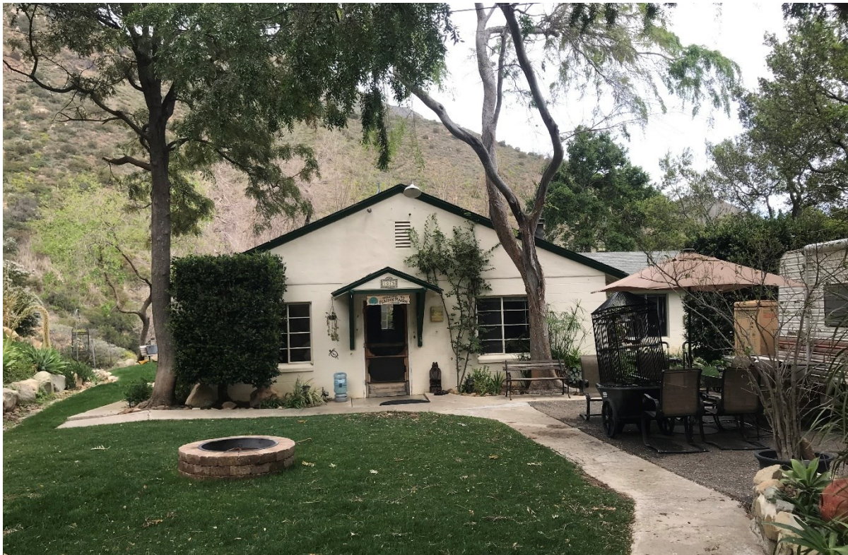
Figure 25 Caretaker's Residence, West Elevation, View to the Northeast
