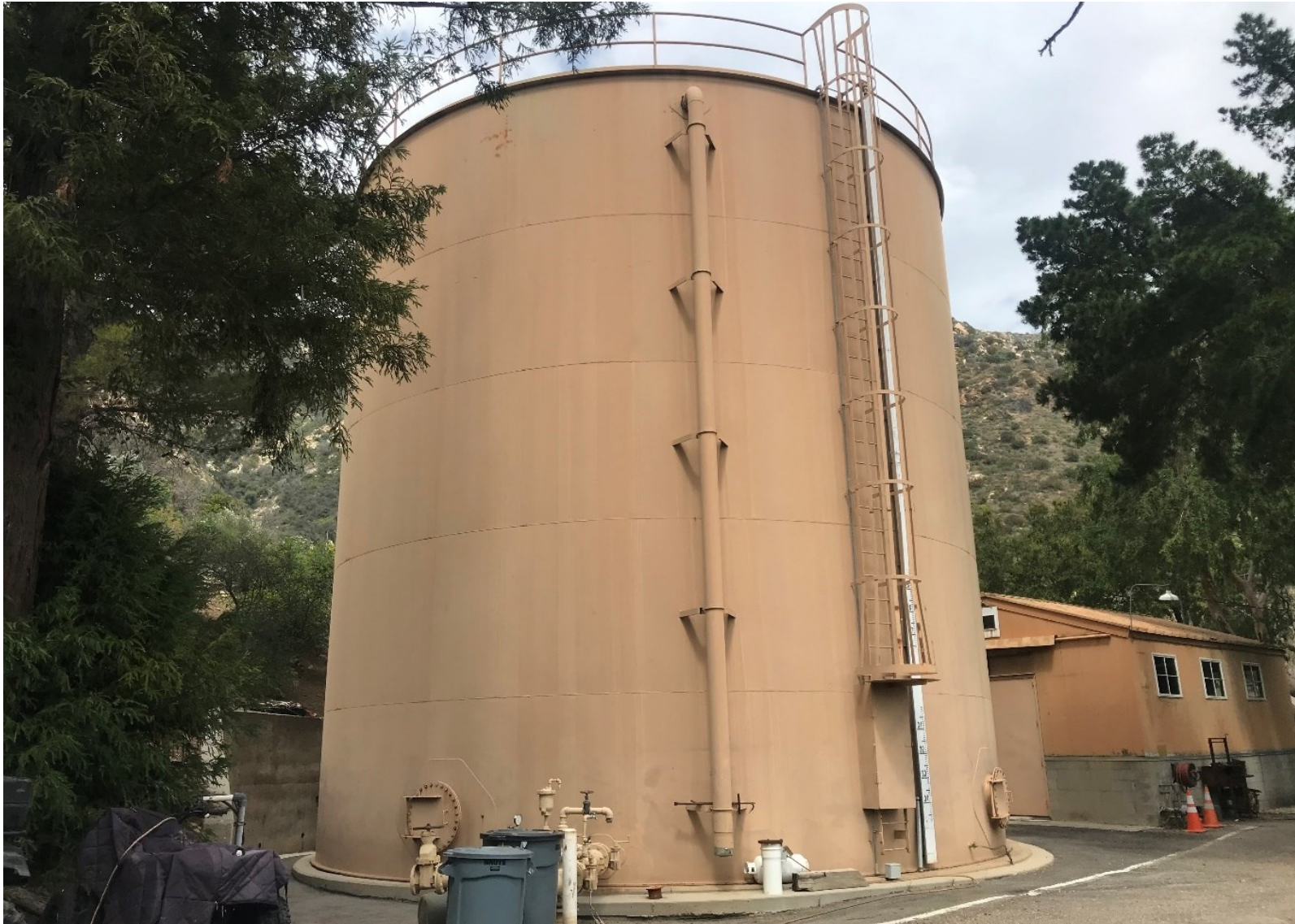
Figure 23 Doultan Reservoir, Southwest Side, View to the Northeast
