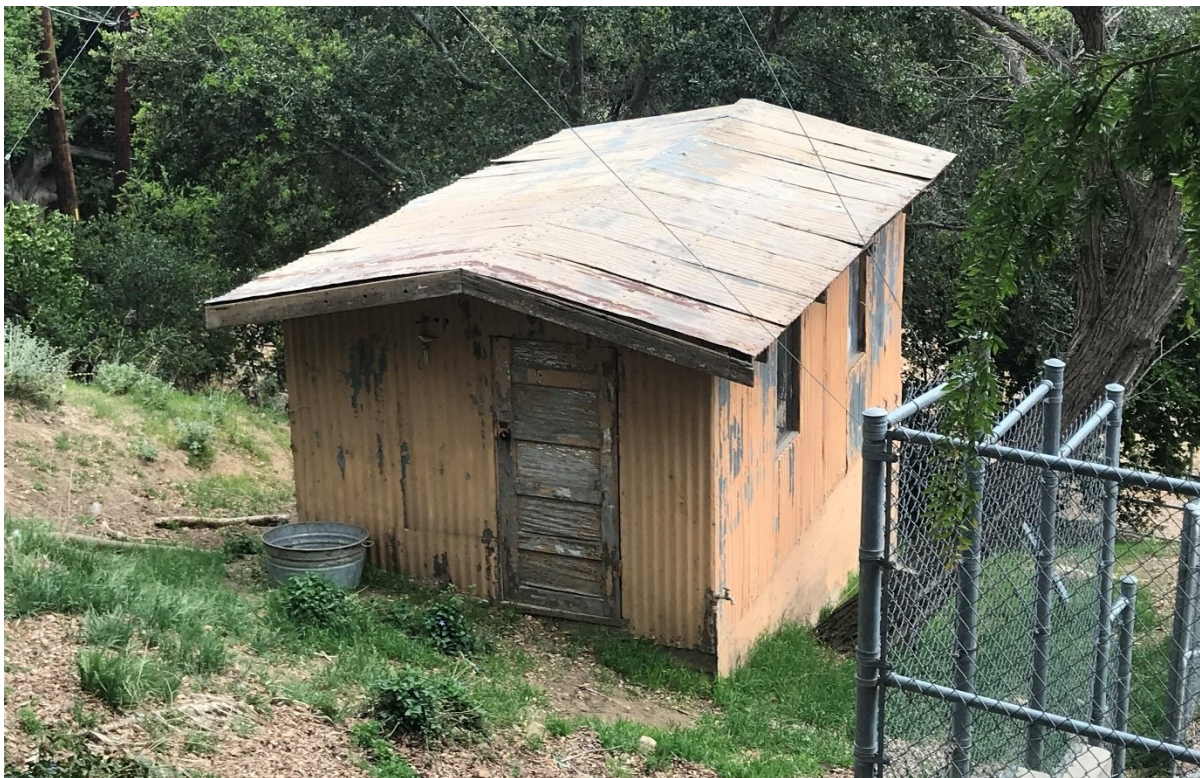
Figure 27 Ancillary Building, North and West Elevations, View to the East
