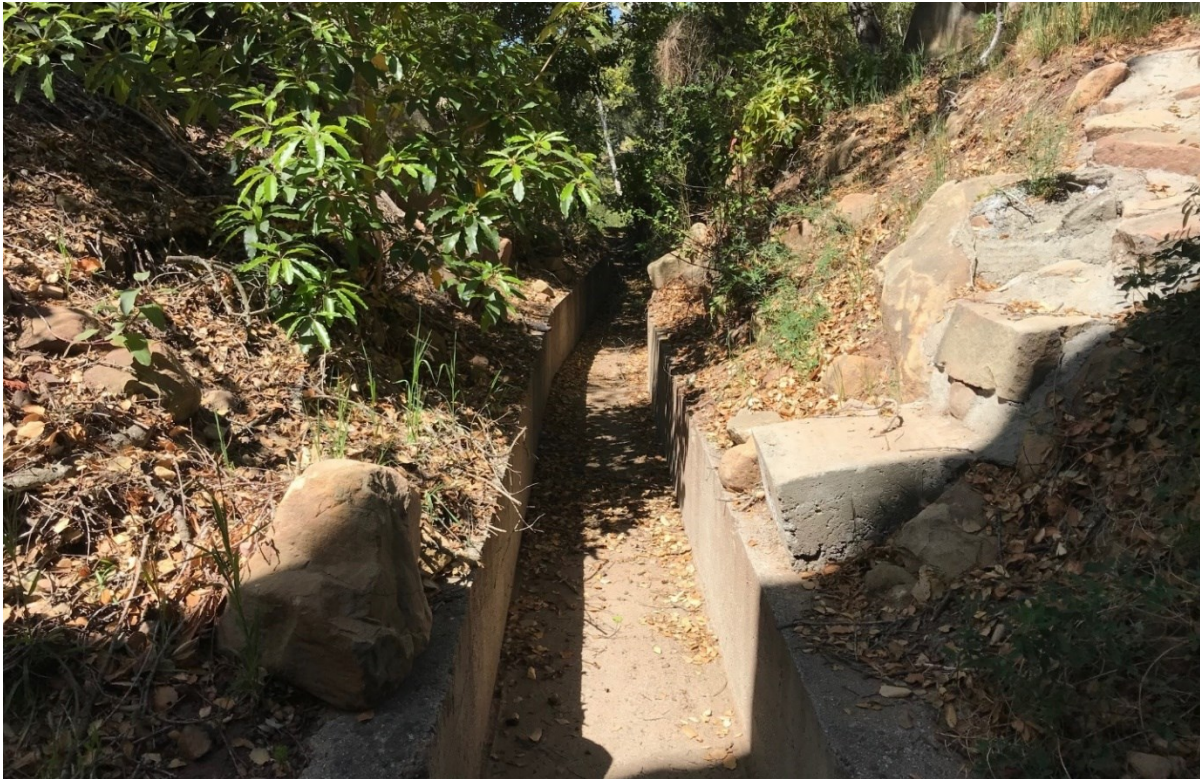
Figure 32 Outlet Ditch, North and East Elevation, View to the Southwest
