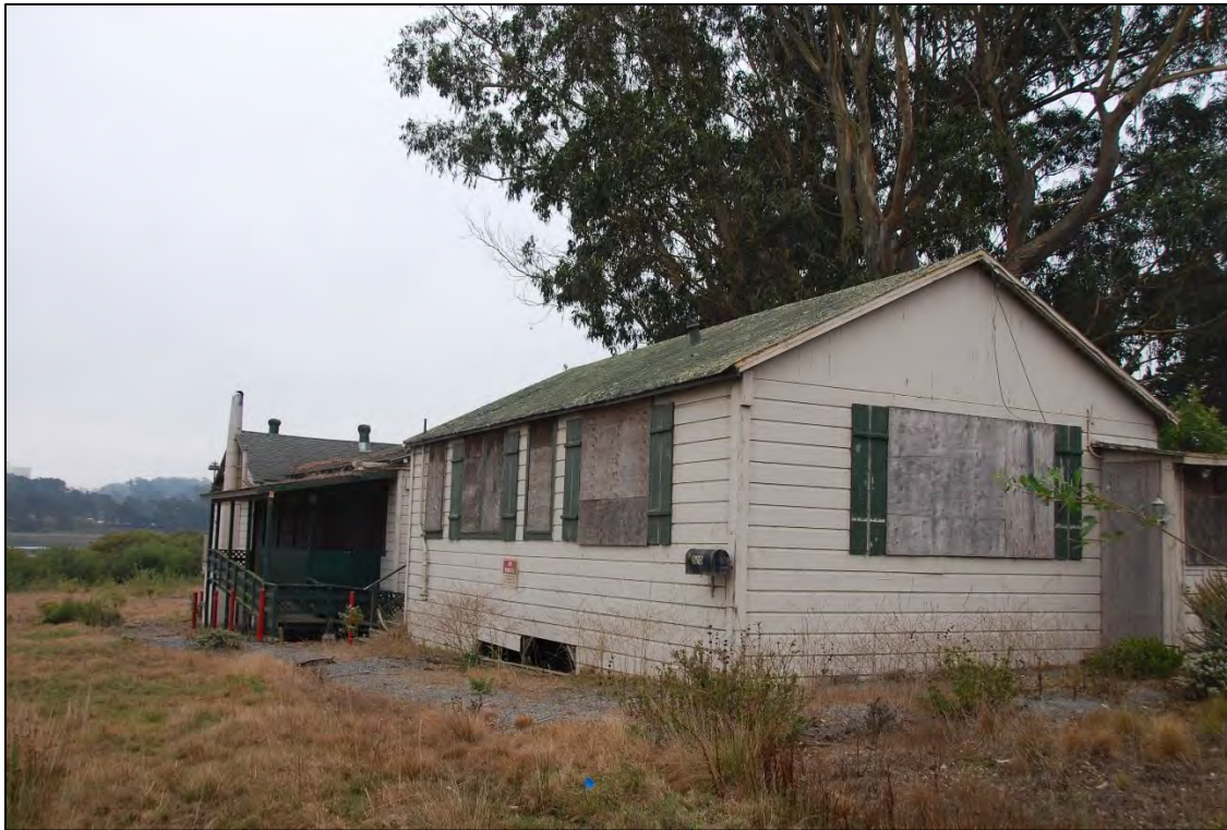
Figure 6: Caretaker's House (view southeast of west and north elevations). Note the Clubhouse is also visible in this photo.
