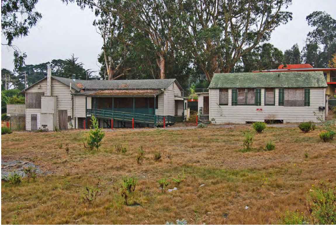
Photo 25. Clubhouse (contributing building) on left and Caretaker's House (contributing building) on right; facing south; 15 October 2019.
