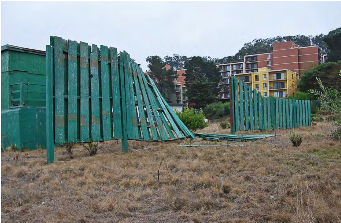
Photo 14. Safety fence (contributing feature) between Skeet Fields 5 and 6; facing southeast; 15 October 2019.
