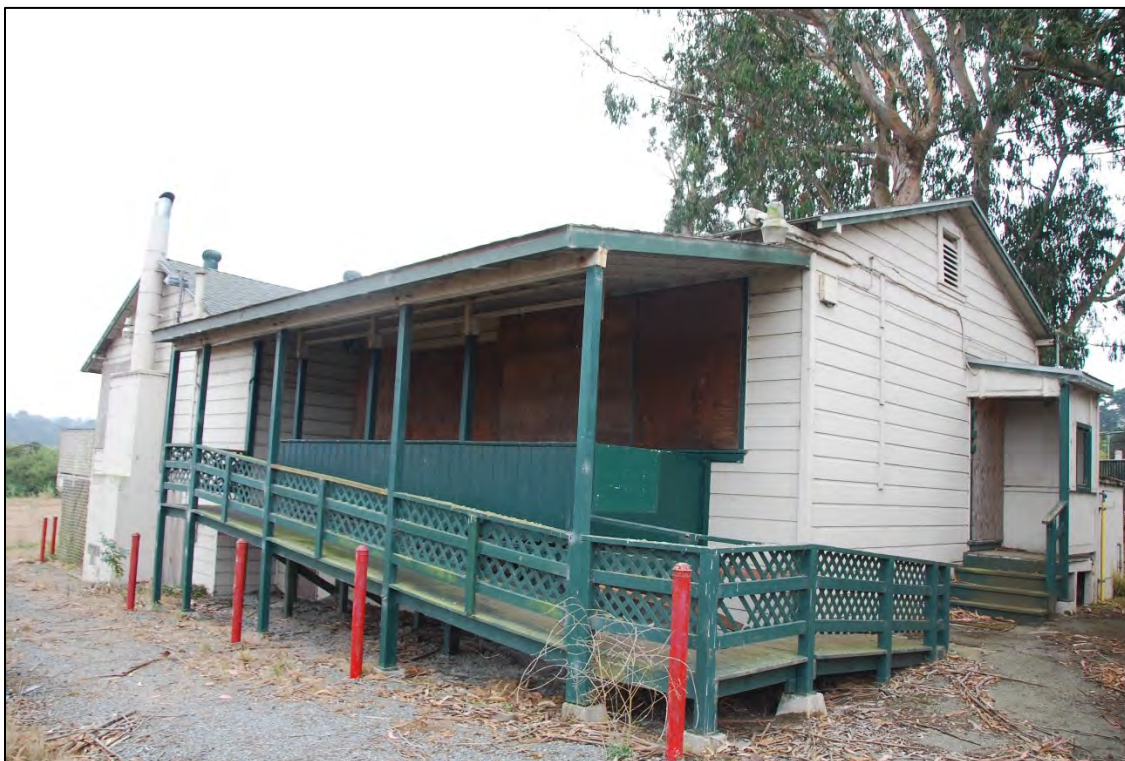
Figure 7: Clubhouse, a contributing feature (view southeast of north and west elevations).
