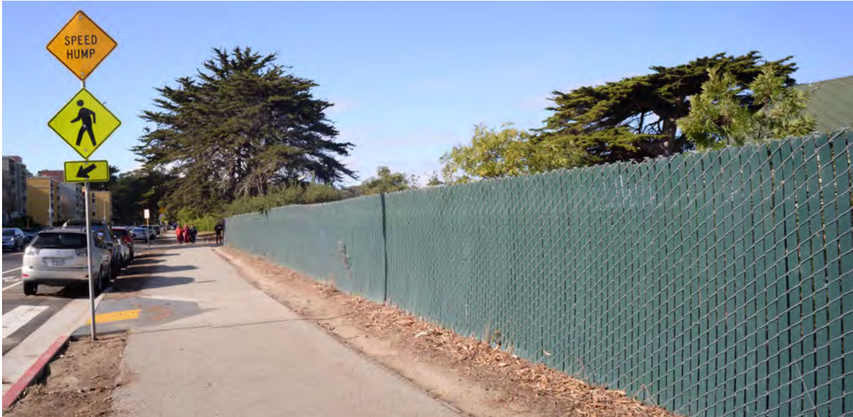
Photo 3 – Existing Fencing Looking Northwest
