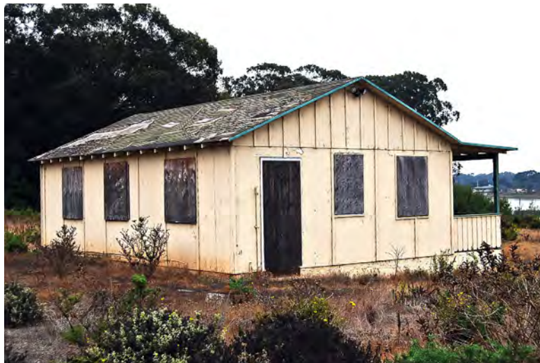
Photo 7. Trap House; facing northwest; (non-contributing feature)
