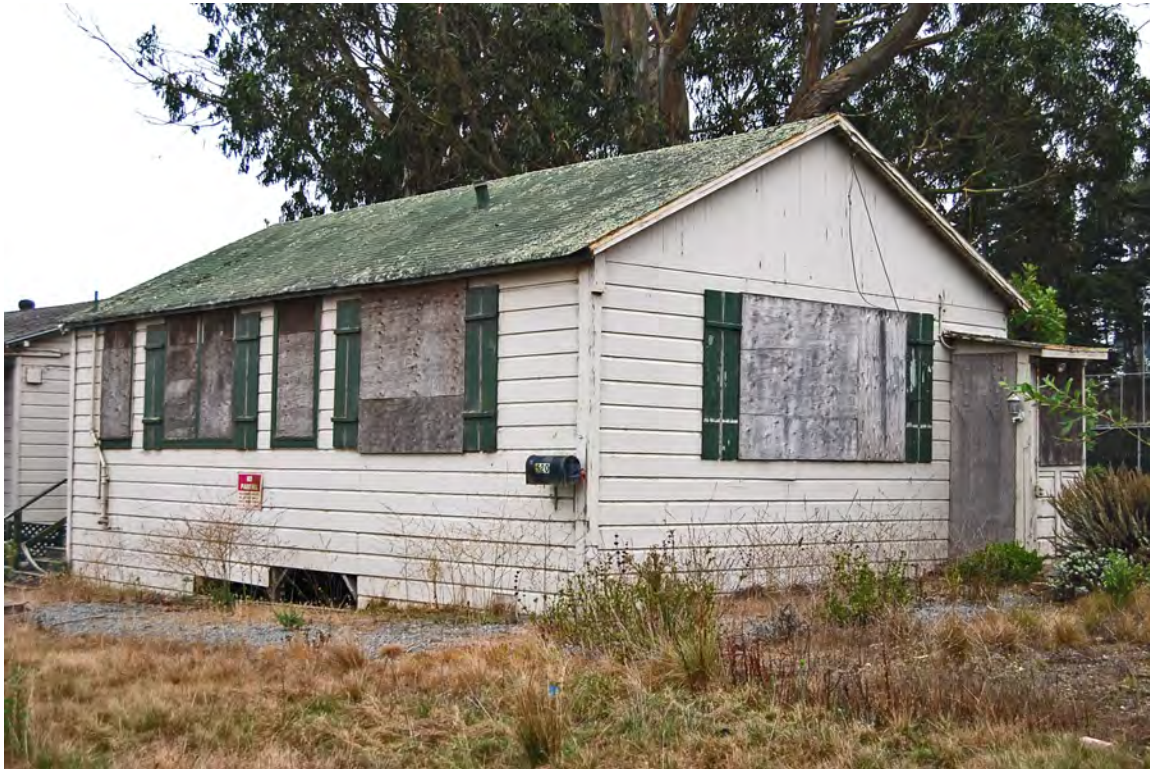
Photo 26. Caretaker's House (contributing building); facing southeast; 15 October 2019.
