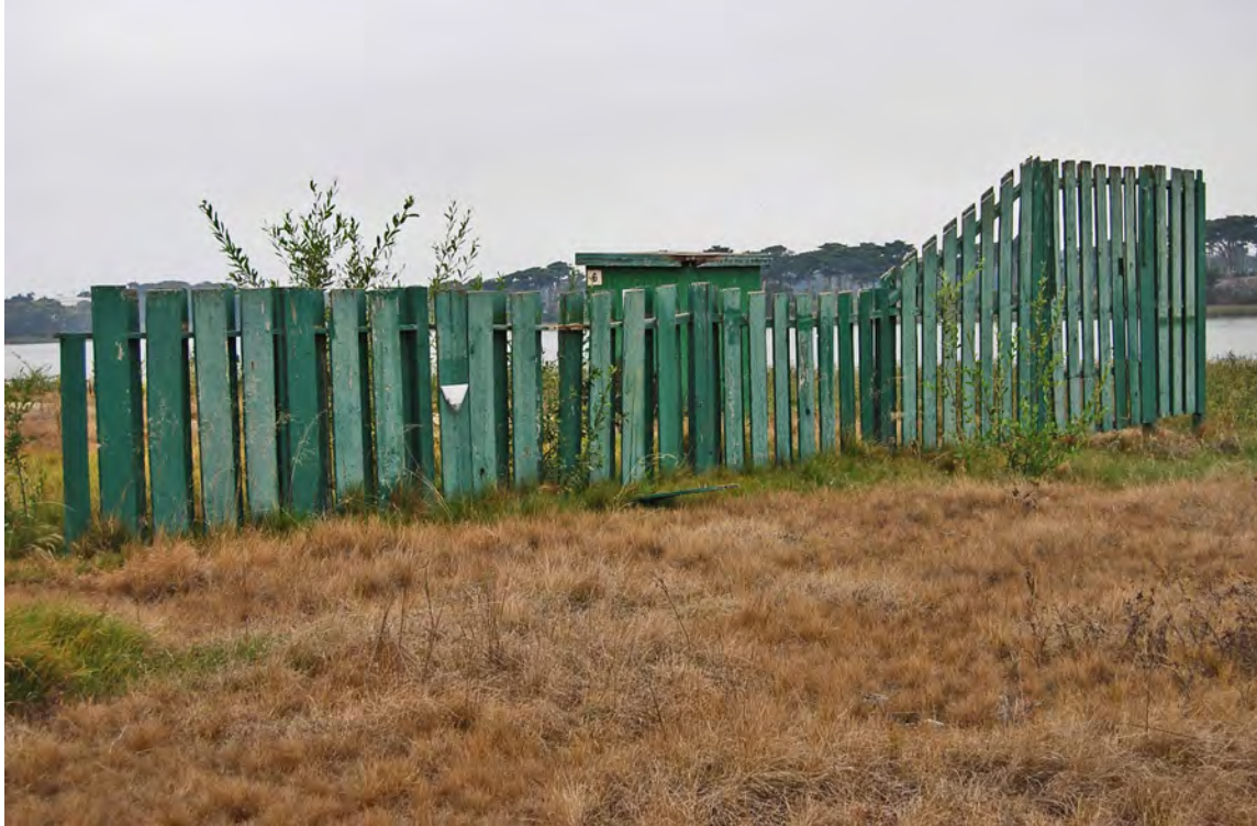
Photo 17. Safety fence (contributing feature) between Skeet Fields 6 and 7; facing northwest; 15 October 2019.
