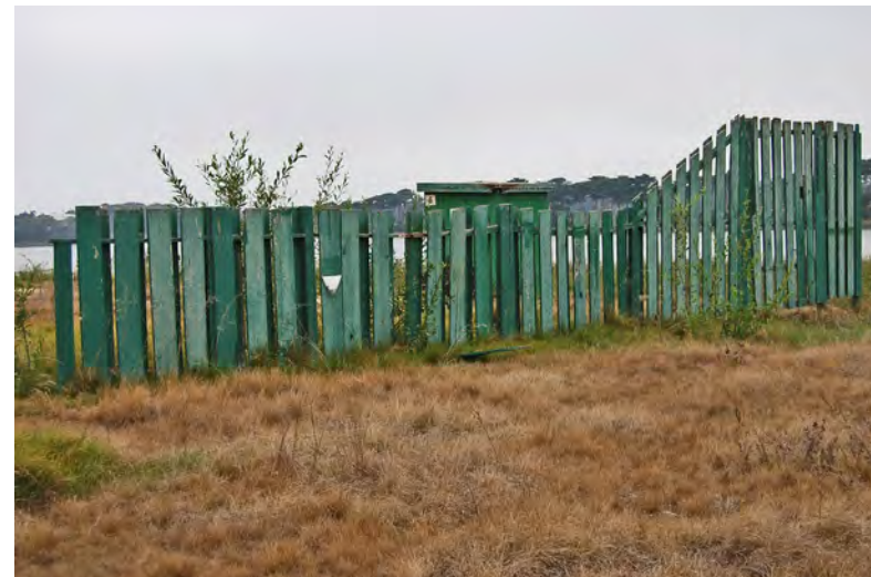
Photo 12. Safety fence between Skeet Fields 6 and 7; facing northwest
