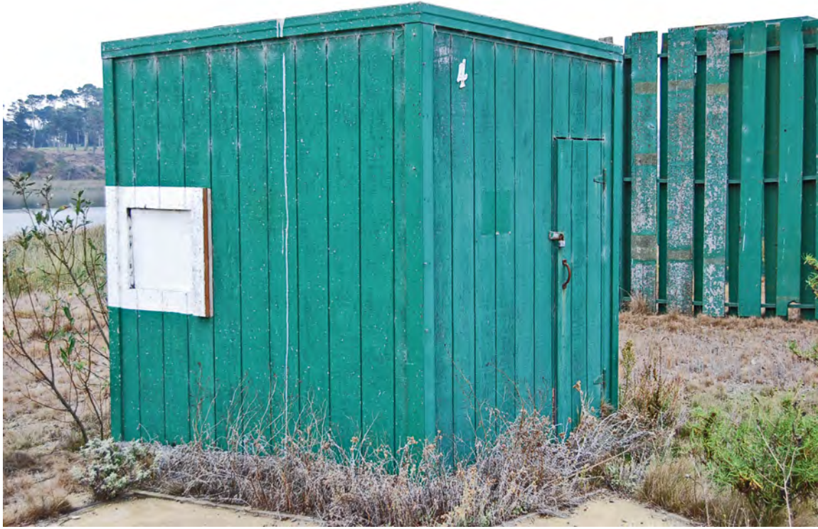
Photo 11. Low House (contributing feature) for Skeet Field 4; facing northeast; 15 October 2019.
