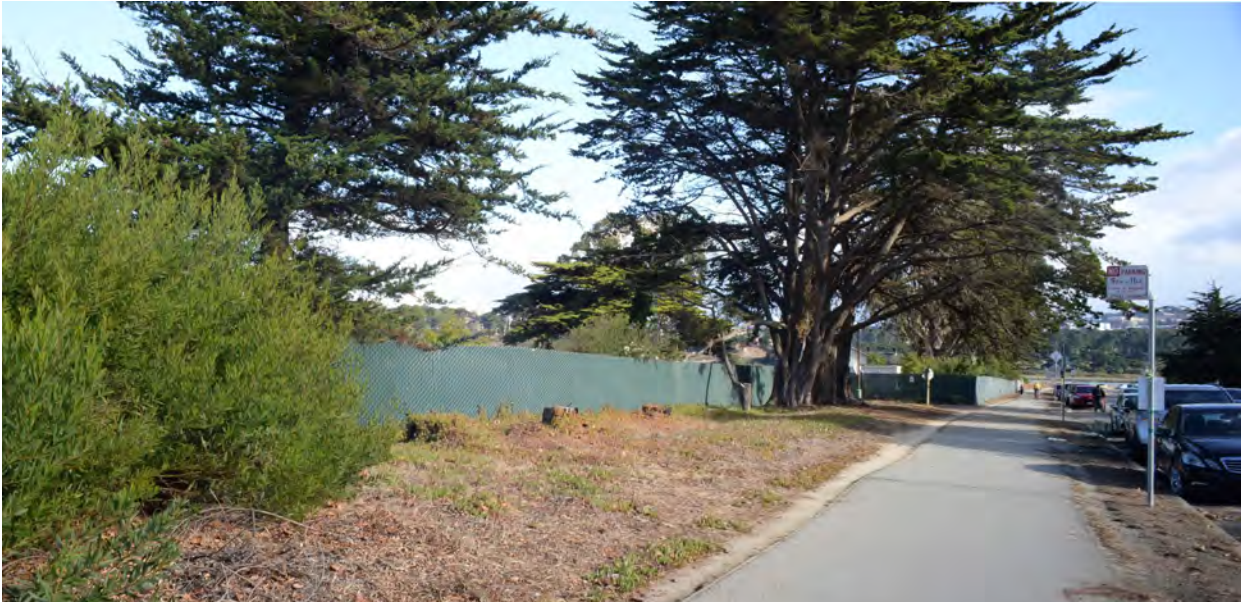
Photo 4 – Existing Fencing Looking Southeast
