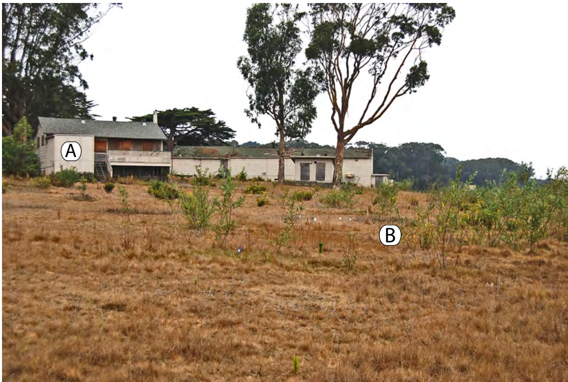
Photo 28. East end of site showing (A) Clubhouse (contributing building) and (B) former location of Skeet Fields 8 and 9 (non-contributing features); facing west; 15 October 2019.
