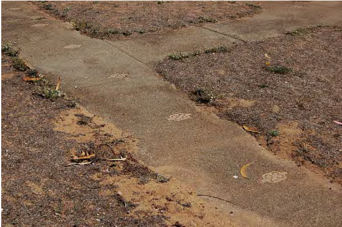
Photo 24. Detail of paved lane layout in trap field with embedded metal tag yardage markers (typical to Fields 1, 2, and 3) (D. Bradley, September 2013).
