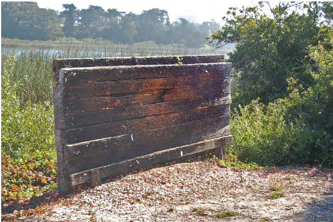
Photo 43. Pattern board located at east end of site; view to NE (D. Bradley, September 2013).
