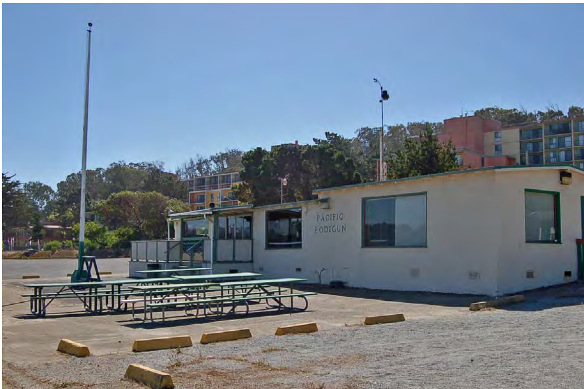
Photo 6. Shell House, Springer memorial flag pole, picnic tables; view to S (D. Bradley, September 2013).
