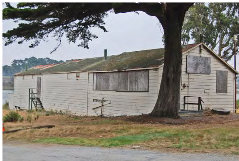
Photo 2. Rifle Range Building; facing northeast; (contributing feature)
