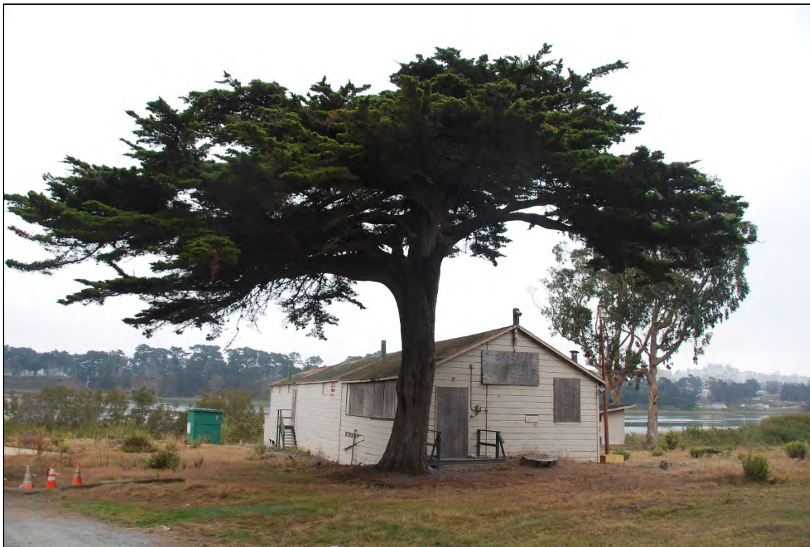
Figure 5: Rifle Range building, a contributing feature (view southeast of west and south elevations)
