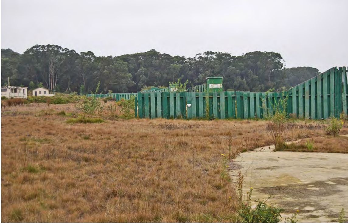
Photo 21. Overview of Skeet Fields 4 to 7 (contributing features) showing linear arrangement (contributing spatial organization characteristic) and level terrace (contributing topographic characteristic); facing west/northwest; 15 October 2019.
