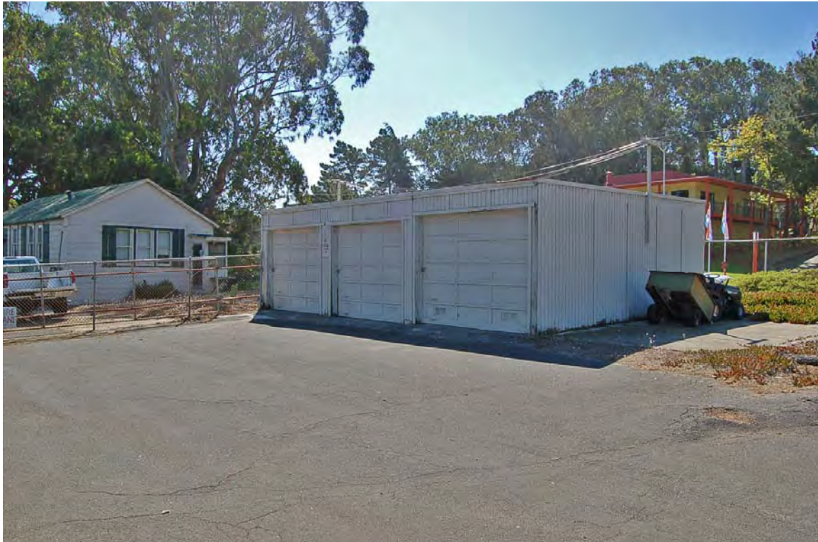
Photo 32. Garage; view to SE (D. Bradley, September 2013).
