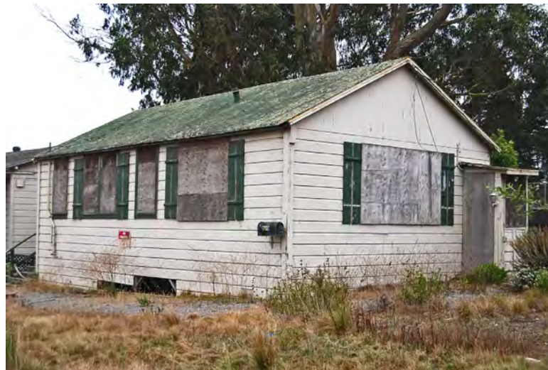
Photo 4. Caretaker's House; facing southeast; (contributing feature)
