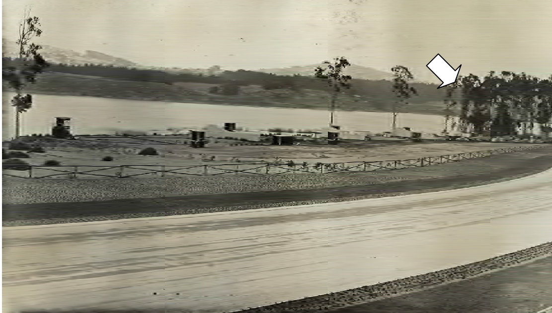
Historic Image 8. Western end of site after the addition of the new skeet fields (Fields 4 to 7) built by club members following flooding and abandonment of original fields in 1937. Photo likely dates from 1938 or 1939 prior to site work done by WPA in 1939 (to prepare the site for the National Skeet Championships held there on 8-12 August 1939) and before the addition of the Rifle Range Building. Also note the presence of a duck tower (see arrow). Source: PR&GC Collection.
