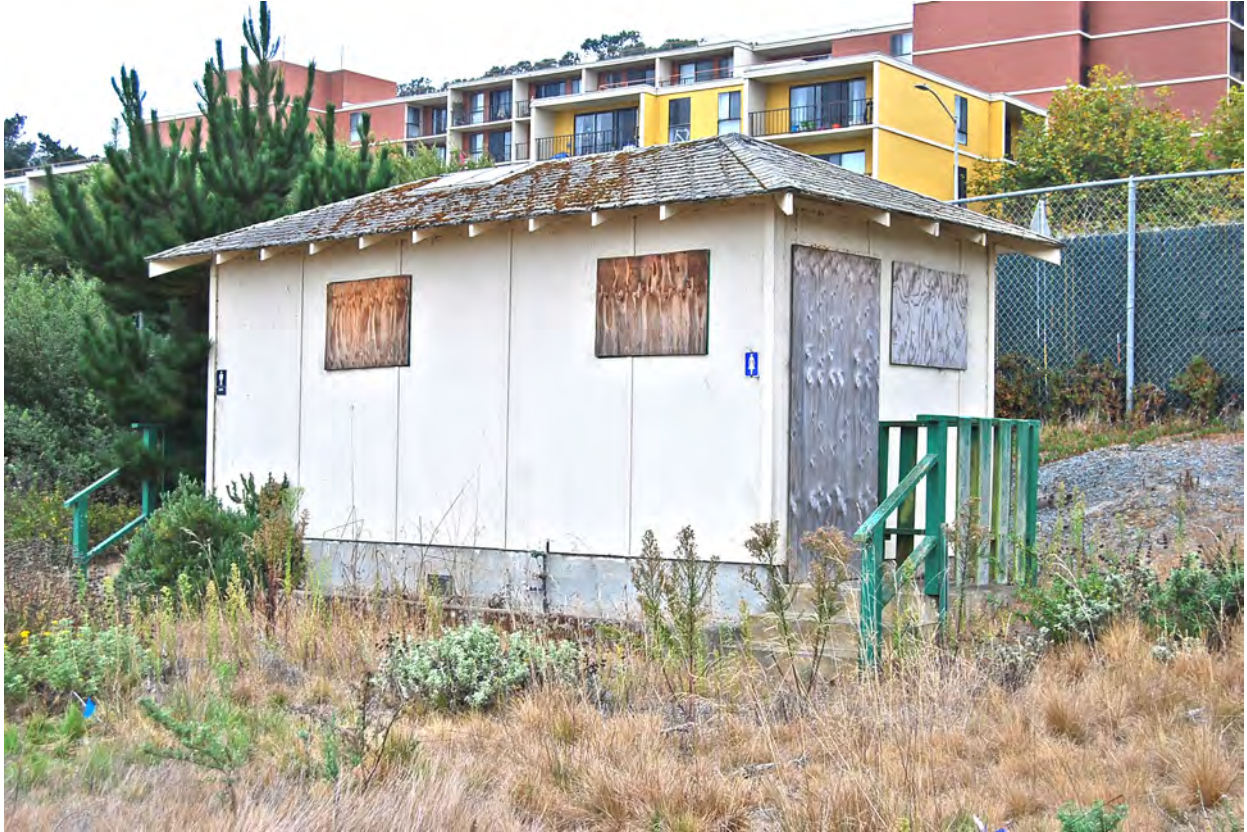
Photo 7. Restroom (non-contributing building); facing southeast; 15 October 2019.
