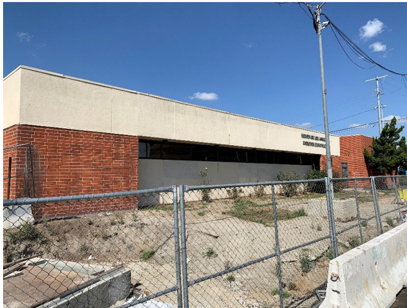
Figure 5-1 East elevation, facing northwest
