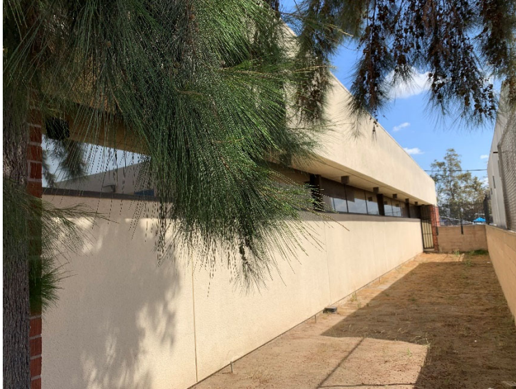
Figure 5-4 South elevation, facing northeast
