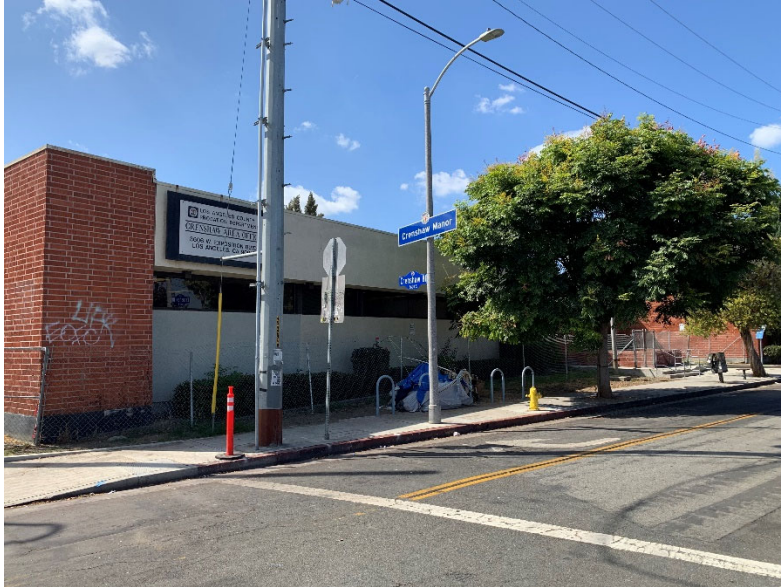
Figure 5-2 North elevation, facing southwest
