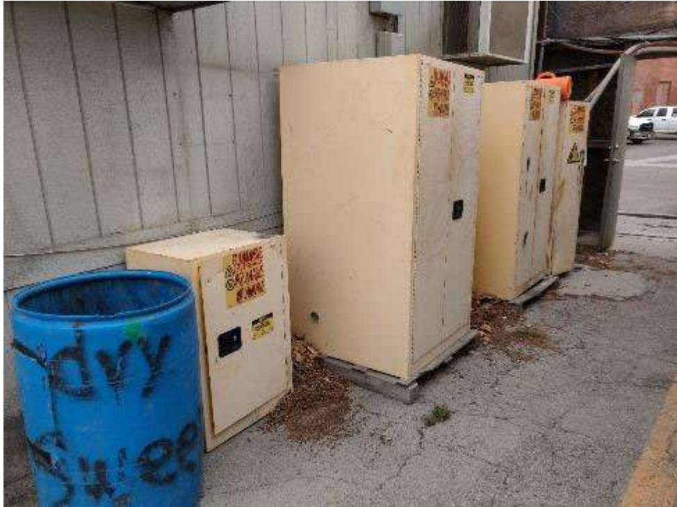
Photo 9: Flammable storage cabinets containing chemicals on the East Block
