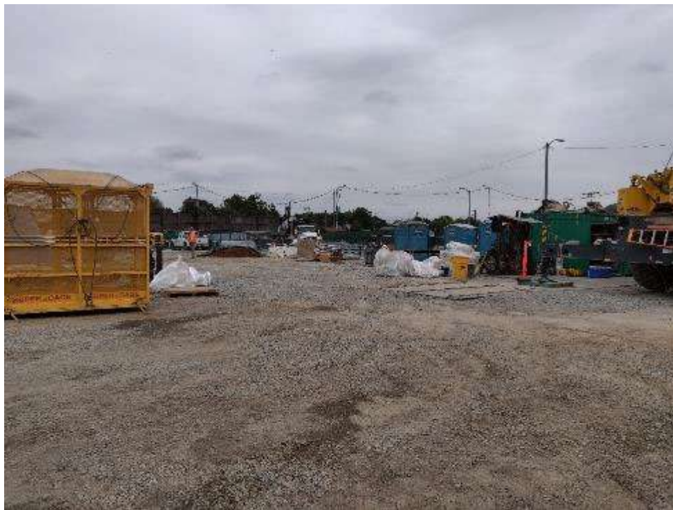
Photo 2: Typical view of constructions activities at the East Block
