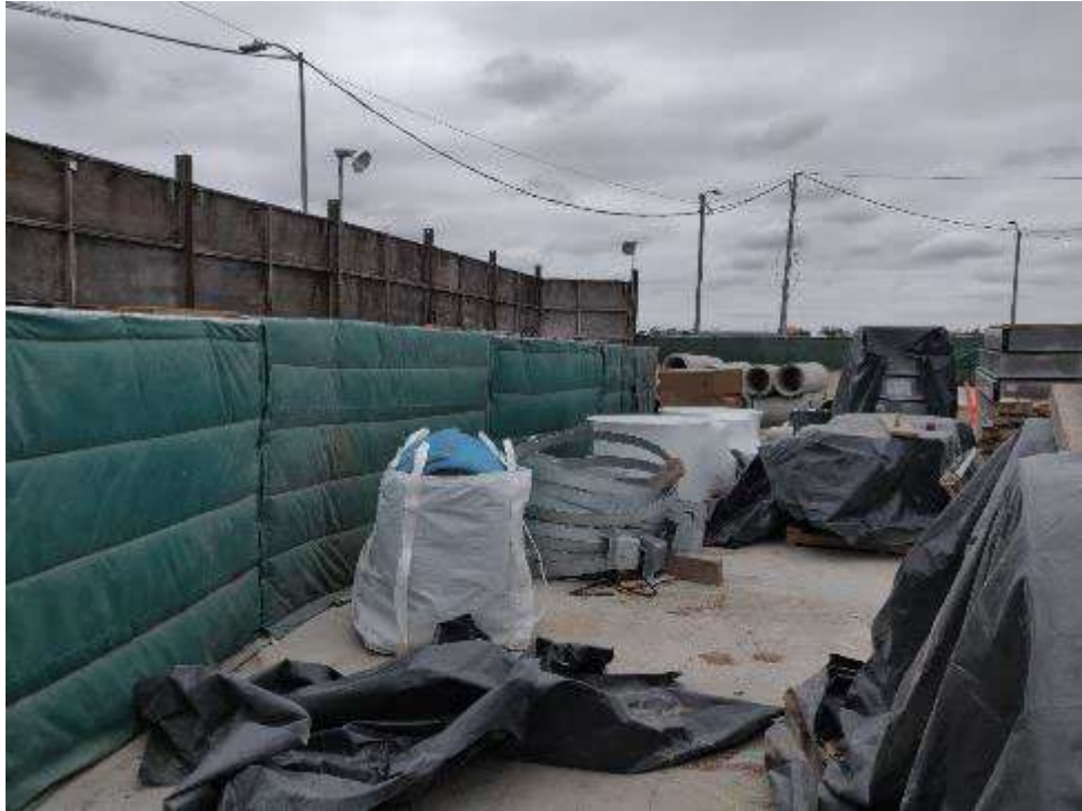
Photo 5: Miscellaneous construction material storage on the East Block
