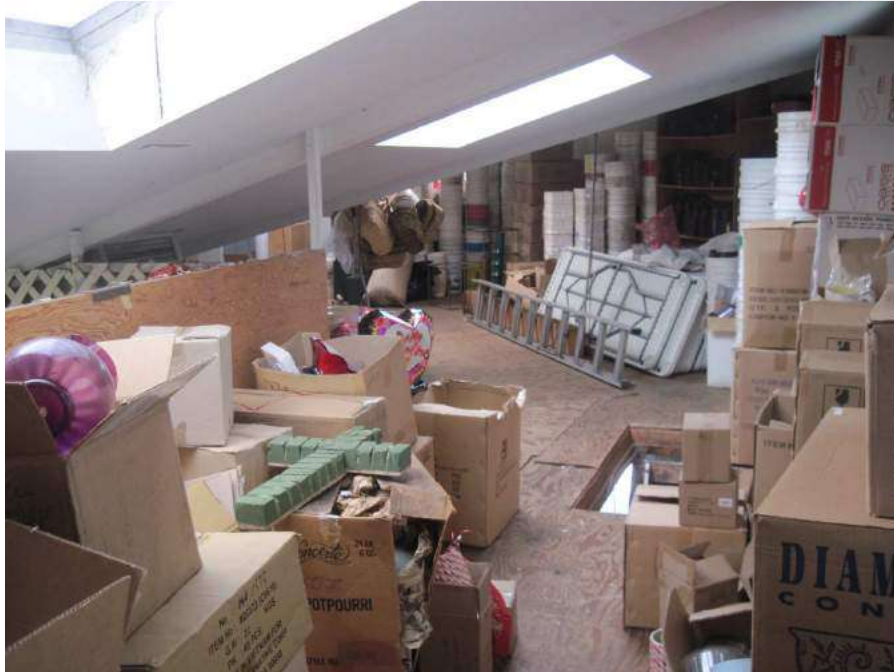
Photograph No. 19: Looking at a mezzanine storage area in the Conroy's Flowers (3646 Crenshaw Boulevard).
