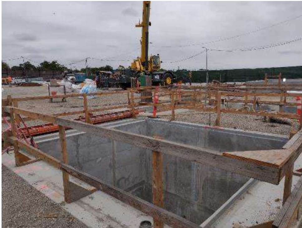
Photo 3: Construction activities associated with the East Block's subway
