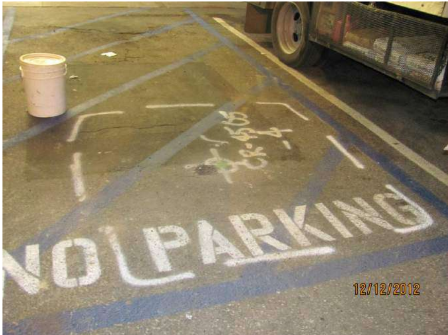
Sampling locations that were abandoned and capped with cold patch asphalt
