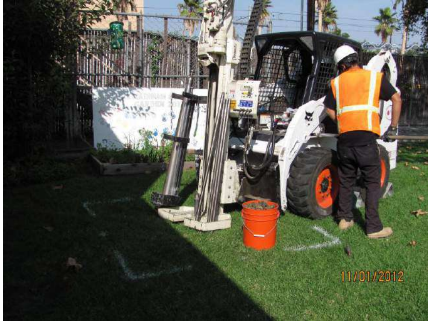
Direct Push drilling – soil sampling
