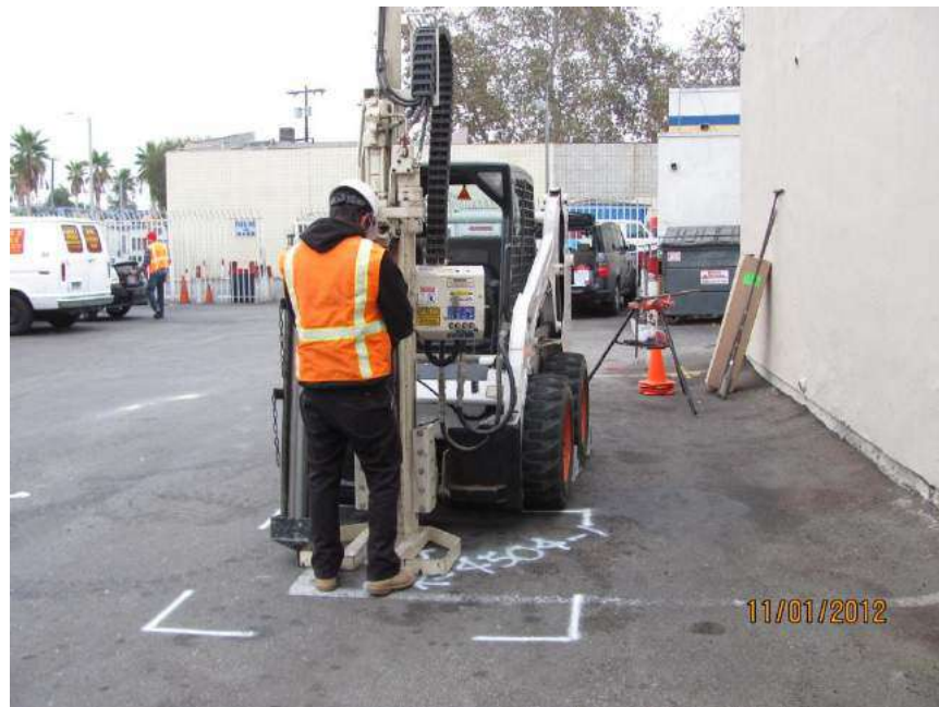
Direct Push drilling – soil sampling
