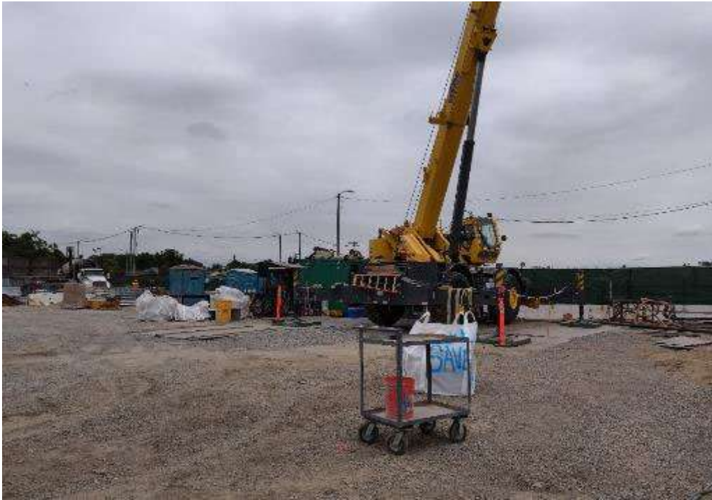
Photo 1: Typical view of constructions activities at the East Block
