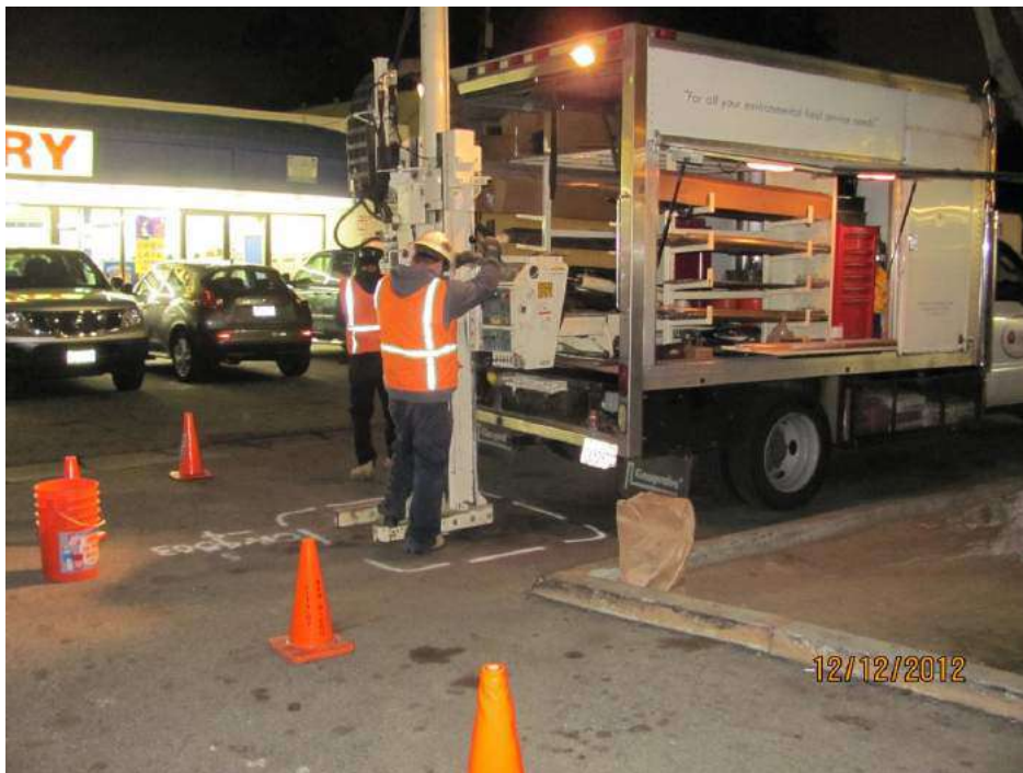
Direct Push drilling – soil sampling
