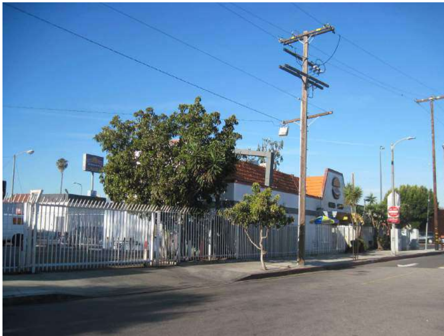
Photograph No. 2: Looking southwest at the on-Site Earlez Grille Chili Factory (3630 Crenshaw Boulevard).
