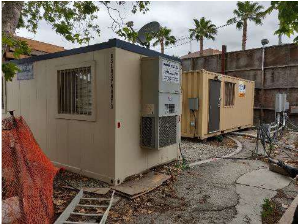
Photo 6: Temporary construction storage and office space on the East Block
