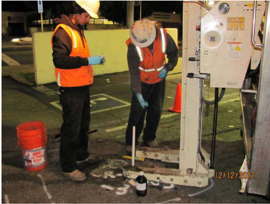
Grab groundwater sampling - Hydropunch™
