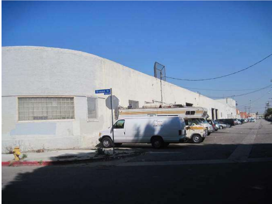
Photograph No. 39: Looking northeast at the adjacent to the east Steeldeck Platform Systems (3335 Exposition Place).
