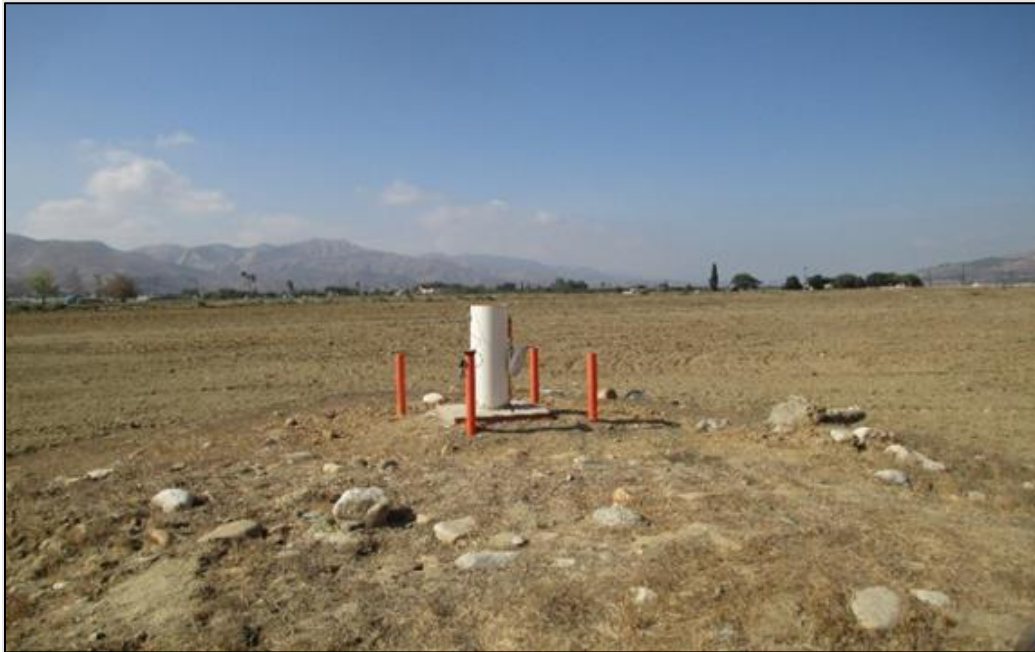
Figure 2: Completed monitoring well and surface casing with bollards.
