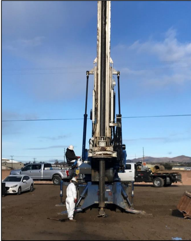
Figure 4: Example auger drill rig.
