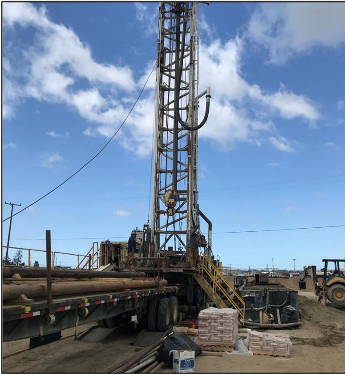
Figure 6. Reverse-rotary drill rig.
