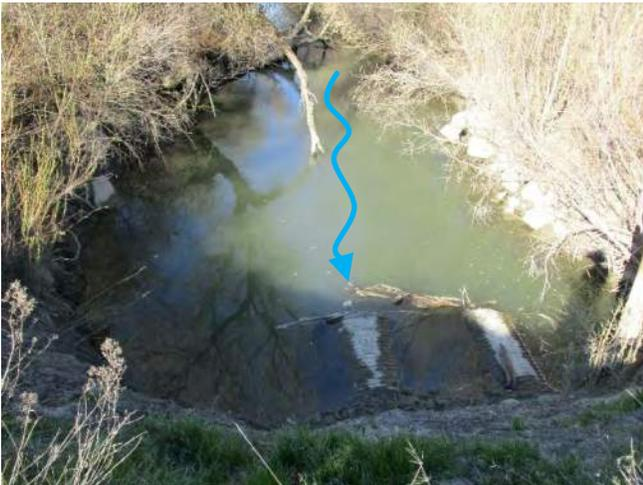
Photo 3. View looking west, toward the two main culvert inlets in the Outfall Channel on the west side of the Yolo Bypass levee. Rip-rap lines the channel. 27 February 2020.
