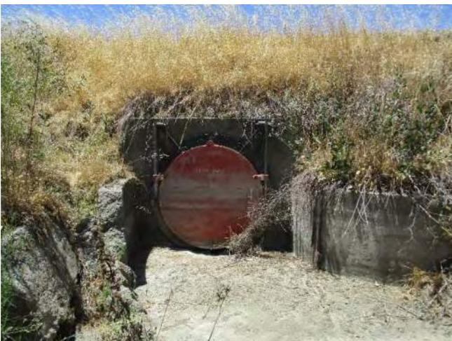
Photo 17. The flapgate on the northernmost culvert outlet on the Outfall Channel. This arm of the channel was dry during fieldwork in February and June. 17 June 2020.
