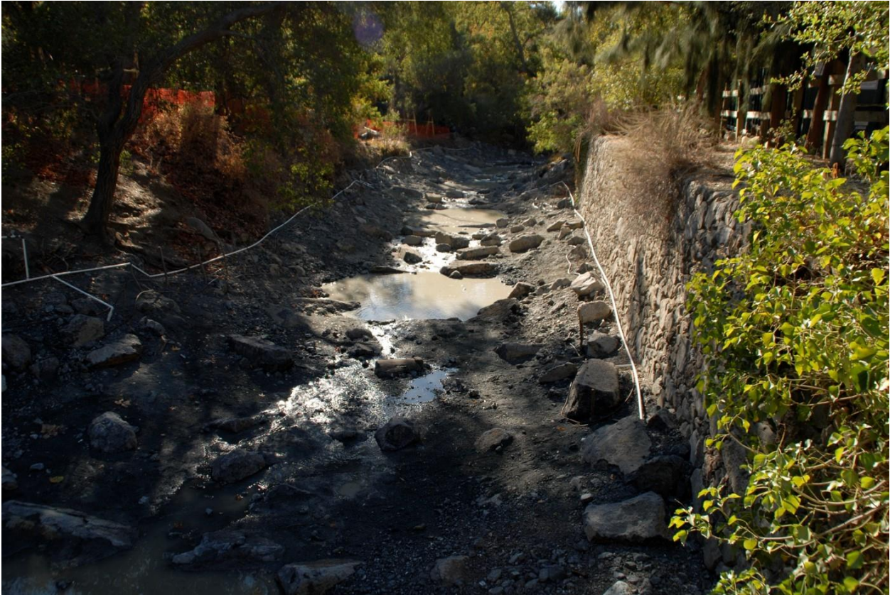
Figure 9-1. A chute and pool roughened channel in Alum Rock Park, San Jose, CA following completion of construction.
