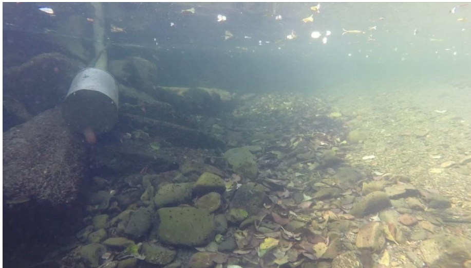
Figure 8-4 Diversion Intake (submerged looking upstream).
