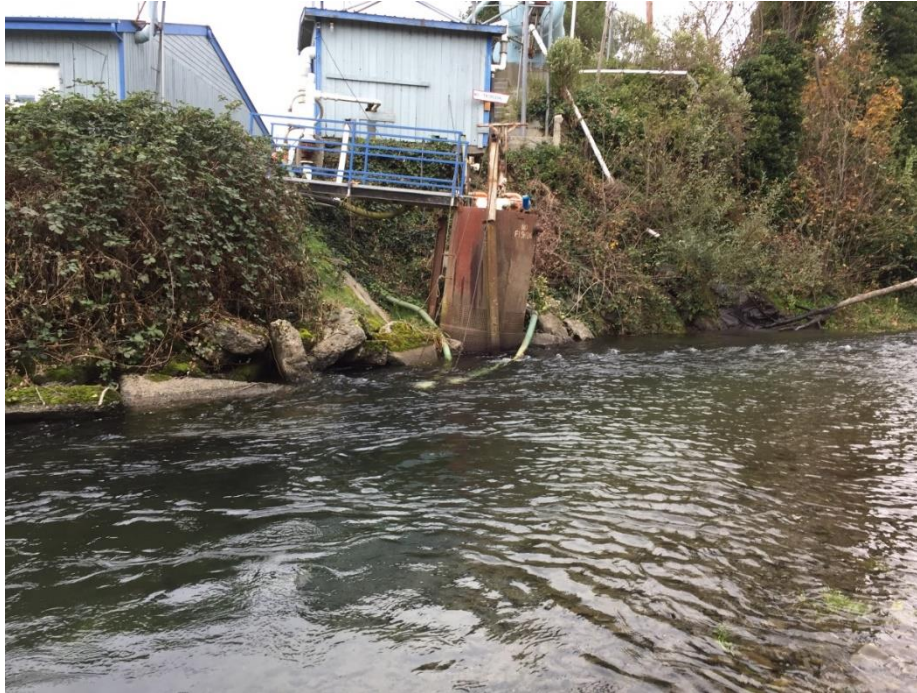
Figure 8-3 Hatchery Diversion Infrastructure (looking towards right bank).
