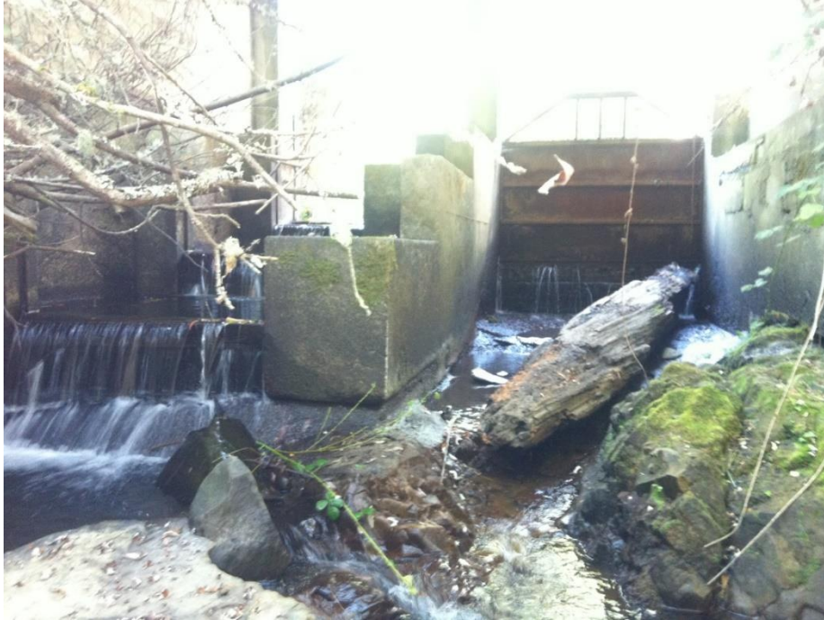
Figure 8-8 Dominie Creek Diversion Structure (looking upstream).
