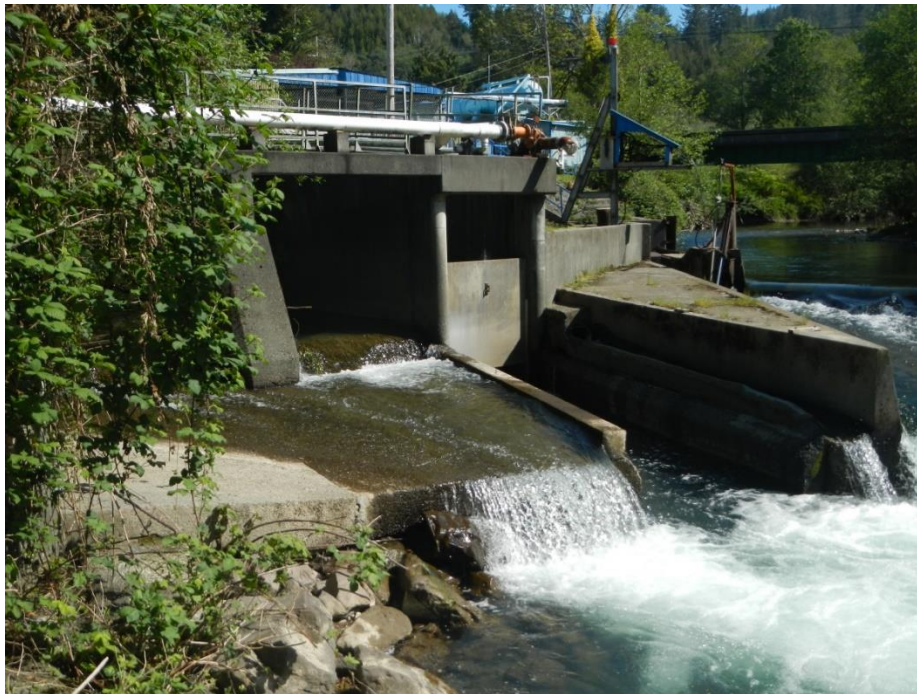
Figure 8-6 Dominie Creek Concrete Apron (looking upstream).
