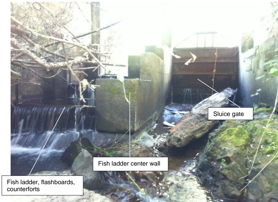
Image 1-6. Dominion Creek diversion structure (facing upstream)
