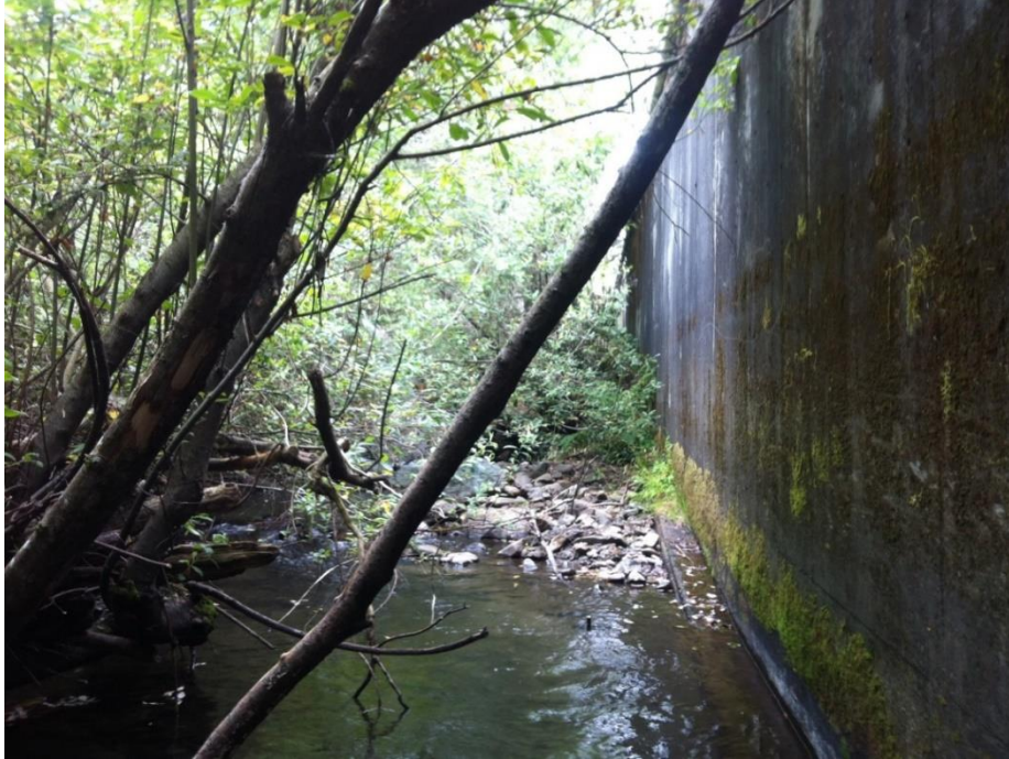
Figure 8-7 Outer Fish Ladder Wall on Dominie Creek (looking upstream).
