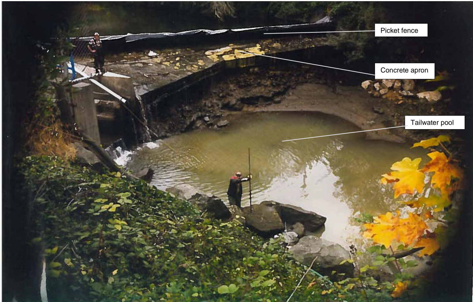
Image 1-1. Rowdy Creek Diversion Weir at confluence with Dominie Creek (looking upstream)
