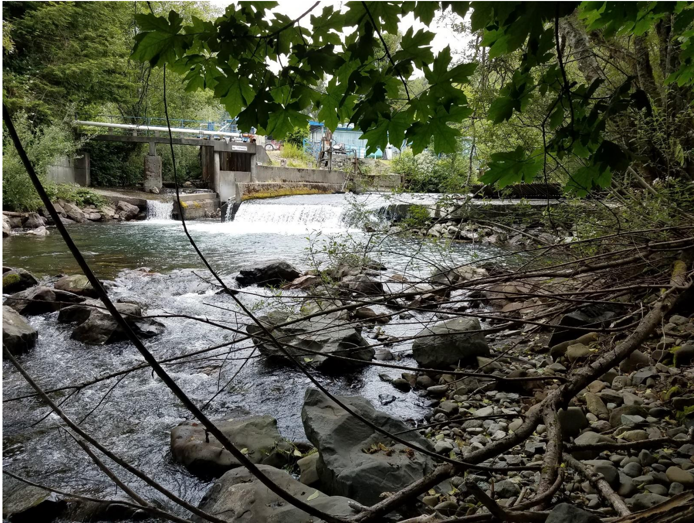
Eastern bank conditions downstream of concrete weir on Rowdy Creek, and confluence with Dominie Creek which enters Rowdy Creek on left. Note the numerous drops from concrete infrastructure present at mouth of Dominie Creek, and downstream of concrete weir.
