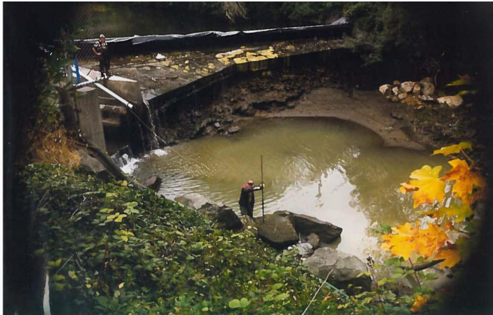
Figure 8-1 Rowdy Creek Diversion Weir (looking south towards river left bank).
