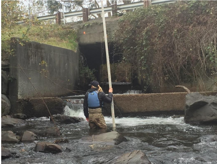
Figure 8-10 Dominie Creek Highway 101 Culvert Crossing (looking upstream).
