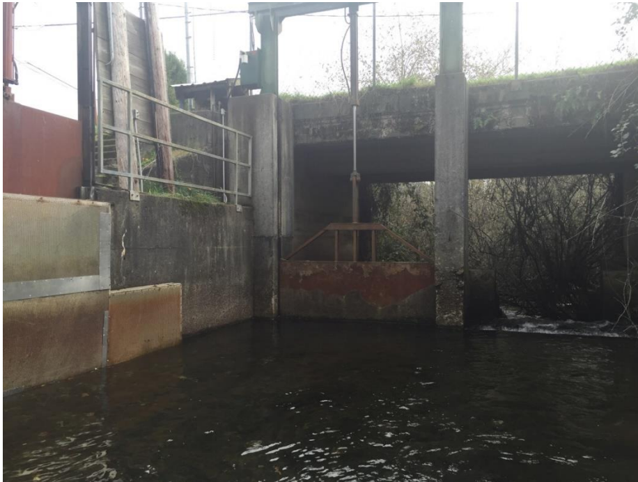
Figure 8-9 Dominie Creek Diversion Structure (looking downstream).
