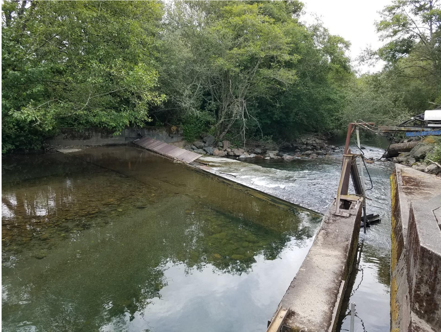
Concrete weir infrastructure on Rowdy Creek, facing downstream.
