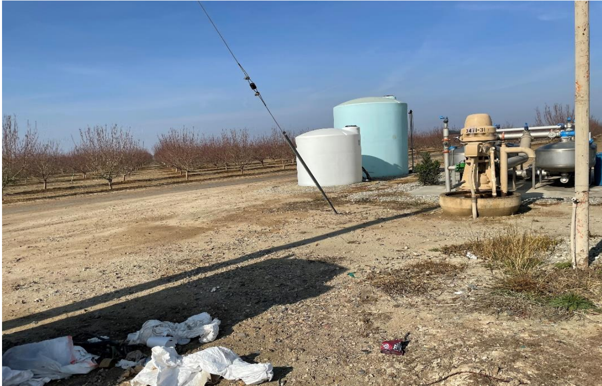
Photo 3. Well 88-25-031 (facing northwest).
