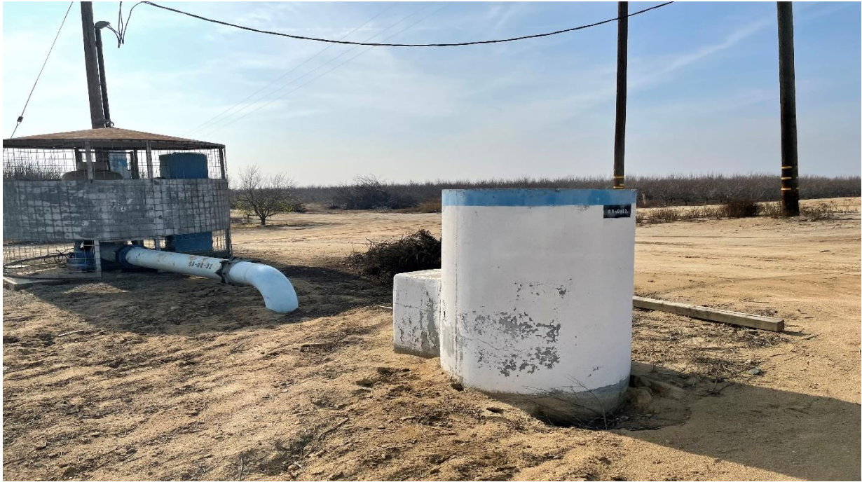
Photo 10. Well 99-00-032 adjacent to orchard facing north.
