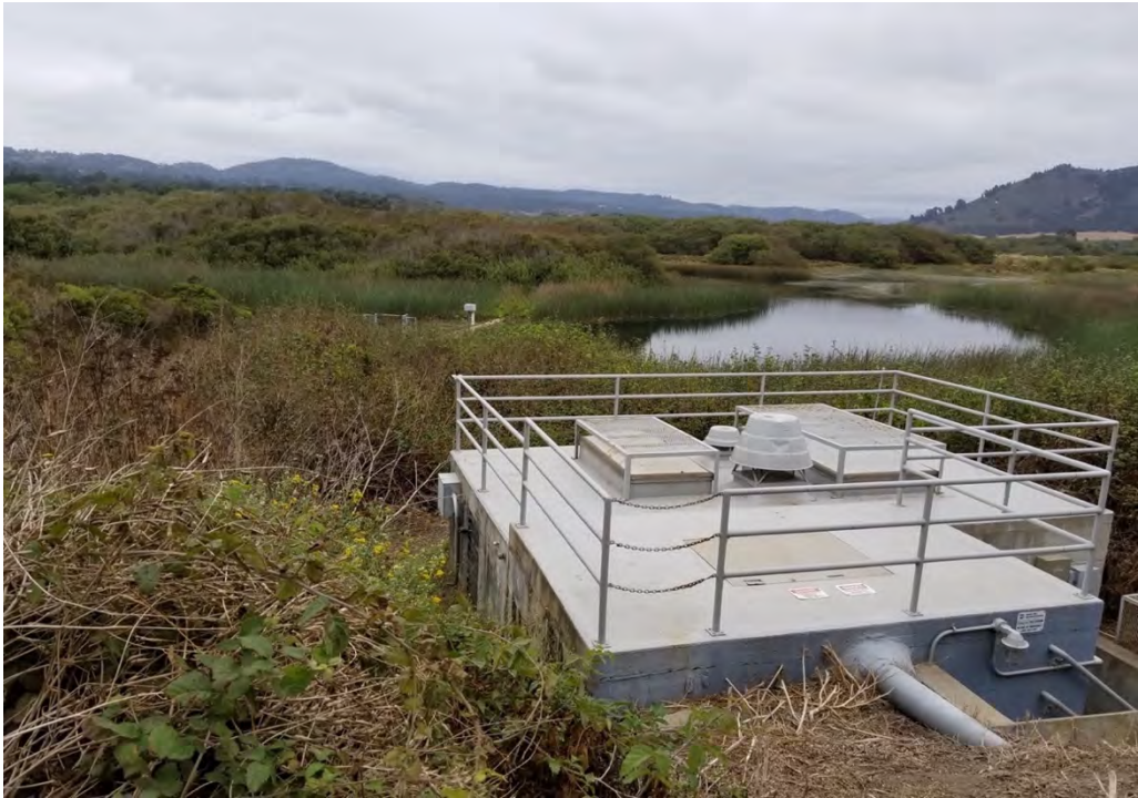
Figure 8. View of Project Area from Calle la Cruz Pump station
